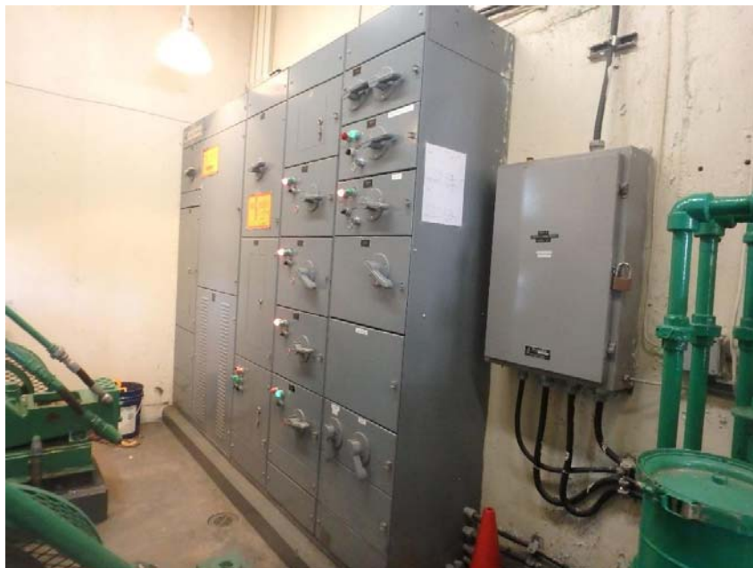
Photo 17 and 18 - Pump Room with MCC and upper gate oil accumulator
