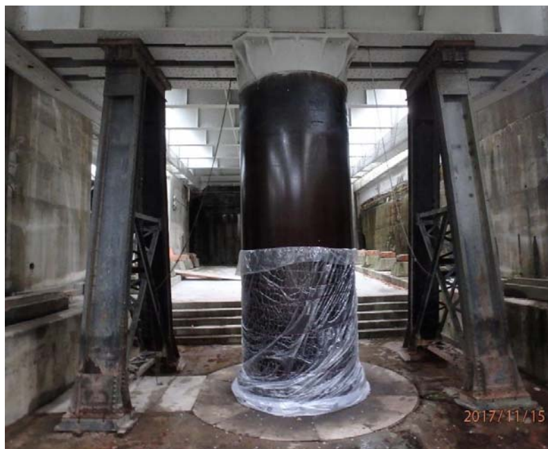
Photo 9 – Ram and Support Frames in navigation season
