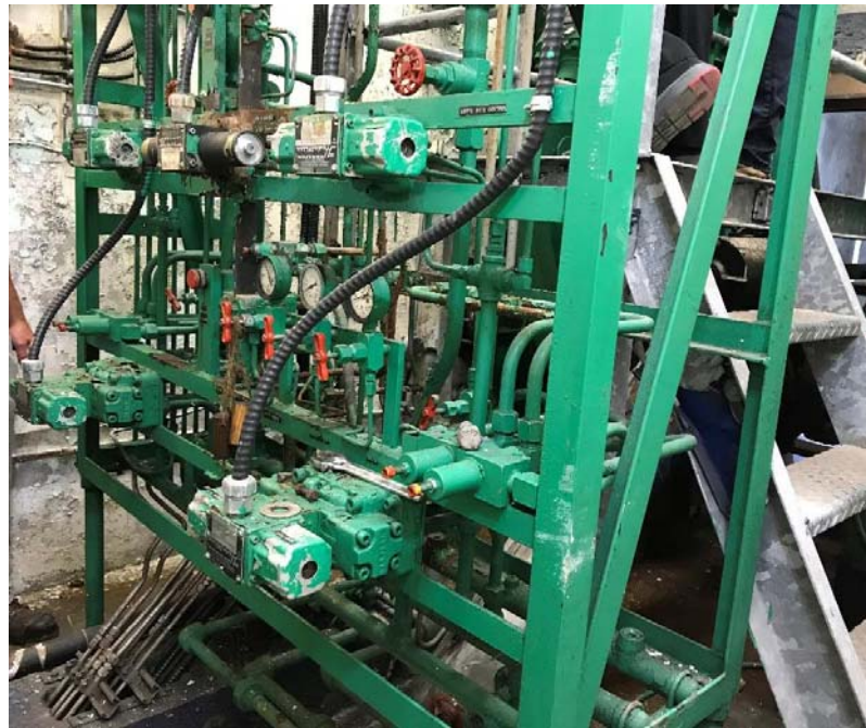
Photo 21 – Upper gate hydraulic controls
