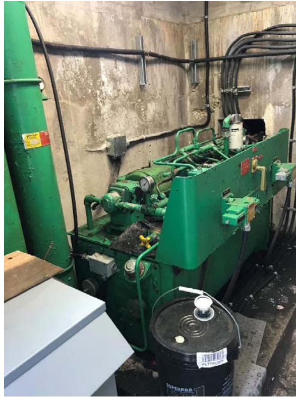
Photo 26 - Guard gate Hydraulic Power Unit (HPU)
