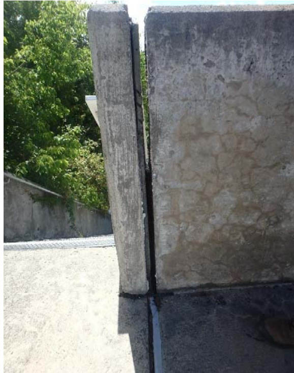
Photo 11 - Increasing joint gap between stairways and the main concrete structure, located upstream of Upper Reach Abutment
