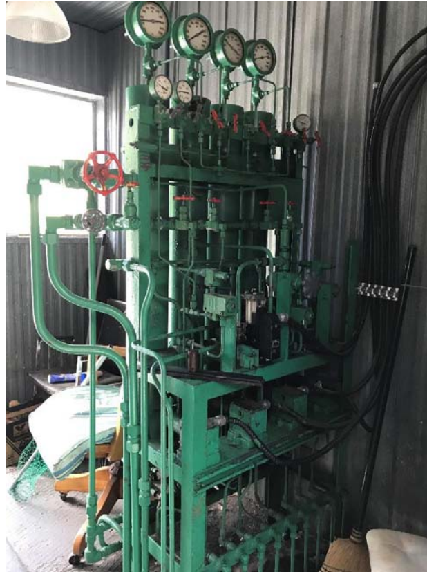
Photo 24 – Lower gates oil accumulator
