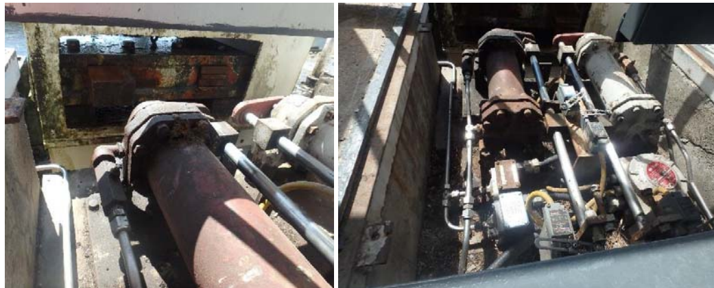
Photo 12, 13 and 14 - Gate latching pins and latching cylinders
