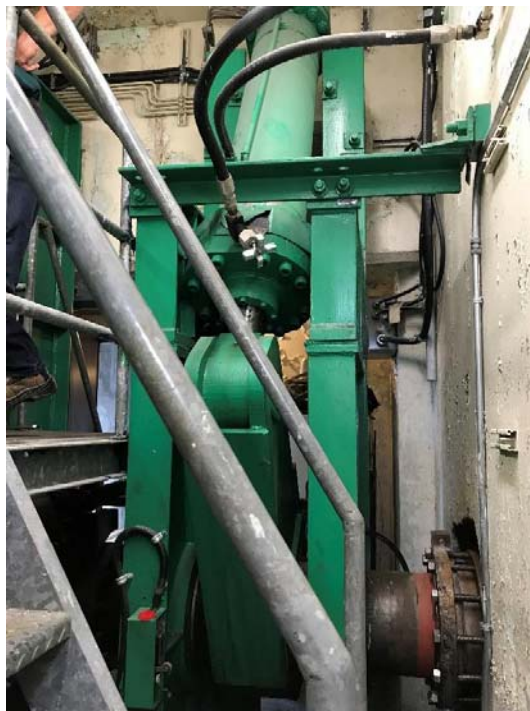
Photo 20 – Upper gate operating cylinder
