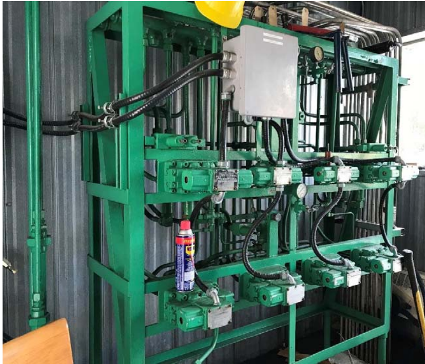
Photo 23 – Lower gates hydraulic controls
