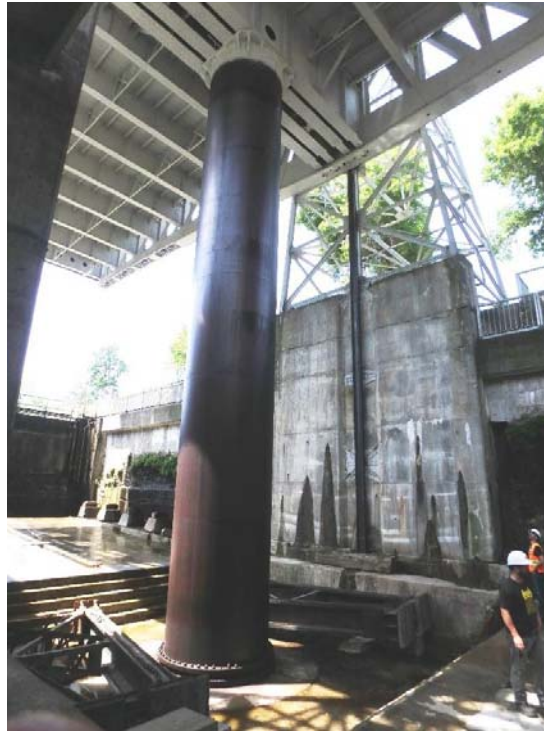
Photo 9 – Ram and Support Frames in navigation season
