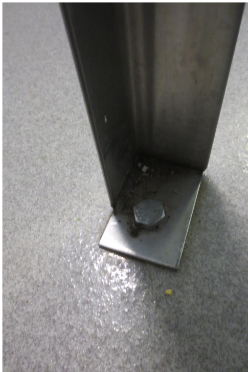
Above: Existing Bed (left) and Shelf (right)Fastener in Assiniboine Unit. New fasteners for new furniture to match
