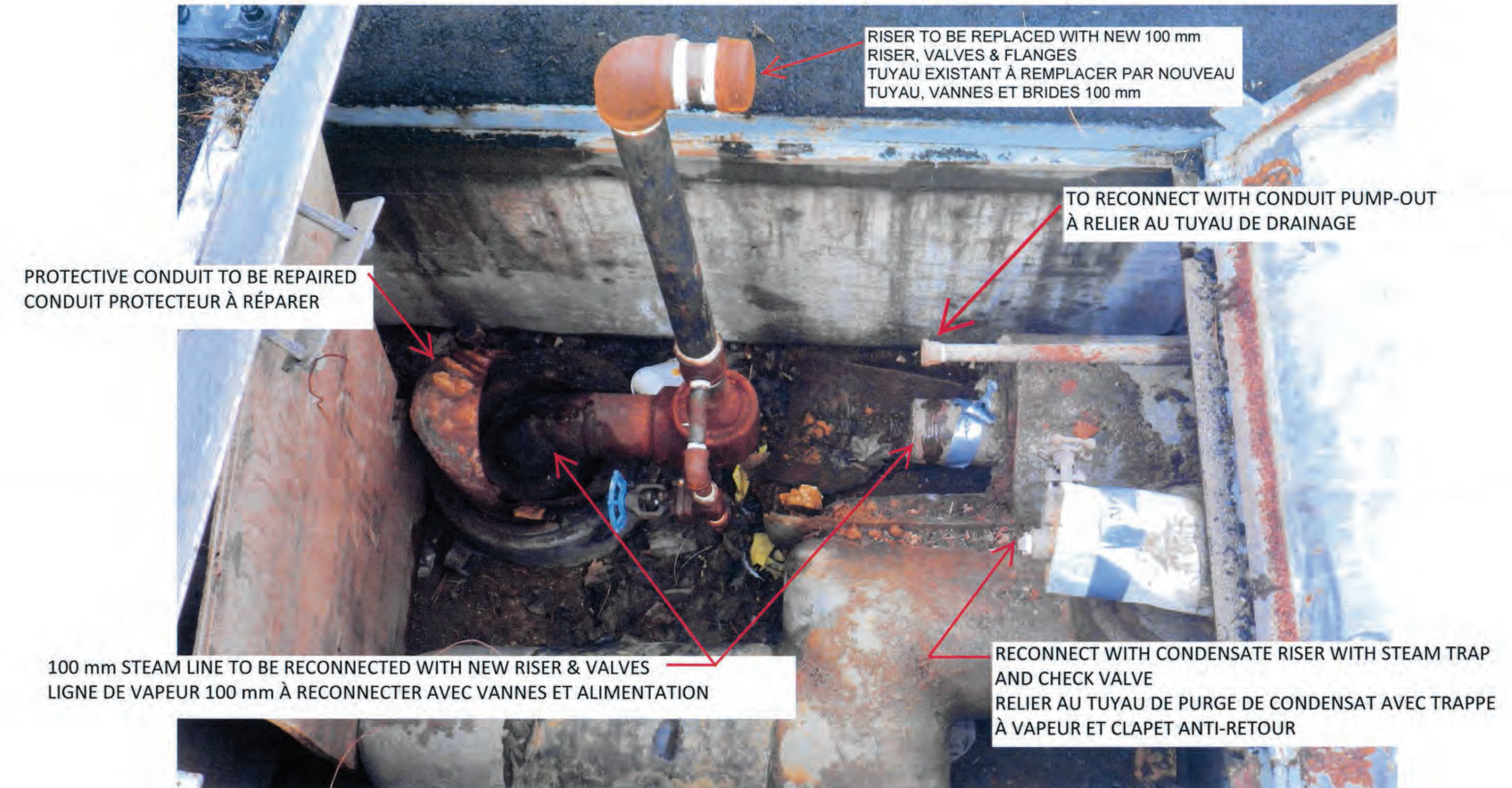
WEST ABUTMENT STEAM & CONDENSATE - ANNOTATED PHOTO CULÉE OUEST - PHOTO TUYAUTERIE VAPEUR & CONDENSAT
