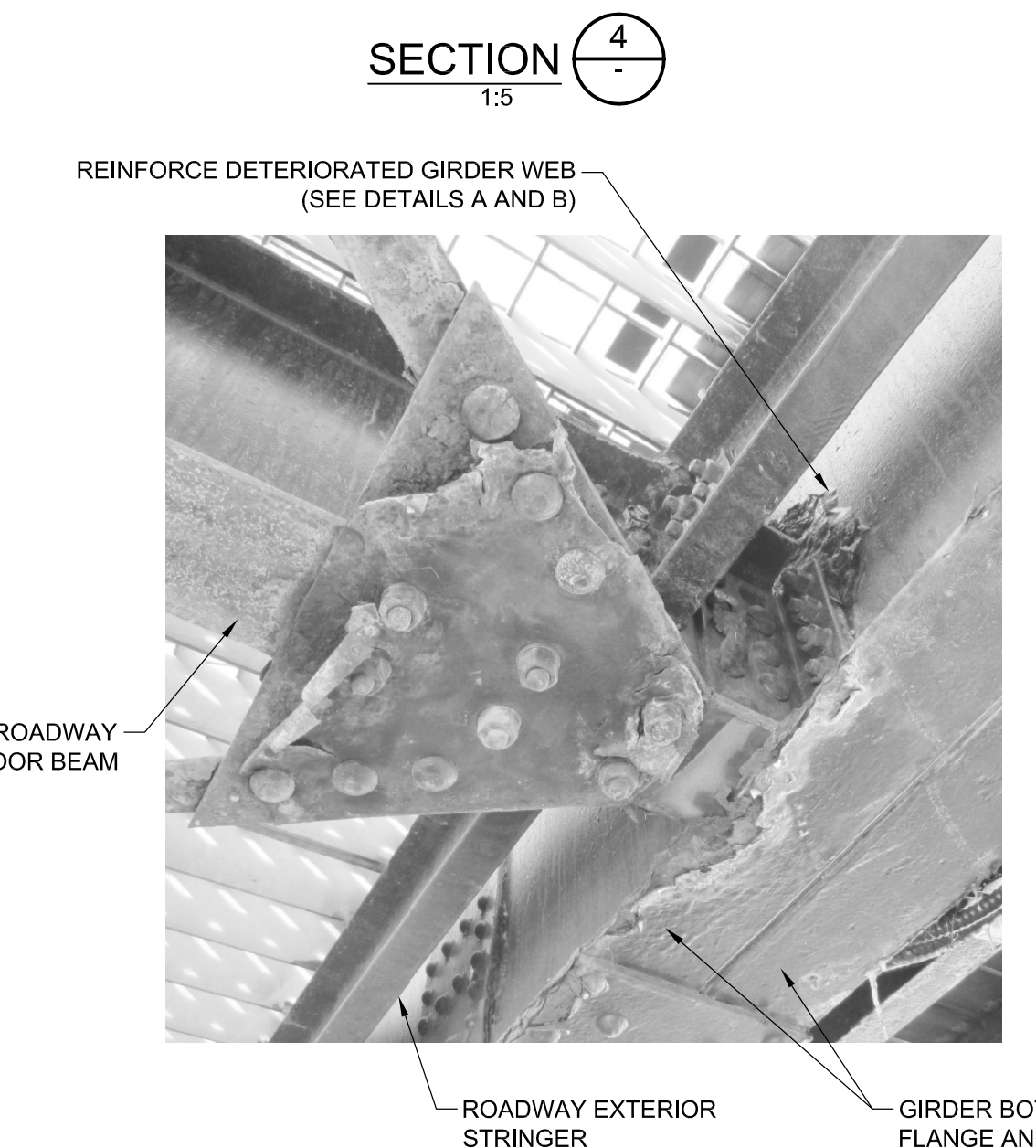
EXAMPLE OF GIRDER WEB DETERIORATION AT FLOOR BEAM CONNECTION (FB5 AT EAST GIRDER SHOWN)
