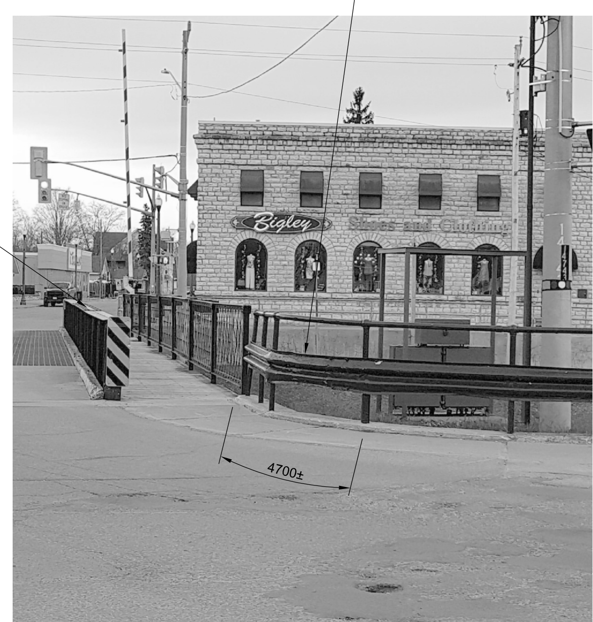
GUIDE RAIL REPLACEMENT (NORTH ABUTMENT)
