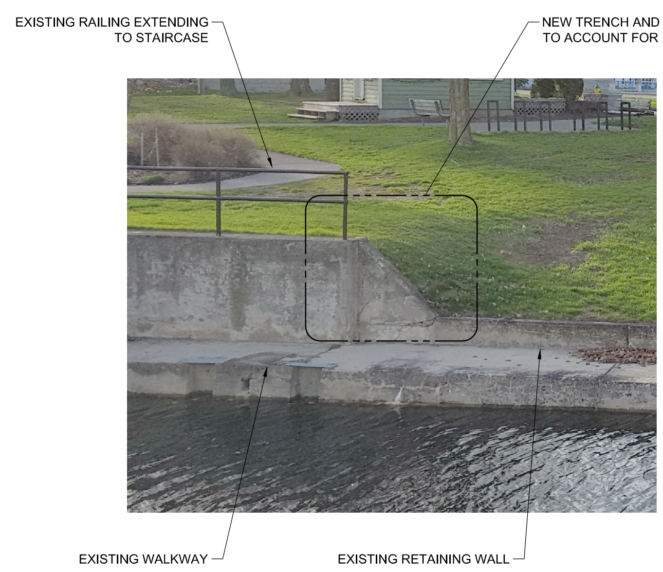
PHOTO 1 (LOOKING NORTH WEST)
