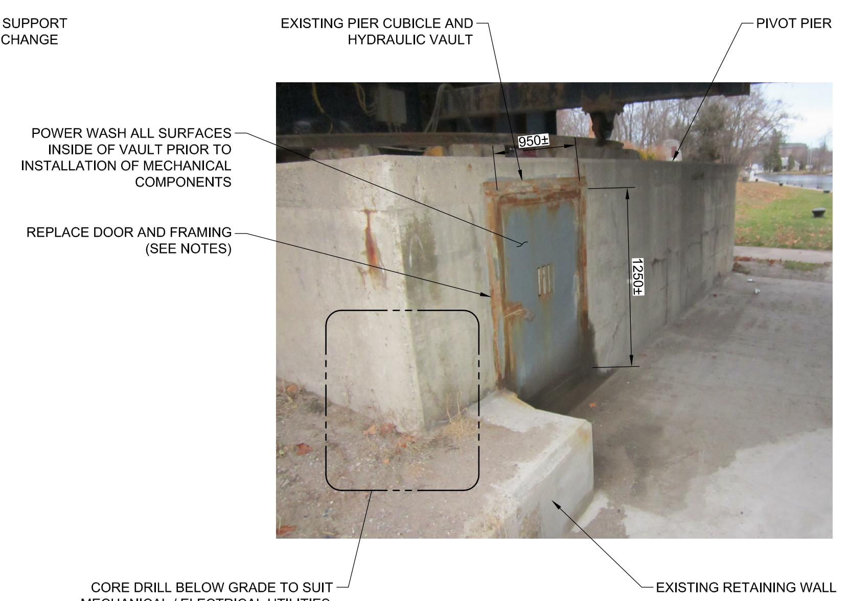
PHOTO 2 (LOOKING NORTH EAST)
