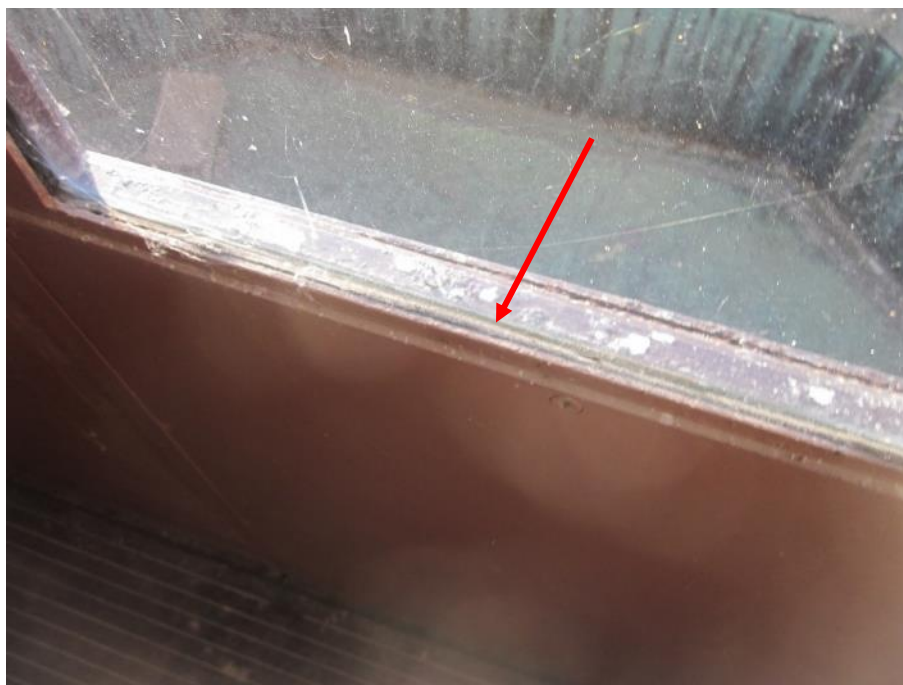
Photo 2: Typical example of asbestos-containing window putty installed between metal frame components and the glass (Window D-D, South Elevation pictured)
