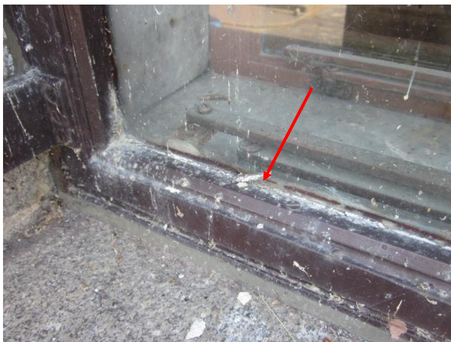
Photo 1: Typical example of asbestos-containing window putty, installed between the metal frame components and the glass (F Window, South Elevation pictured).
