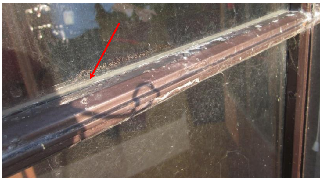
Photo 4: Typical brown painted window components contain 707 to 921 ppm lead
