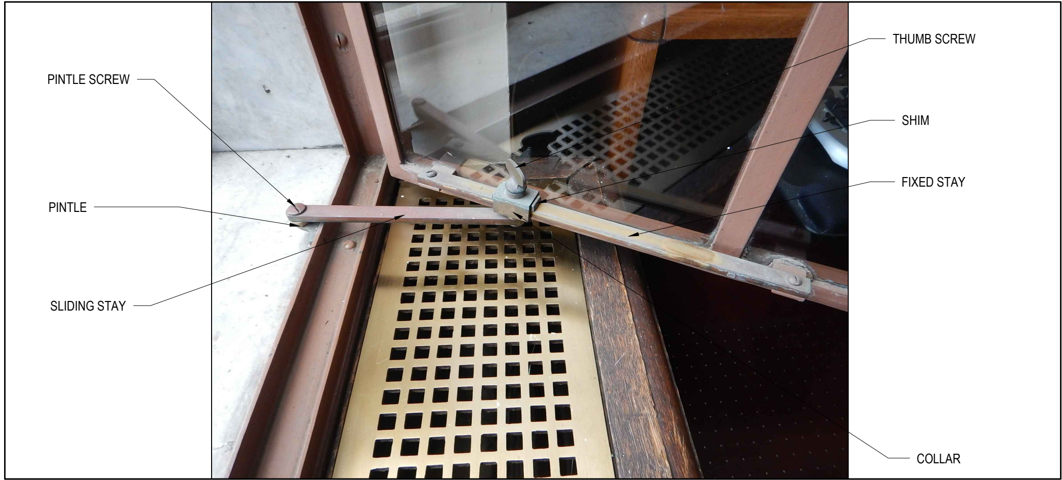
6 TYPICAL CASEMENT STAY COMPONENTS N.T.S.
