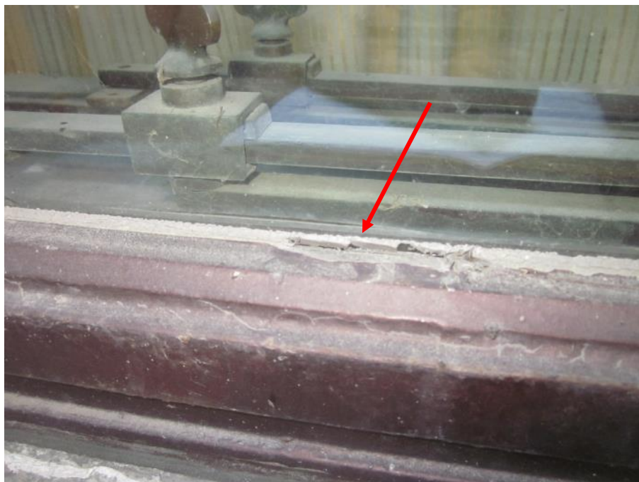
Photo 3: Typical example of asbestos-containing window putty installed between metal frame components and the glass (Window O, West Courtyard pictured).
