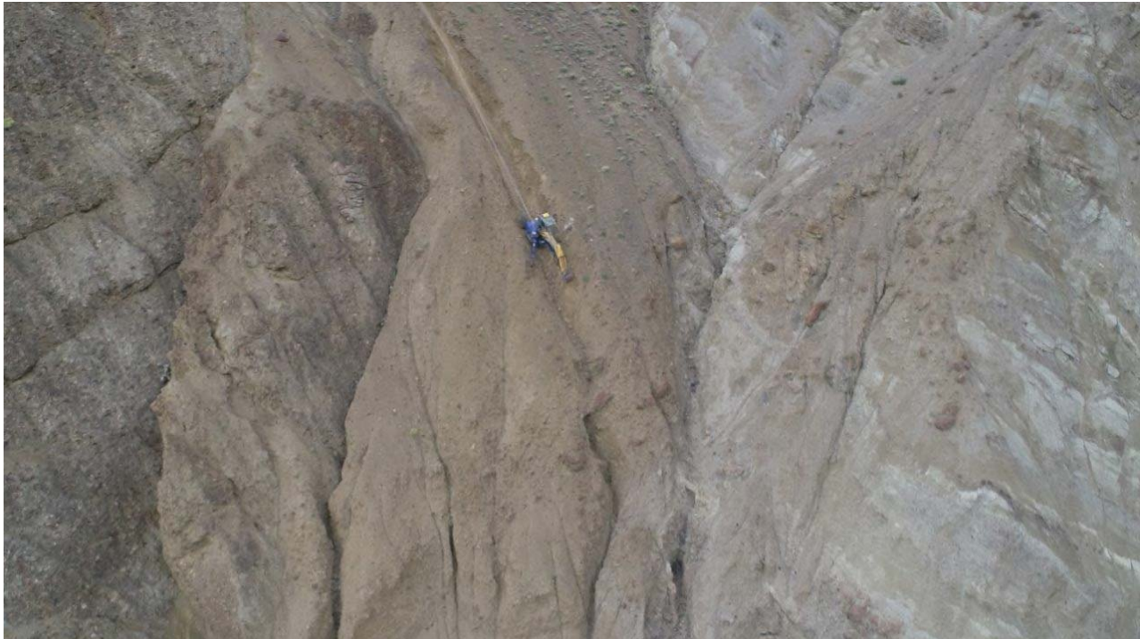
Figure 2 - Spider excavator descending the steep slopes using a remote operated winch assist
