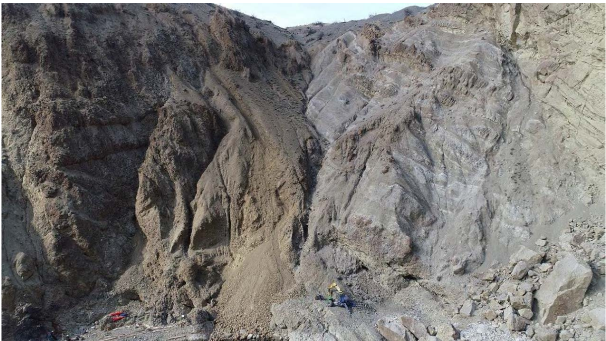
Figure 1 - Spider excavator working to establish access along the base of the slide
