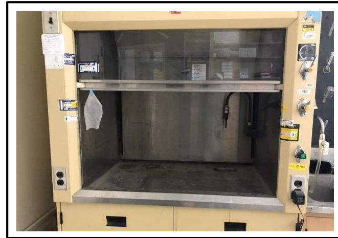
Photograph 2: Asbestos containing transite panels in fume hood rooms EW6 – Building 50
