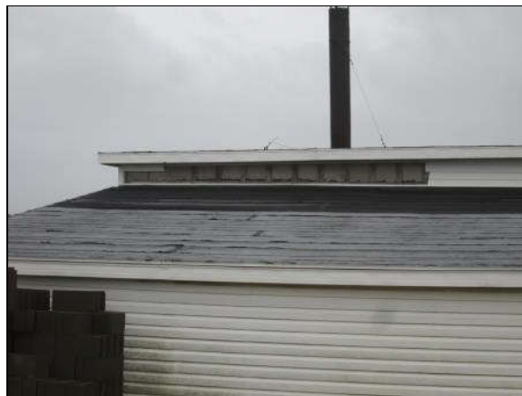
Photograph 2 – Asbestos-containing roofing materials.
