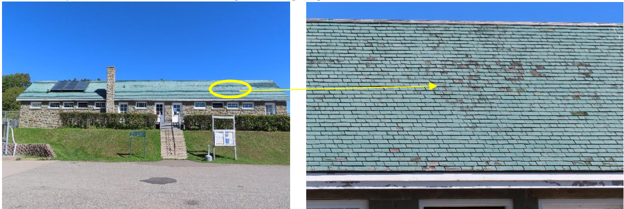
Figure 3: Bathhouse Roof Requiring Replacement
