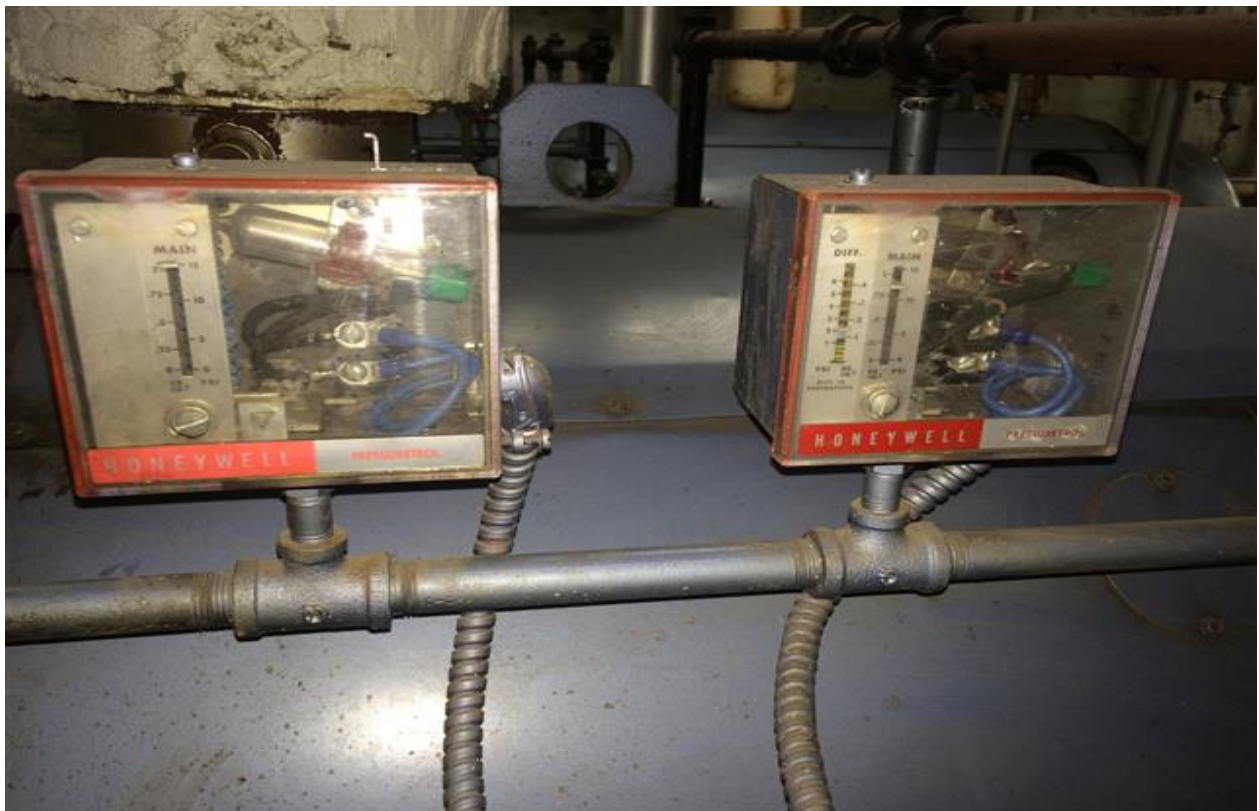
PHOTO 6: Two of four mercury thermostats that were observed to be connected to the two boiler units in the Basement of the subject building.
