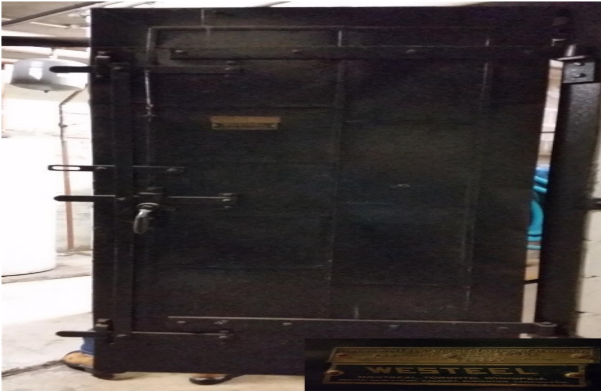
PHOTO 7: View of fire rated door found in the Basement of the subject building. Fire rated doors are known to have been manufactured with asbestos, they should be presumed to be asbestos-containing unless proven otherwise by laboratory analysis.
