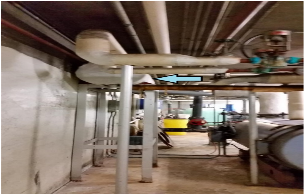
PHOTO 5: View of sample location of thermal insulating parging cement over diamond mesh, over fibre glass on the heat exchange cylinder, (grey and off-white colour) located in the Basement of the subject building. A bulk sample (BS-FBH-12A) of this material was found to contain 40 % Chrysotile .
