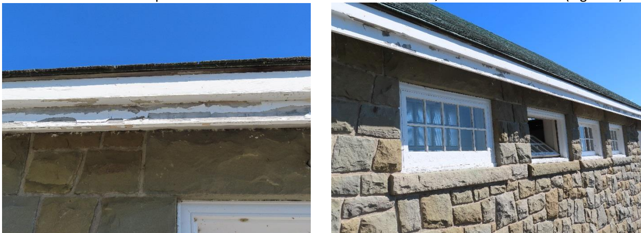
Figure 4: Exterior Wood Trim and Windows Requiring Replacement
