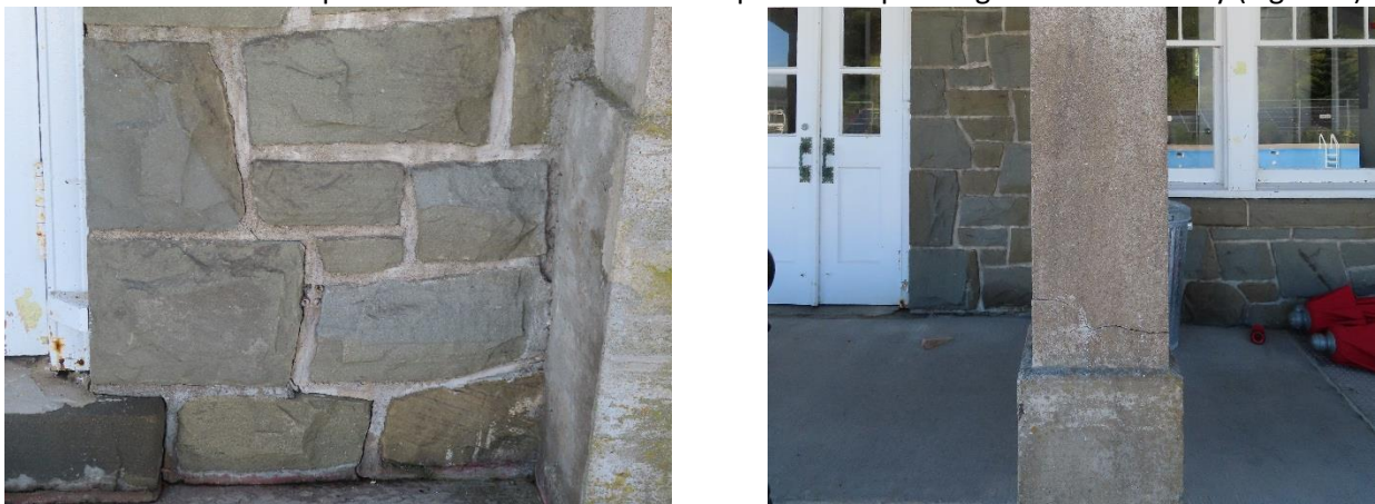
Figure 5: Areas of Stone Masonry and Concrete Deficiencies
