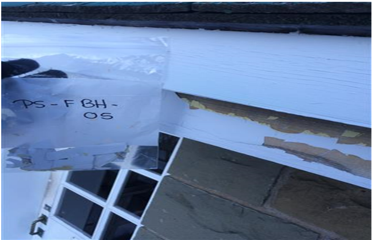
PHOTO 3: View of exterior wood door and frame located outside of Area 2 of the First Floor, sample location of paint sample PS-FBH-05 (White paint chips), which was determined by laboratory analysis to be lead leachate toxic.
