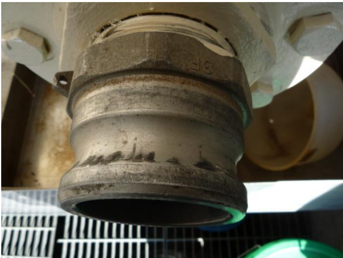
3" Camlock coupler at the dock connection point
