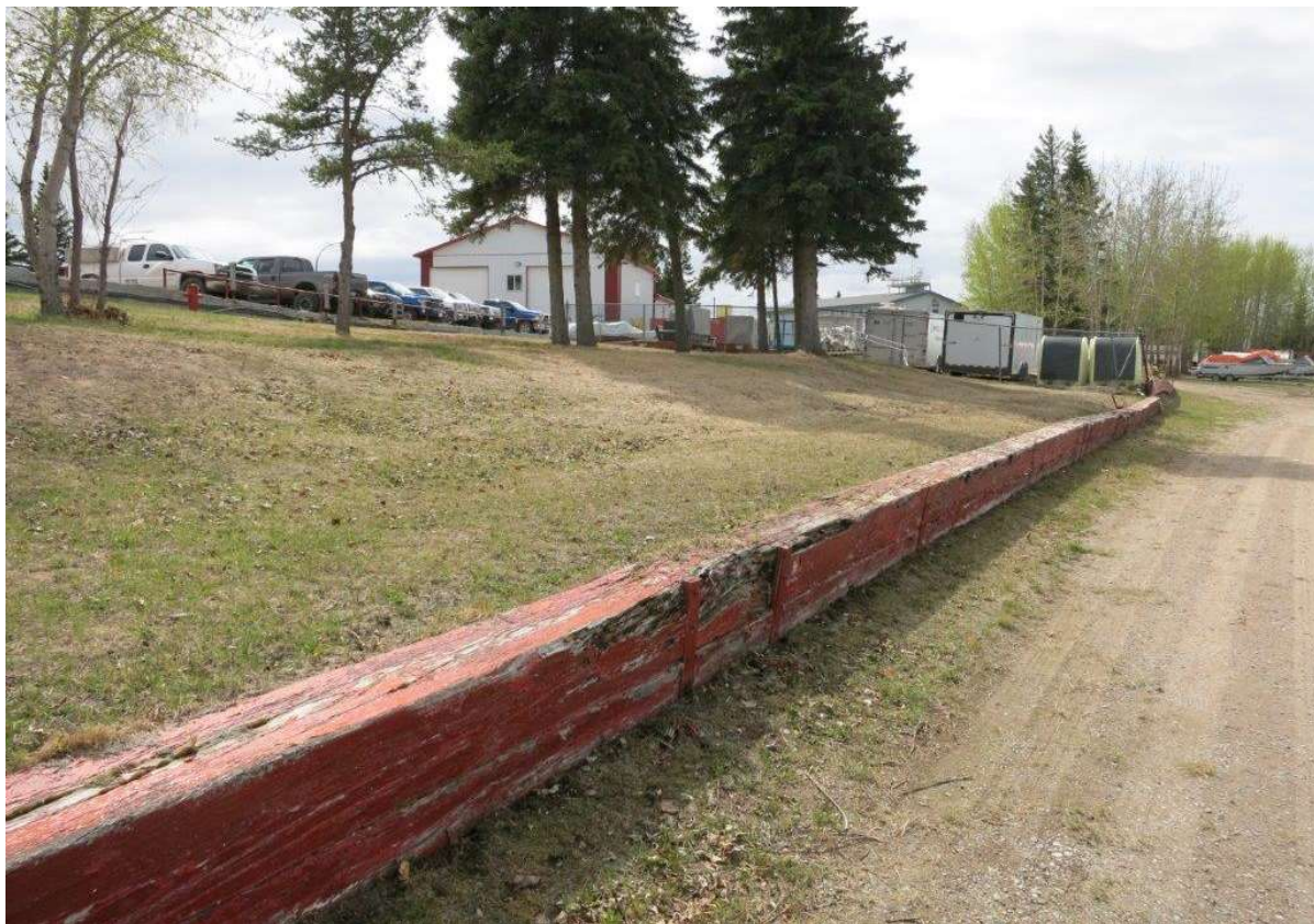
Photo 8: Deteriorated Retaining Wall
