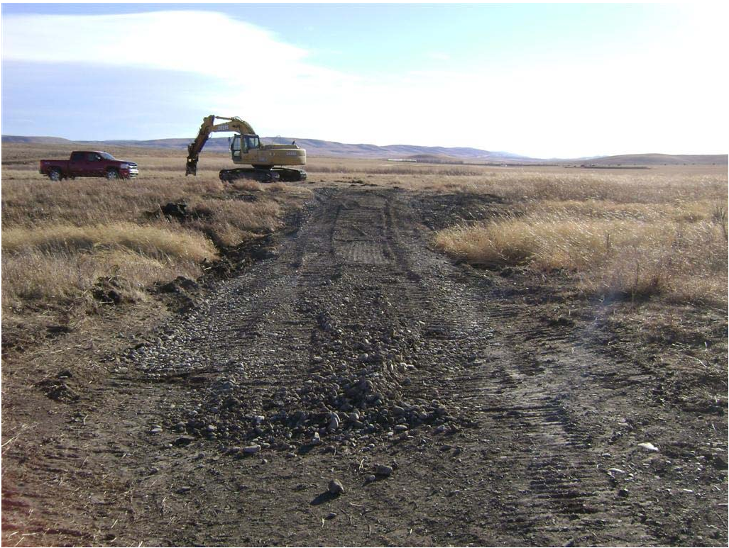
Photo 17: Looking west at gravel fill over new culvert
