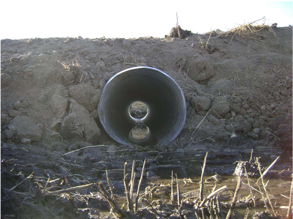
Photo 18: New culvert installed on haul road to borrow pit
