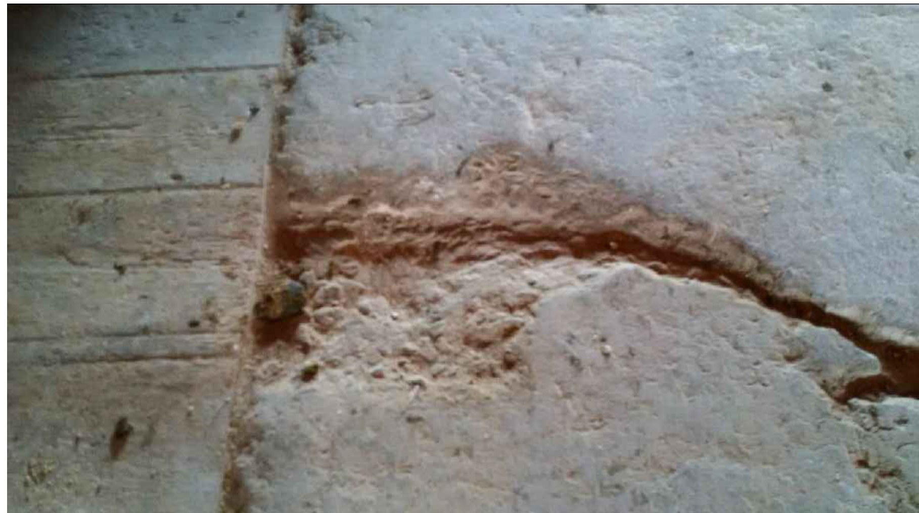
4 SPALLS IN CONCRETE SLAB EX13
