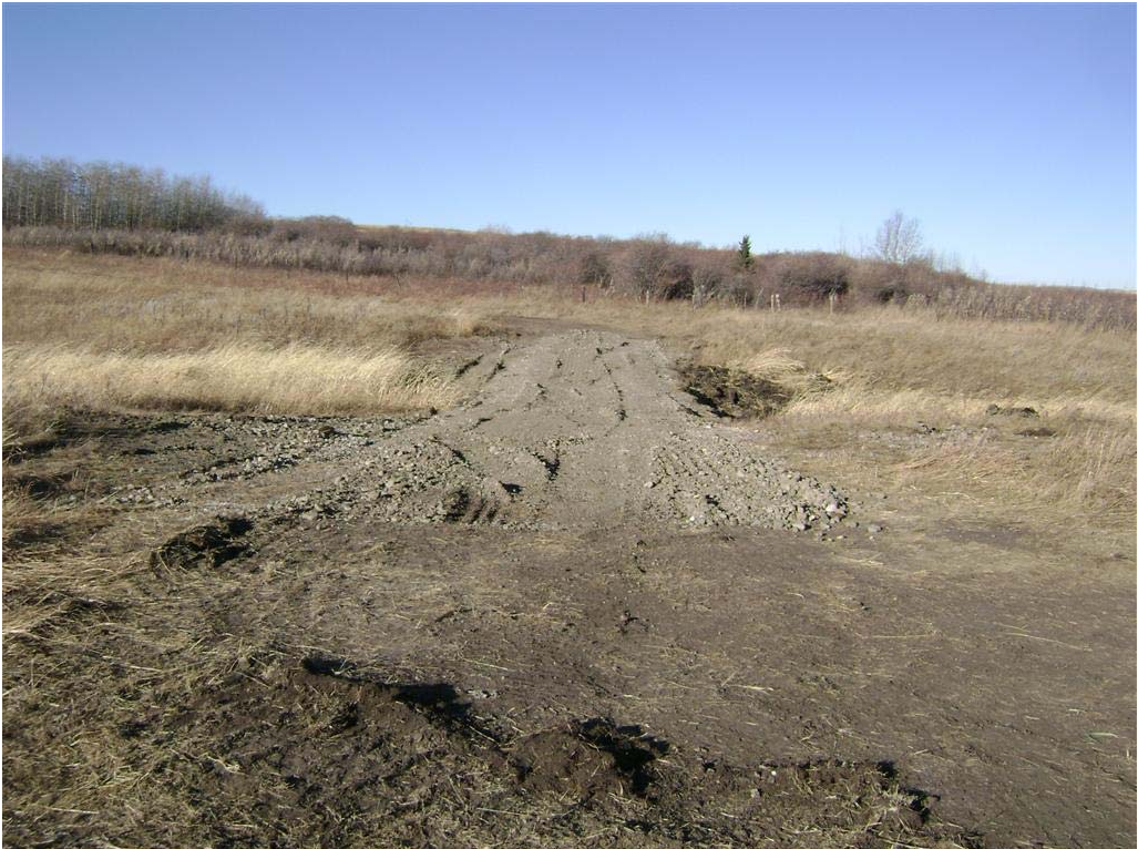
Photo 16: Gravel fill placed along low area over culvert, looking east
