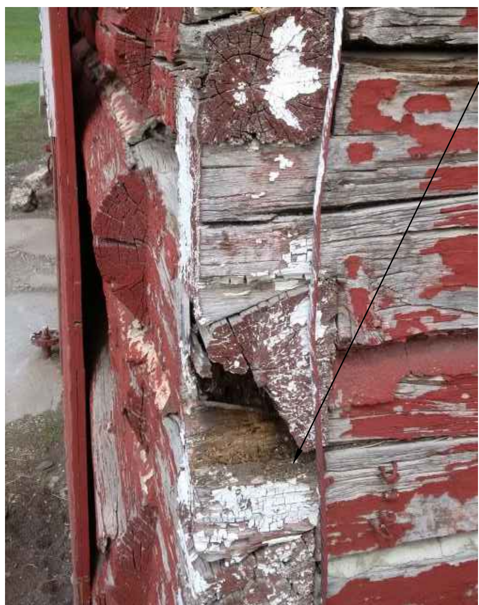
5 DOVETAIL CORNER (S-E) EX21
