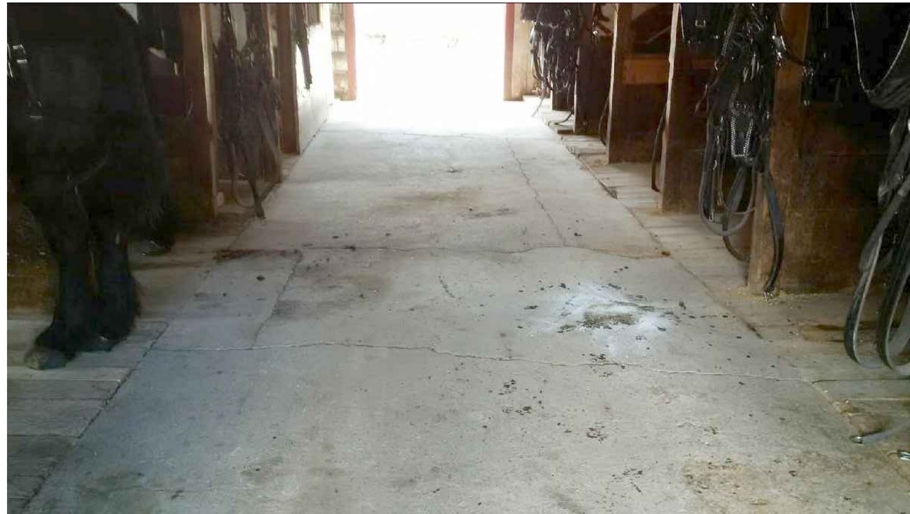
2 CONDITION OF CONCRETE SLAB IN CENTRE AISLE EX13
