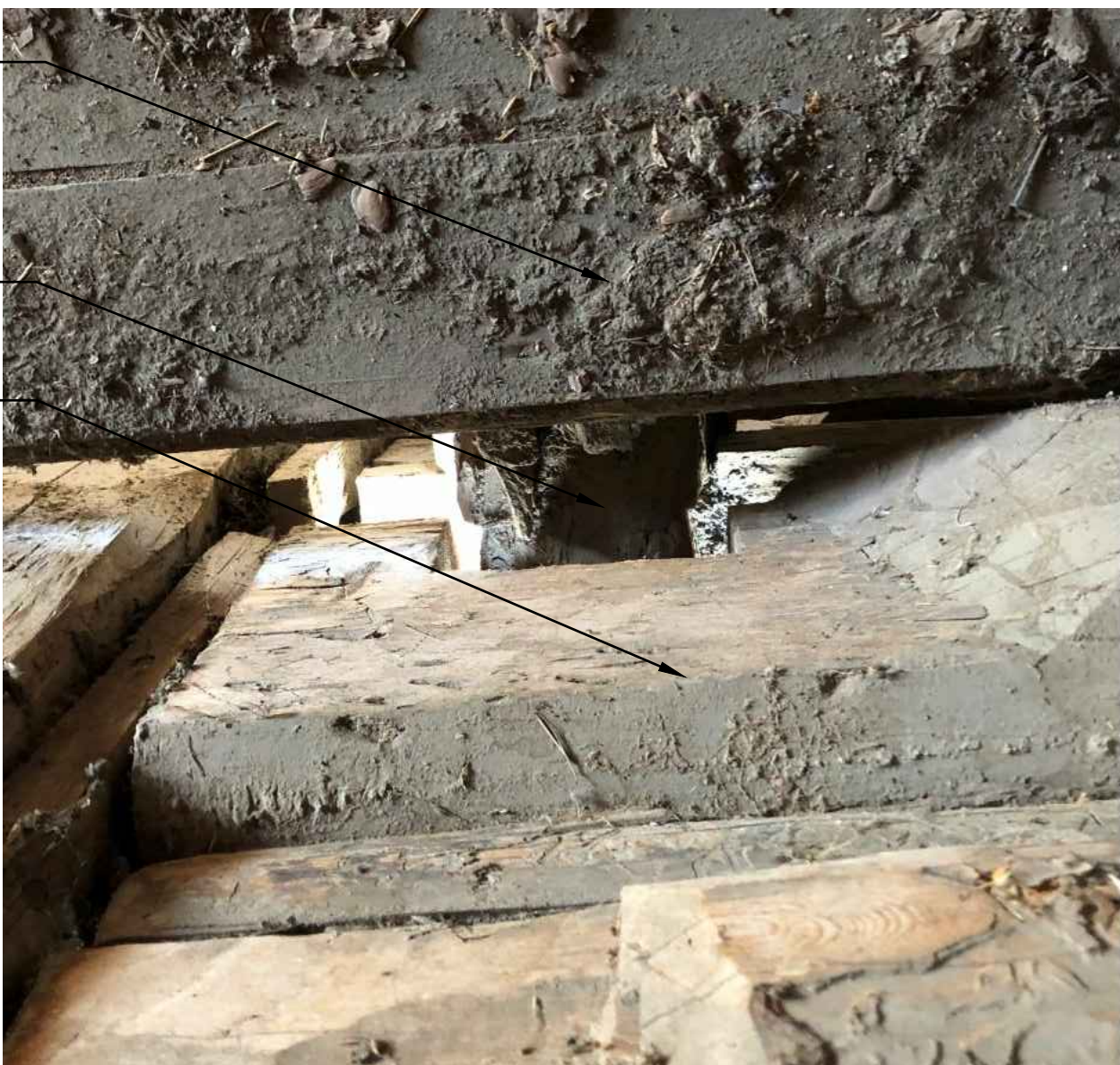
6 JOIST CONNECTION AT WALL (INTERIOR) EX21
