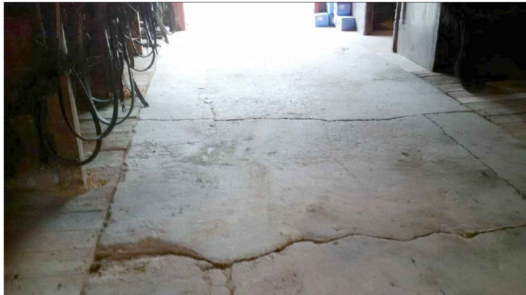
3 LOCALIZED HEAVING OF CONCRETE SLAB EX13
