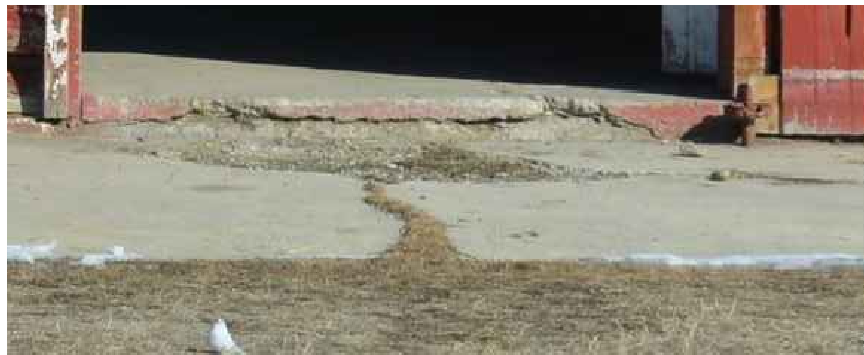
6 CRACKING AND SPALLS IN CONCRETE SLAB EX13
