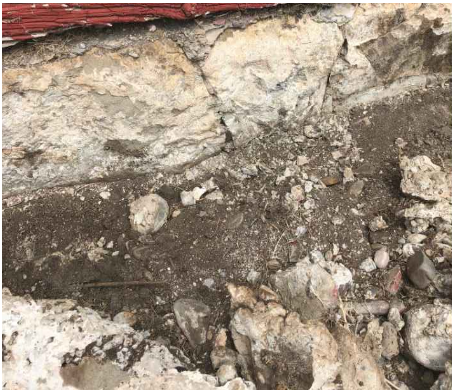
9 SANDSTONE FOUNDATION WITH SOME CONCRETE COVER REMOVED EX21
