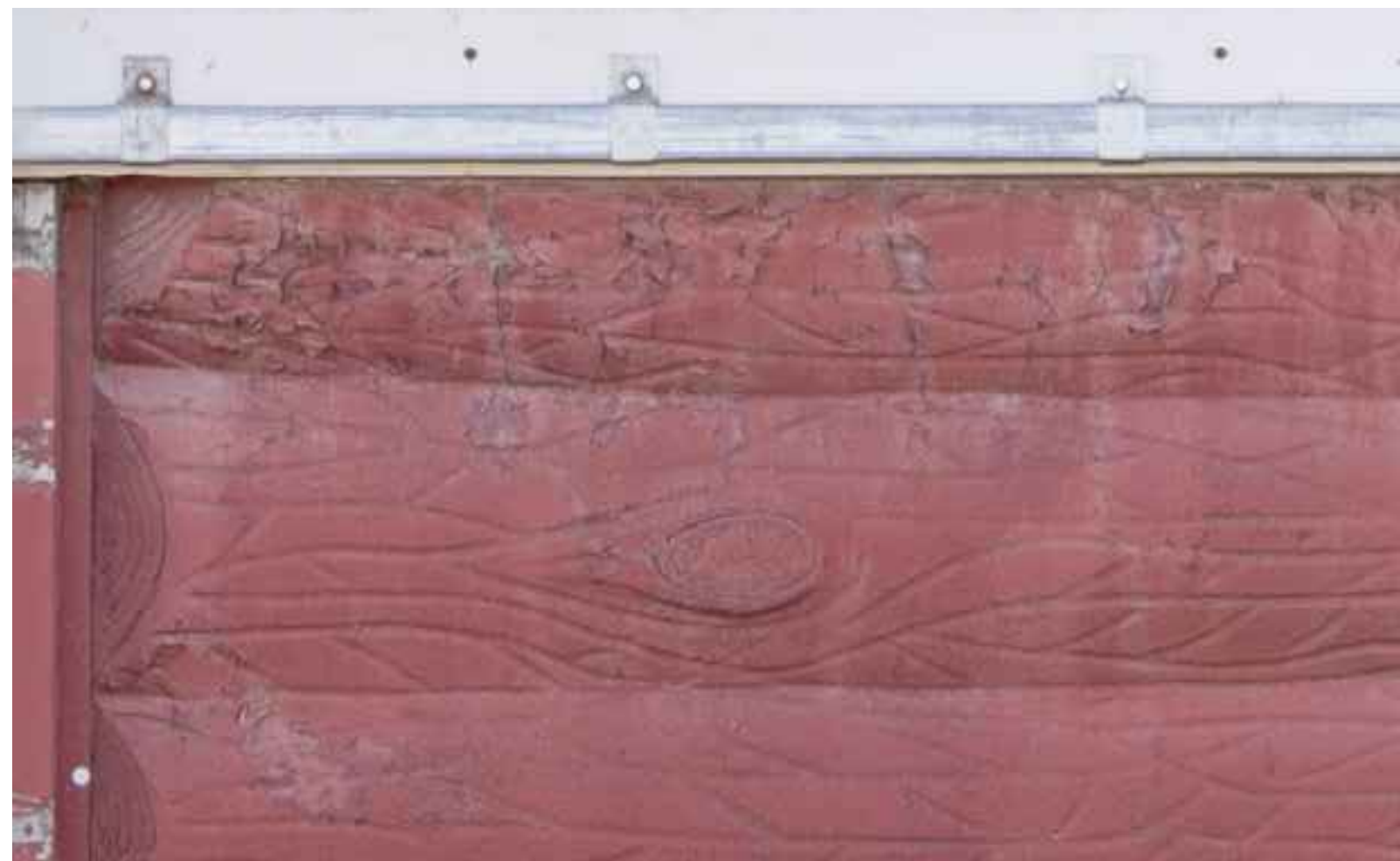
7 EX22 ALLIGATORING AND STREAKING
