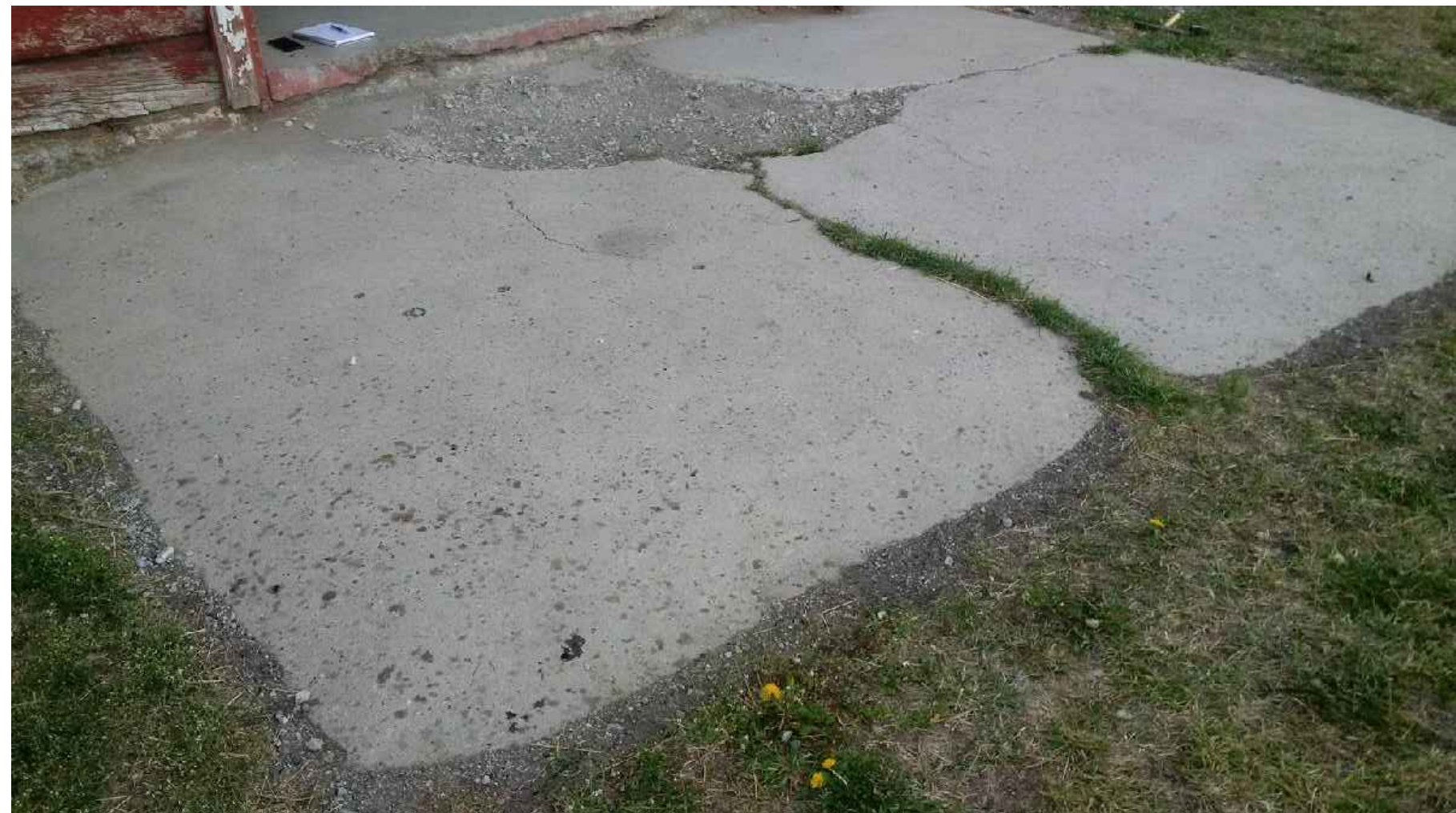
5 CONDITION OF CONCRETE SLAB AT SOUTH ENTRANCE EX13
