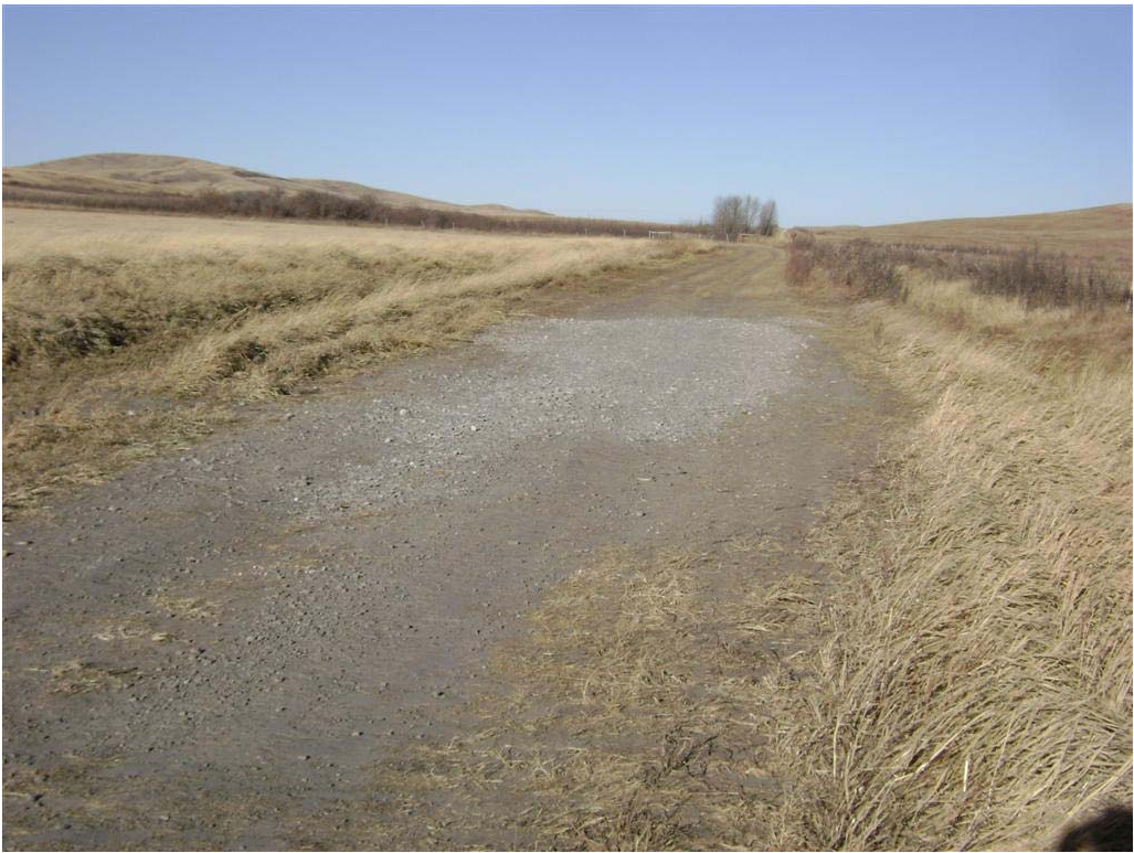
Photo 15: Gravel fill placed in rough section of haul road
