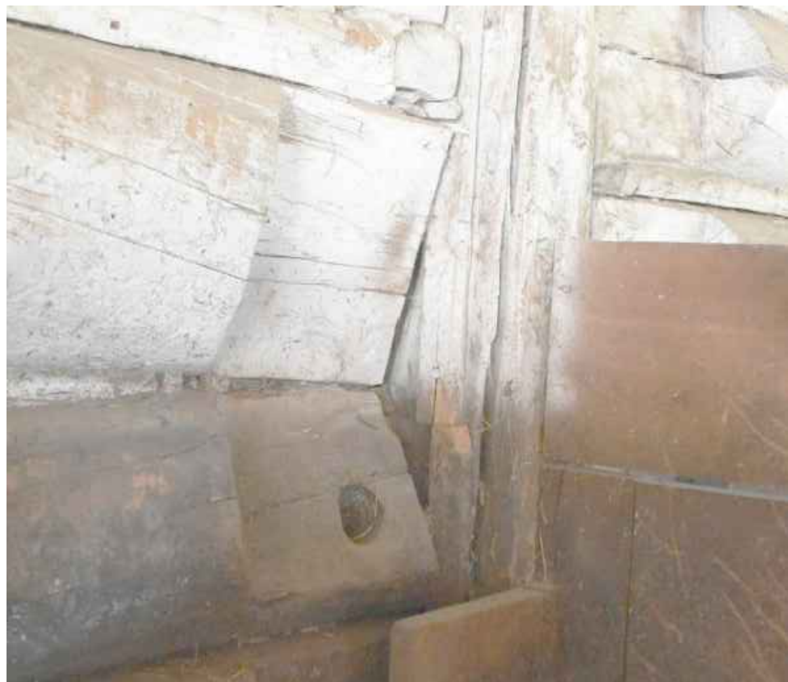
10 TWISTED LOGS ADJACENT TO EAST/WEST ELEVATION POST EX21
