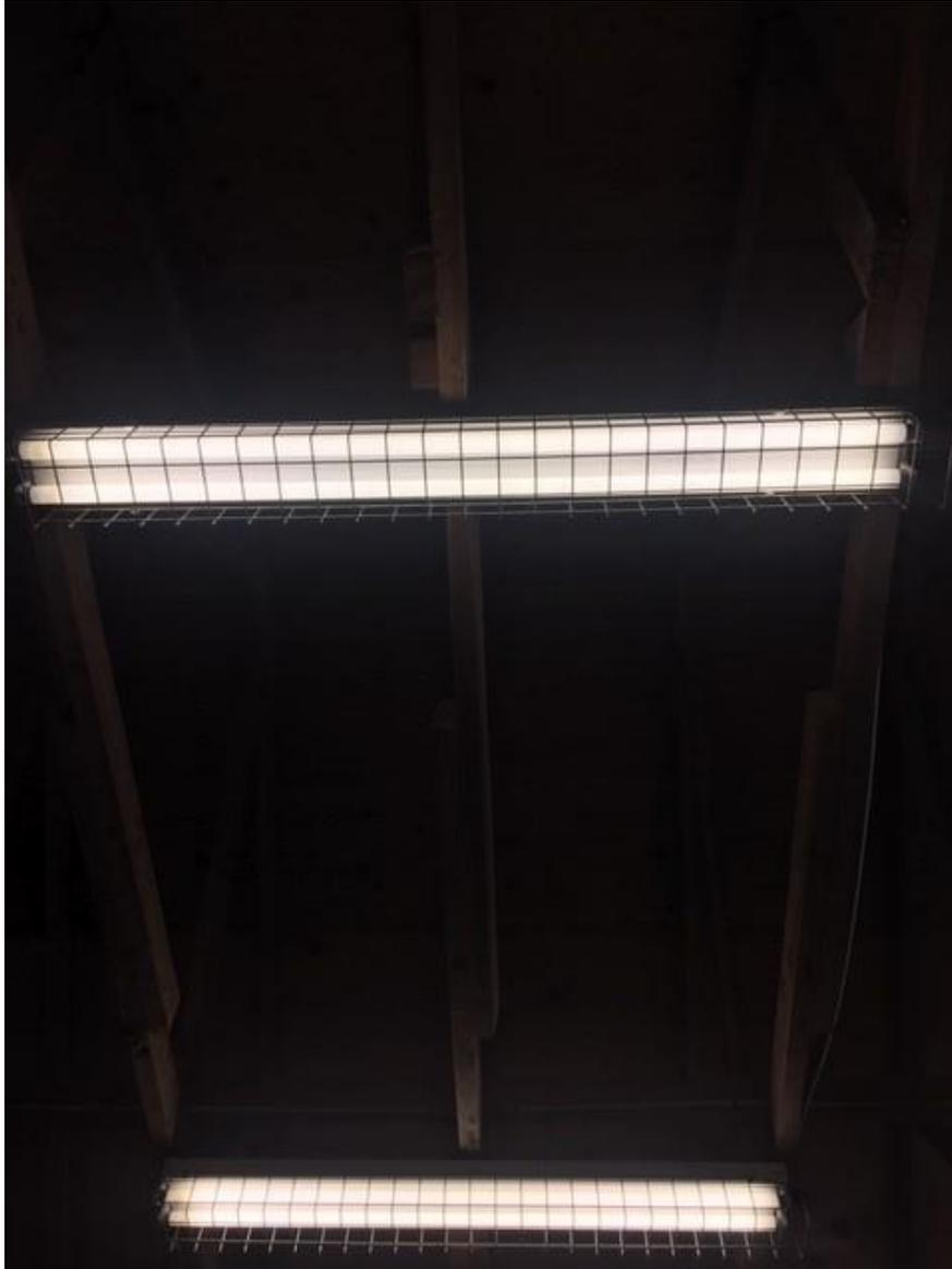
**Photograph #1:** Example of mercury-containing fluorescent light tubes within the building.
