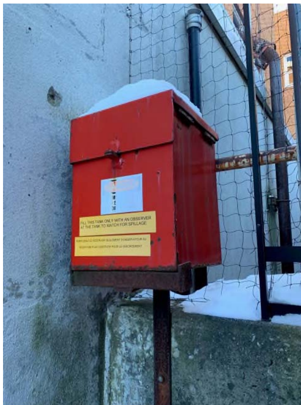
Photo 5: Outside fill pipe spill container at Building 5B
