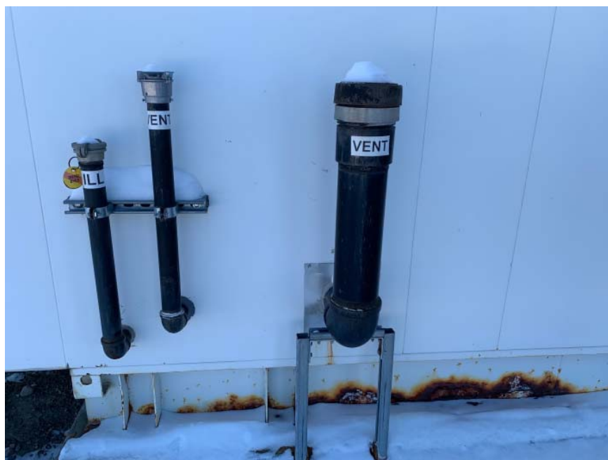
Photo 3: Outside pipe configuration and rust on fuel storage tank system at Building 91/T82F
