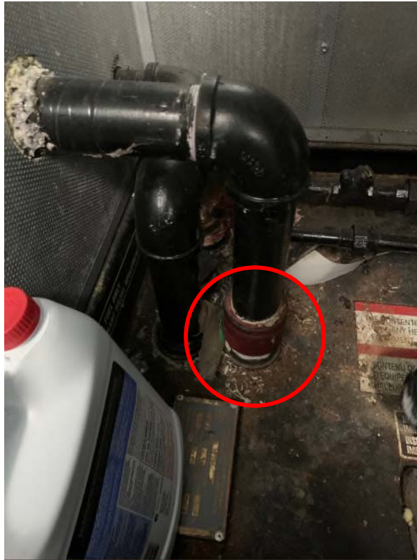
Photo 1: whistle valve (circled) installed on the inside of the fuel storage tank system at Building 91/T82F
