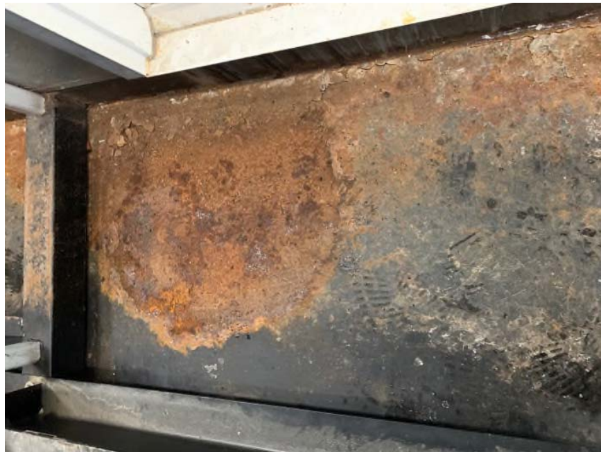
Photo 2: Rust on the floor of the fuel storage tank system at Building 91/T82F
