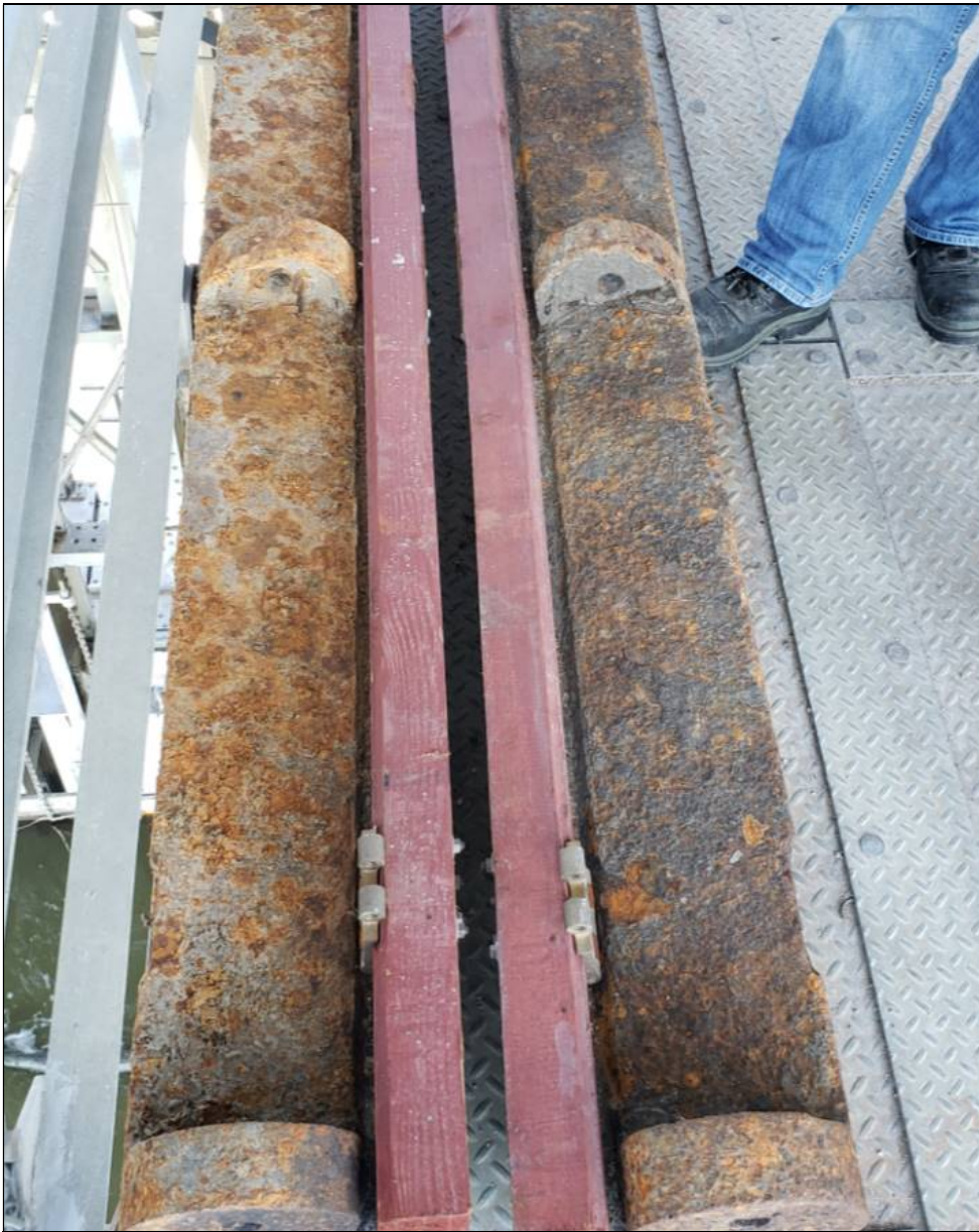
Figure 5: Two existing curtain shoes, both connected to wooden curtain slats
