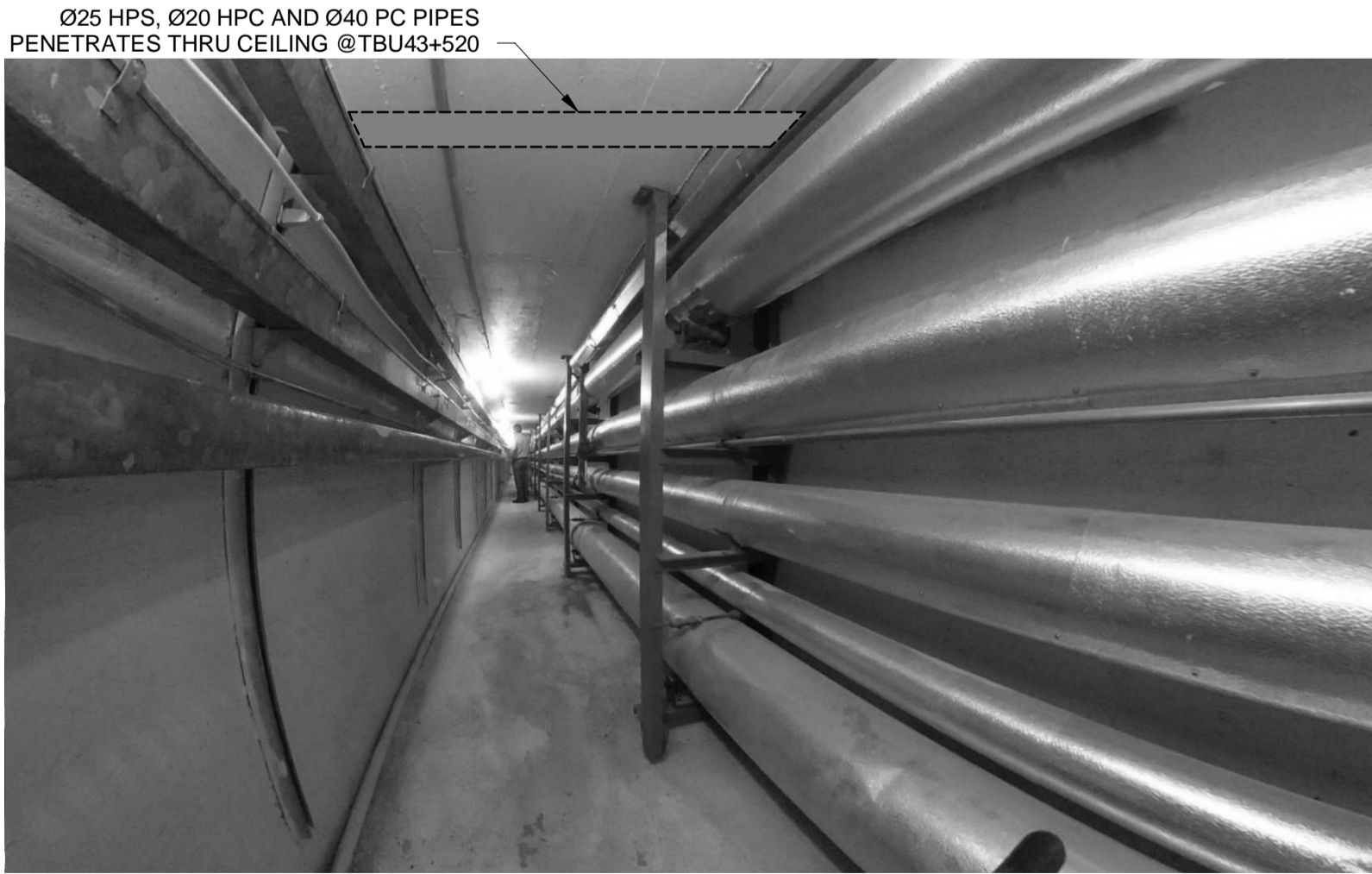
1 FIELD INSTALL CONNECTION POINT @ TBU43+520 Scale: N.T.S.
