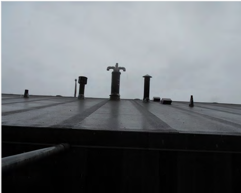
Chimneys and Stacks [F2] 91270-80-810-000002 Furnace Closet 3 - Satisfactory condition-reliable N LOW
