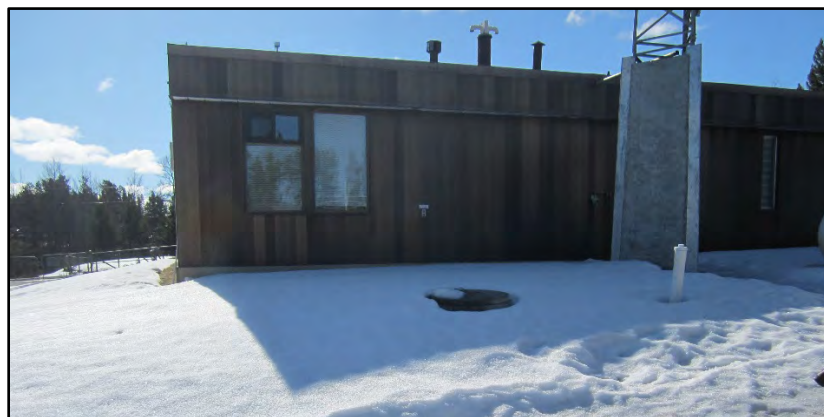
Figure 1: Septic Tank Lid and Cleanout
