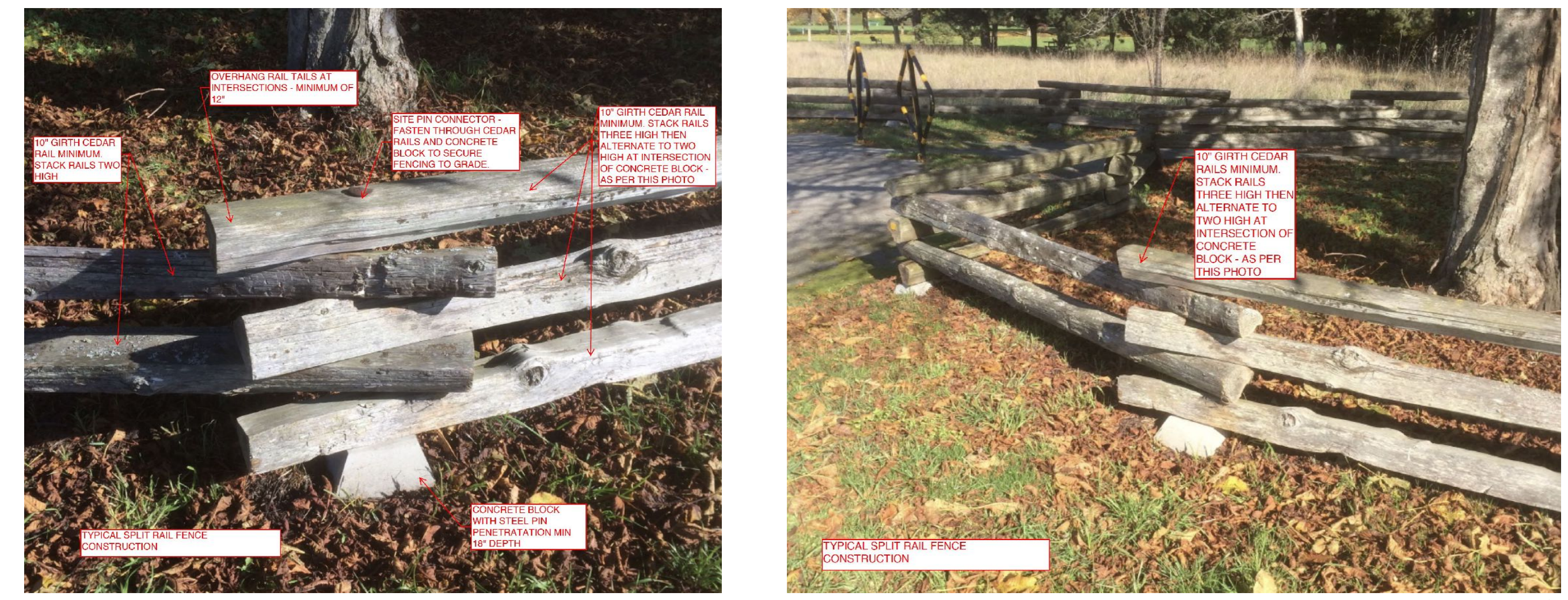
5 TYP. SPLIT RAIL FENCE CONSTRUCTION A1.02
