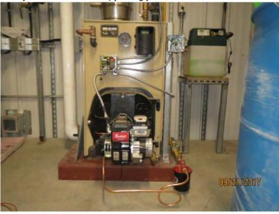
1 X Burner. Beckett Model AFG - Nozzle size 0.75 gph angle 70 deg type B, pump pressure is 100psi.
