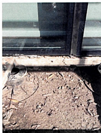
27. Missing Mastic Joint
