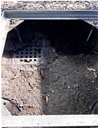
15. Grill Removed Exposing Outlet
