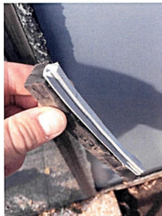
28. Removed Section of Mastic
