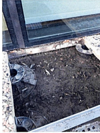
14. Debris Below Paving
