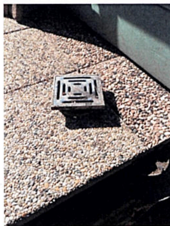
20. Typical Roof Outlet
