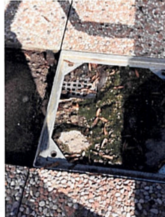
16. Poor Drainage Outlet
