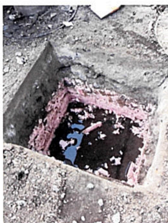
21. Water Found Beneath Insulation
