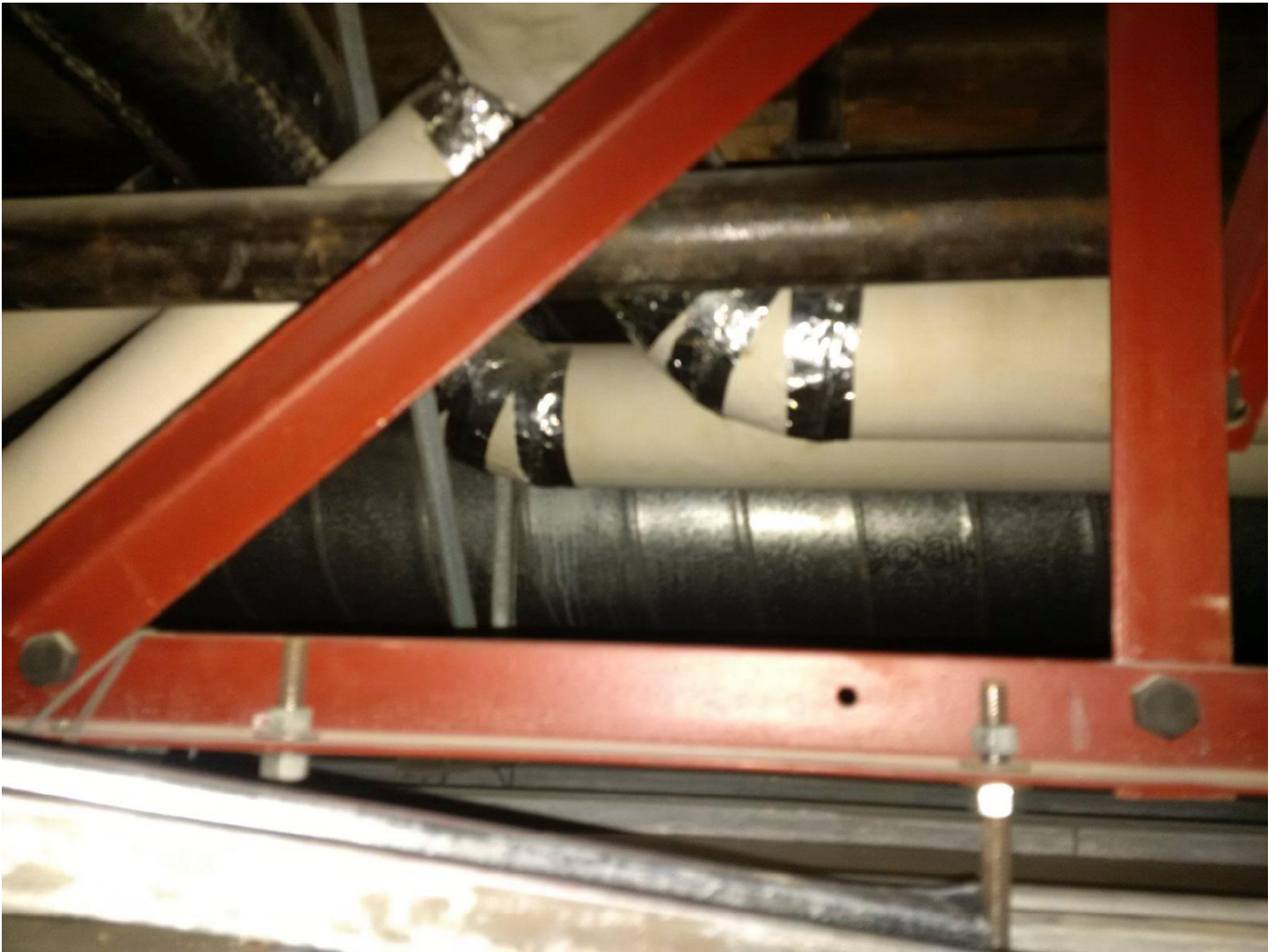
Photo 3: Typical ceiling space above washroom 044, with pipes insulated with fibreglass and bare pipes and ducts.
