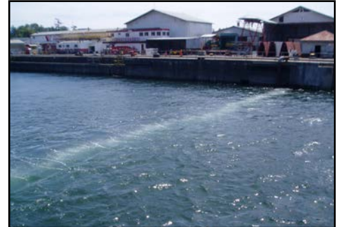
Bubble curtain employed during vessel transfer.
