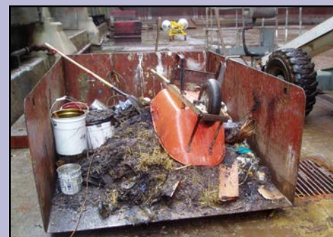
INADEQUATE waste grit storage.
