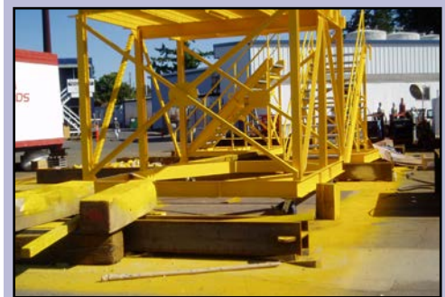
INADEQUATE containment.
