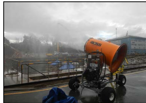
Dust suppression unit in operation.
