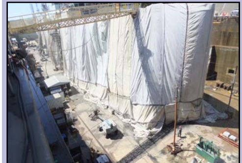
ADEQUATE containment.
