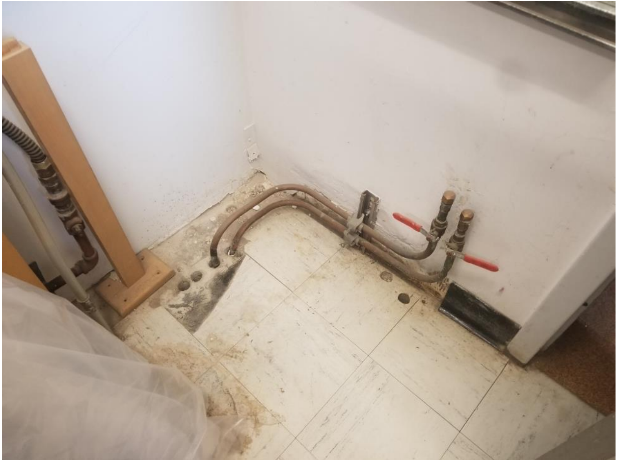
Photo 1. First floor, lab EW-06, next to door on south wall, 4 fair condition vinyl floor tiles.
