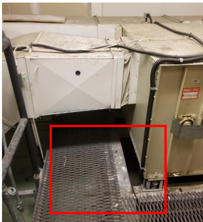
Photo 2. Mezzanine above boiler room, on catwalk, north-east corner, 1 square metre debris.
