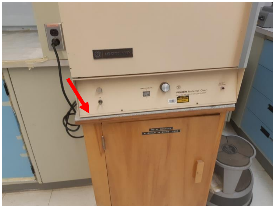
Photo 1. Ground floor, room 9 countertop, 2 linear metres fair condition transite.
