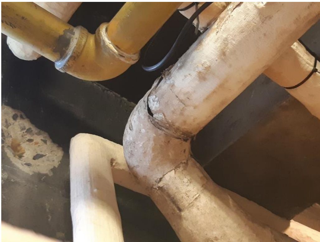
Photo 8. Basement, mechanical room, west wall, 1 fair condition fitting.
