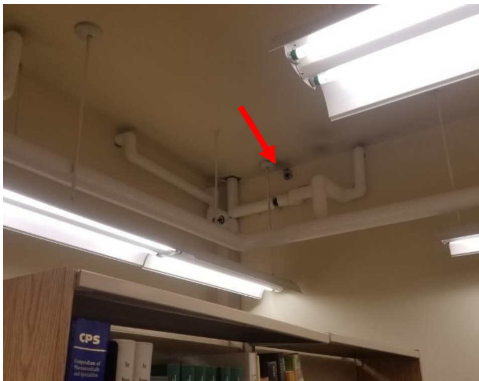
Photo 8. Basement, office 114, east wall in north-east corner, <1 square metre poor condition Aircell in wall penetration.
