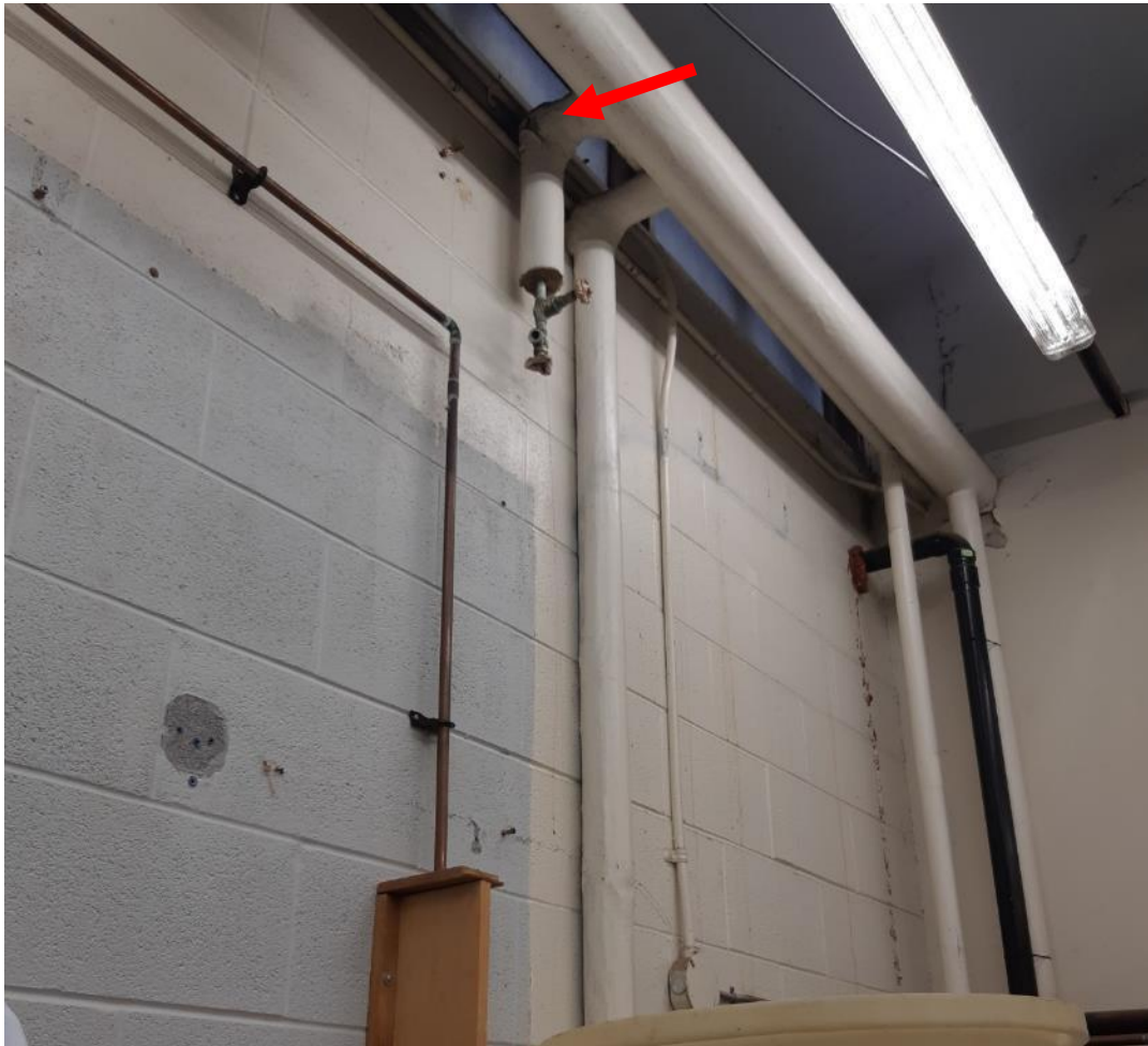
Photo 3. Ground floor, 2 nd floor, south wall, 1 fair condition fitting.
