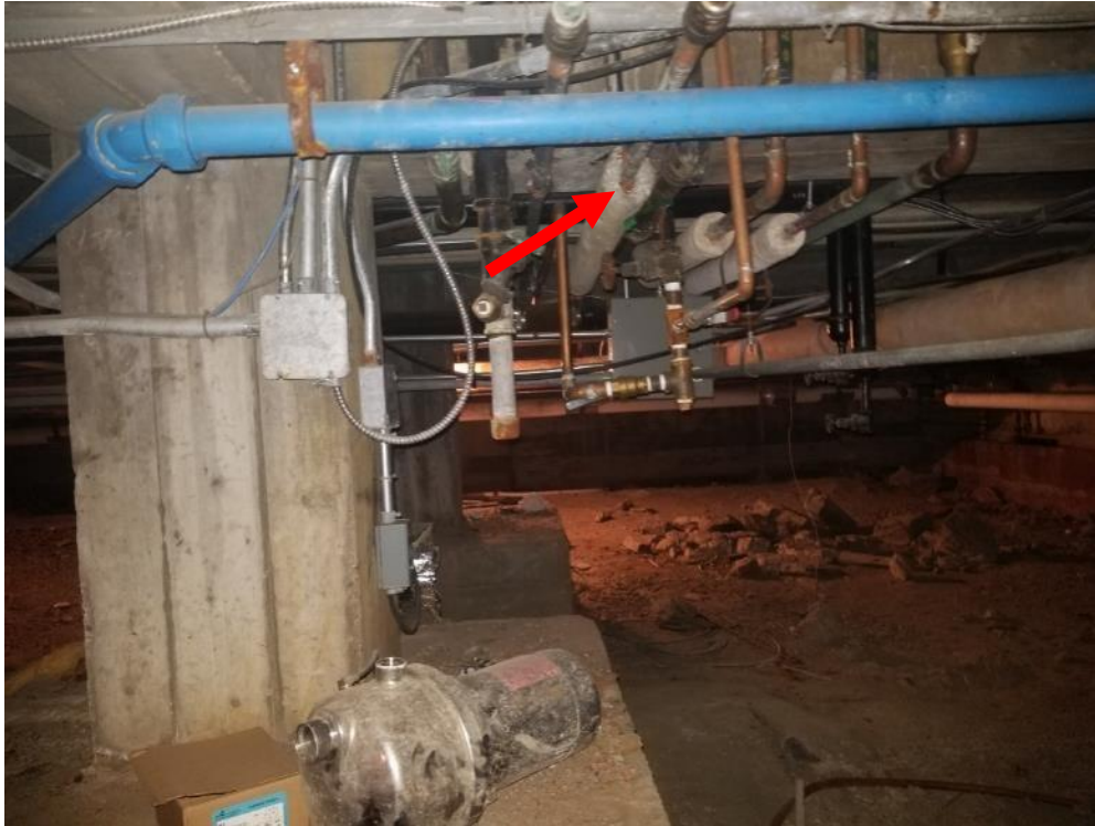
Photo 3. Basement, crawlspace, central, <1 linear metre poor condition Aircell.
