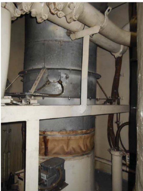
Figure 4: Photograph of in-situ engine room exhaust axial fan
