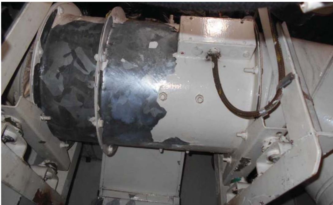
Figure 14: Photograph of in-situ Focsule Deck supply axial fan
