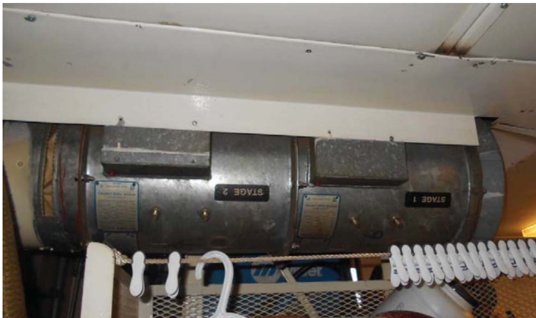
Figure 18: Photograph of in-situ Deck Workshop supply axial fans
