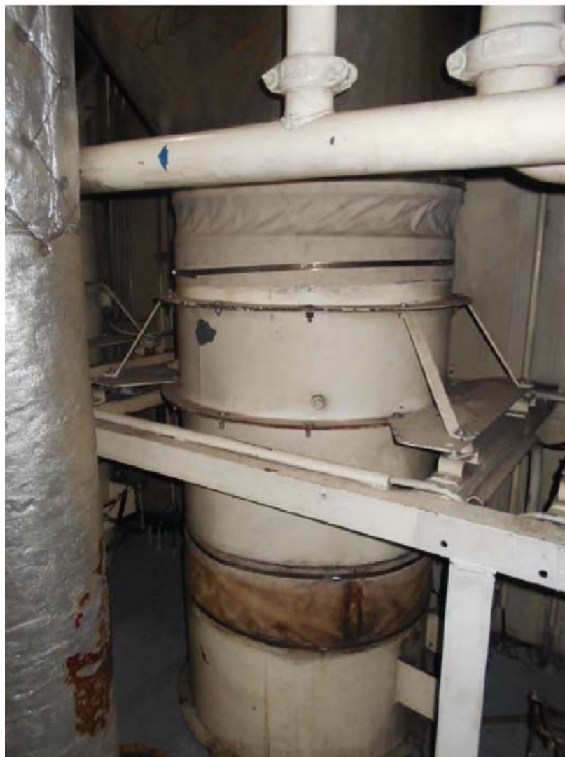
Figure 2: Photograph of in-situ engine room Supply Fan
