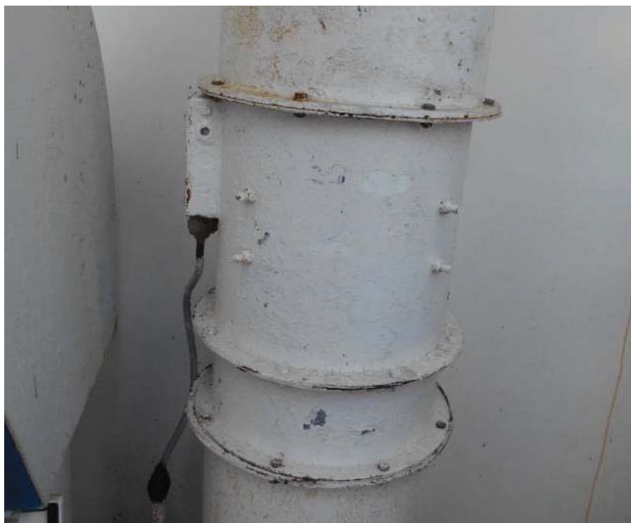
Figure 16: Photograph of in-situ Galley exhaust axial fan – installed on open deck
