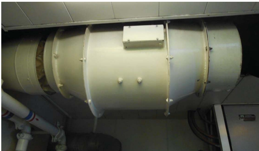
Figure 12: Photograph of in-situ Emergency Generator supply axial fan
