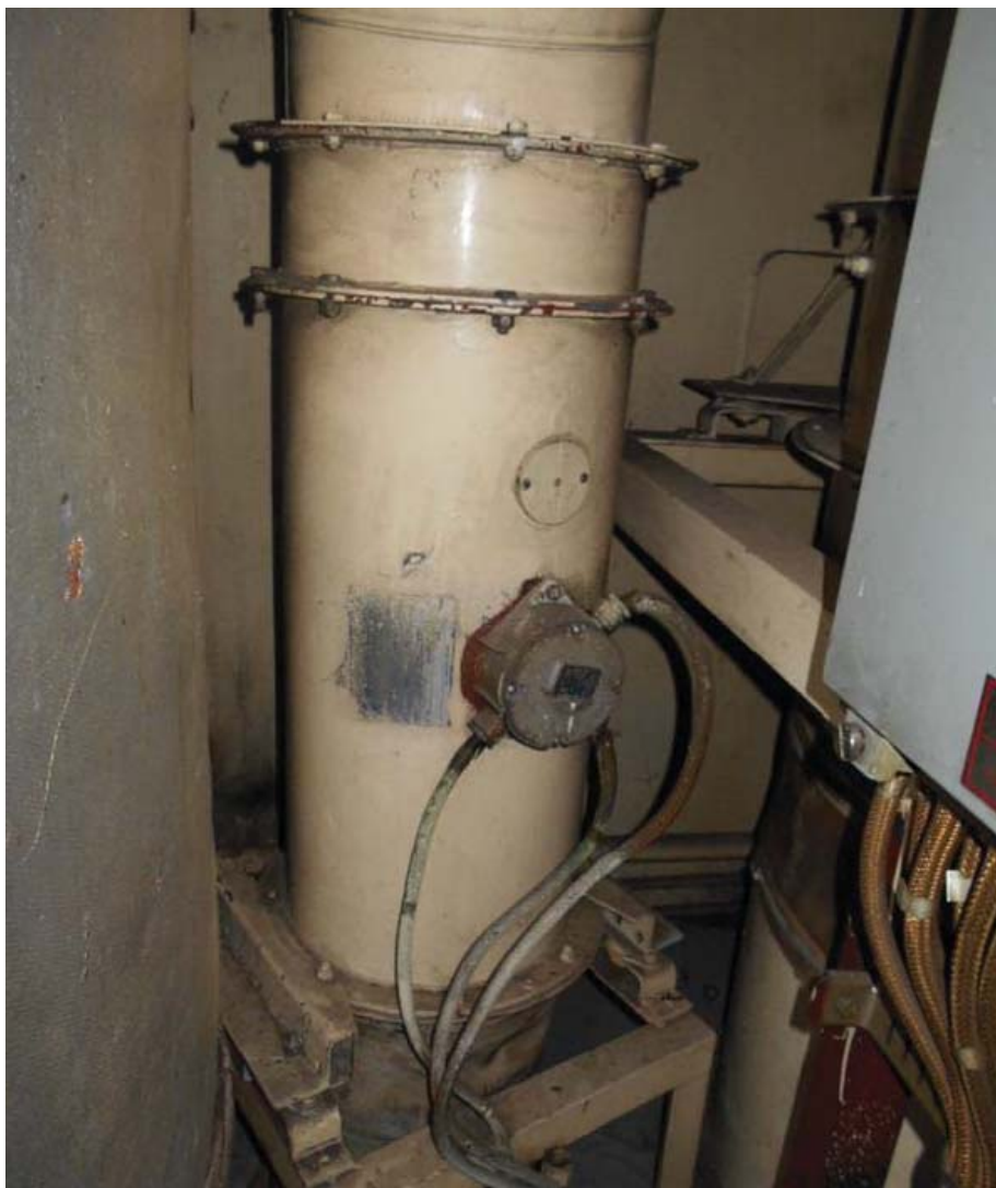
Figure 20: Photograph of in-situ MCR supply axial fan
