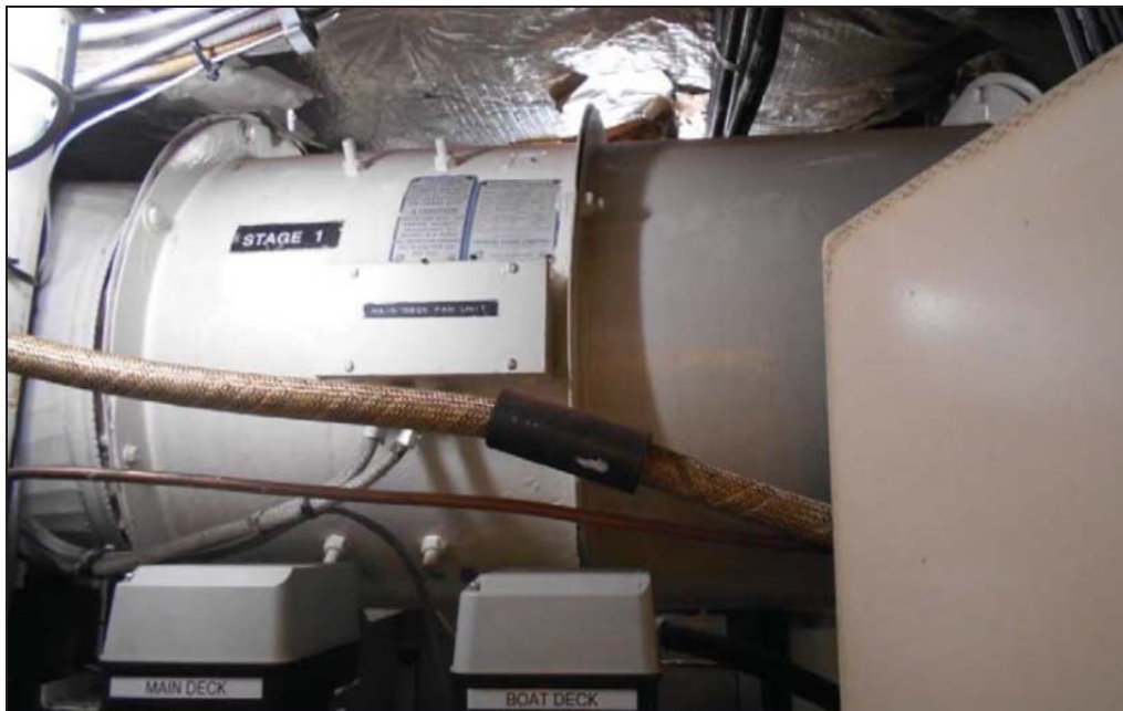
Figure 8: Photograph of in-situ main deck supply axial fan
