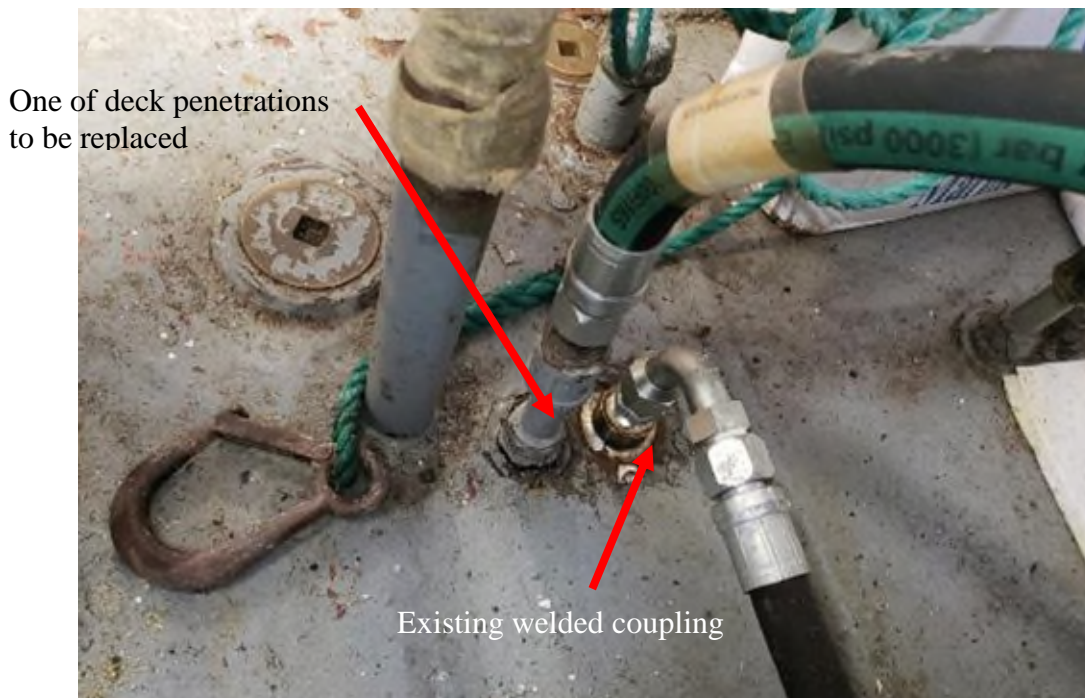
Photograph 4: View of Deck Penetrations
