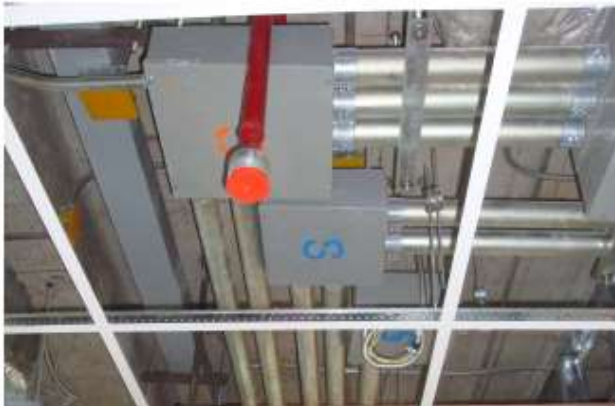
STENCIL SPRAY PAINTED JUNCTION BOXES - BLUE FOR SECURITY
