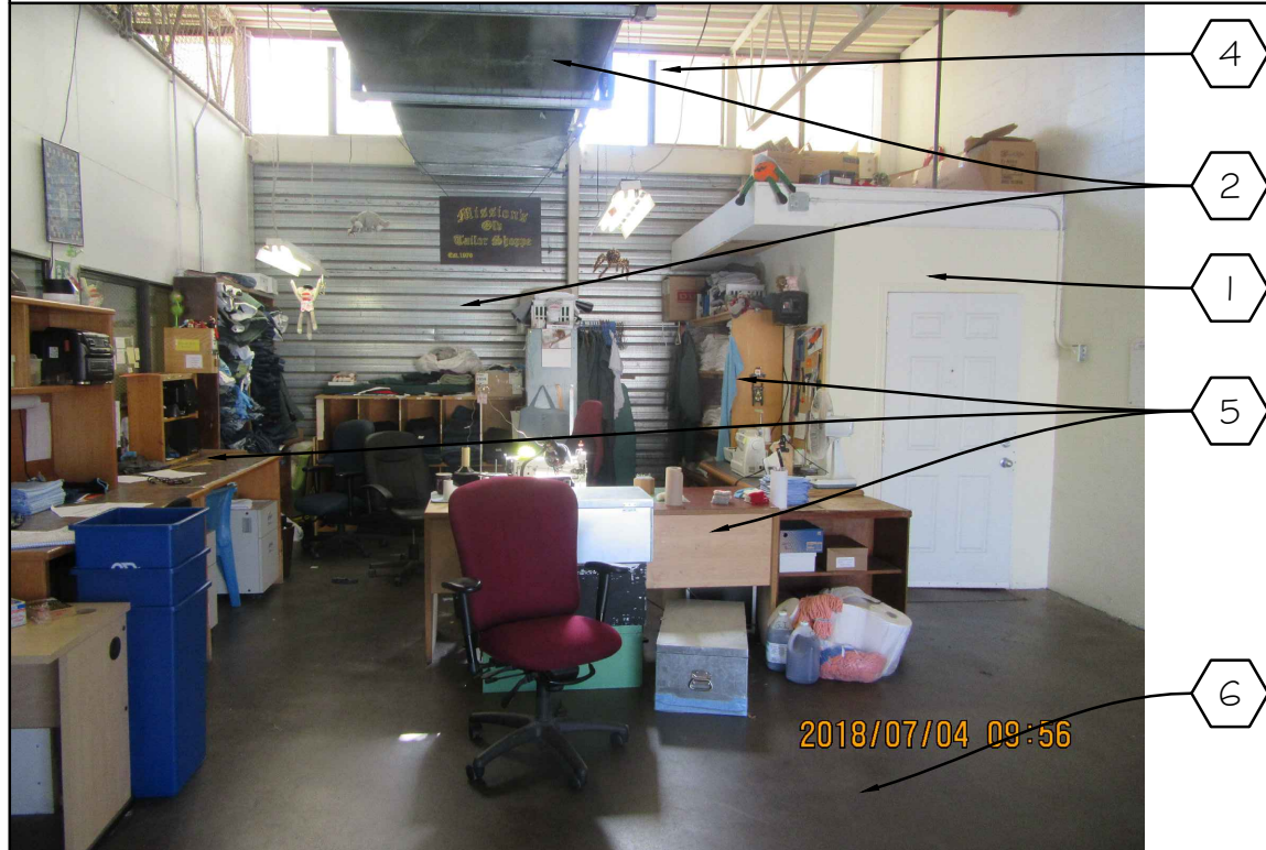
1 PHOTO OF EXISTING CONDITION
