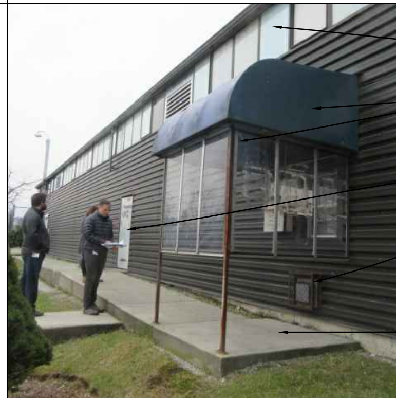
8 PHOTO OF EXISTING CONDITION
