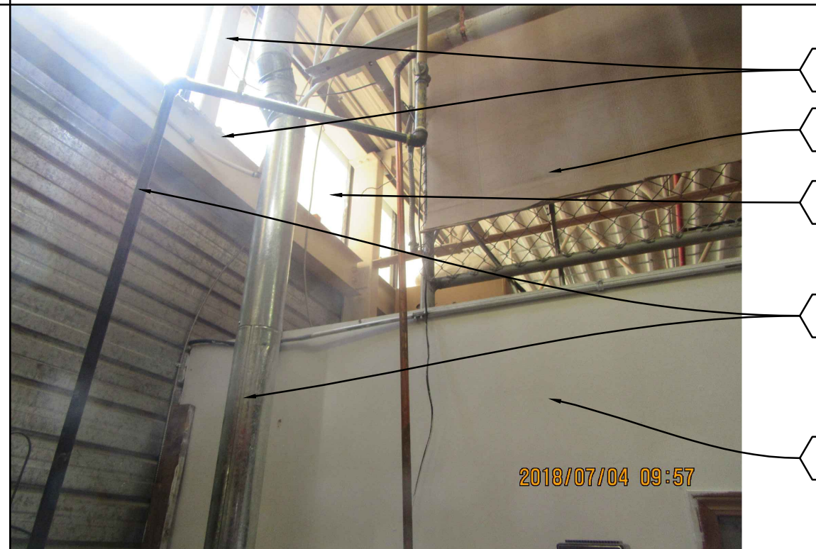
4 PHOTO OF EXISTING CONDITION
