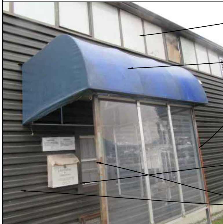
7 PHOTO OF EXISTING CONDITION
