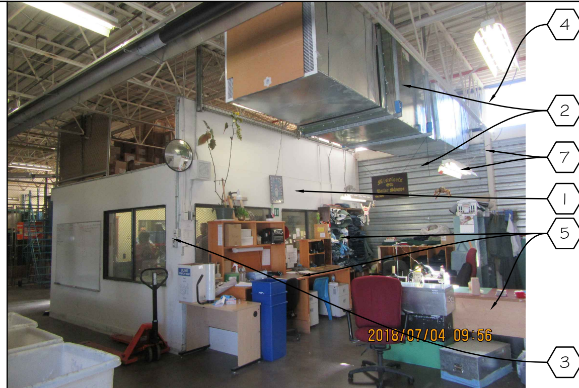
2 PHOTO OF EXISTING CONDITION
