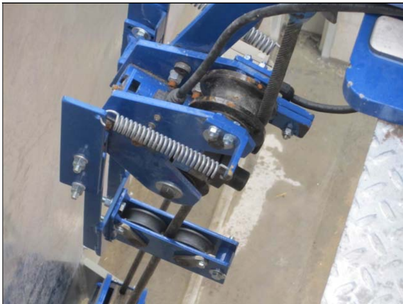
Figure 14: Big Chaudière South Dam, slack rope limit device.
