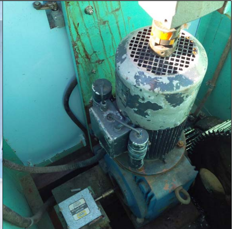
Figure 7: Portage Dam, detail of hoist motor
