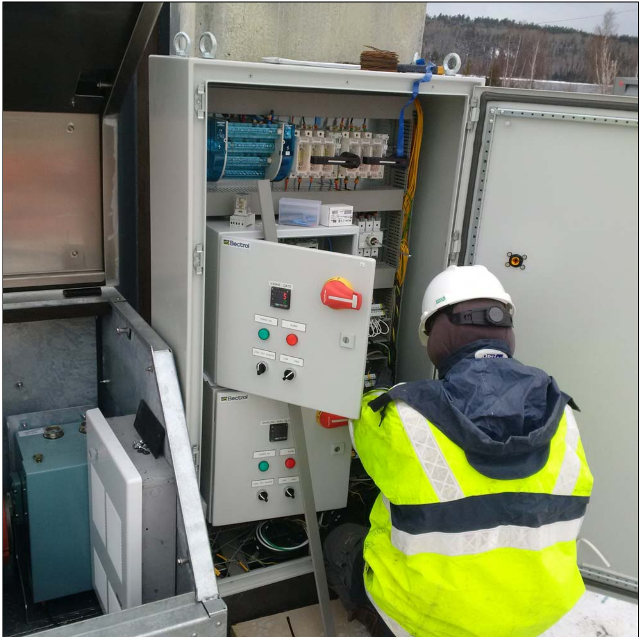
Figure 25: Latchford Dam gate control panel during construction in December 2016.
