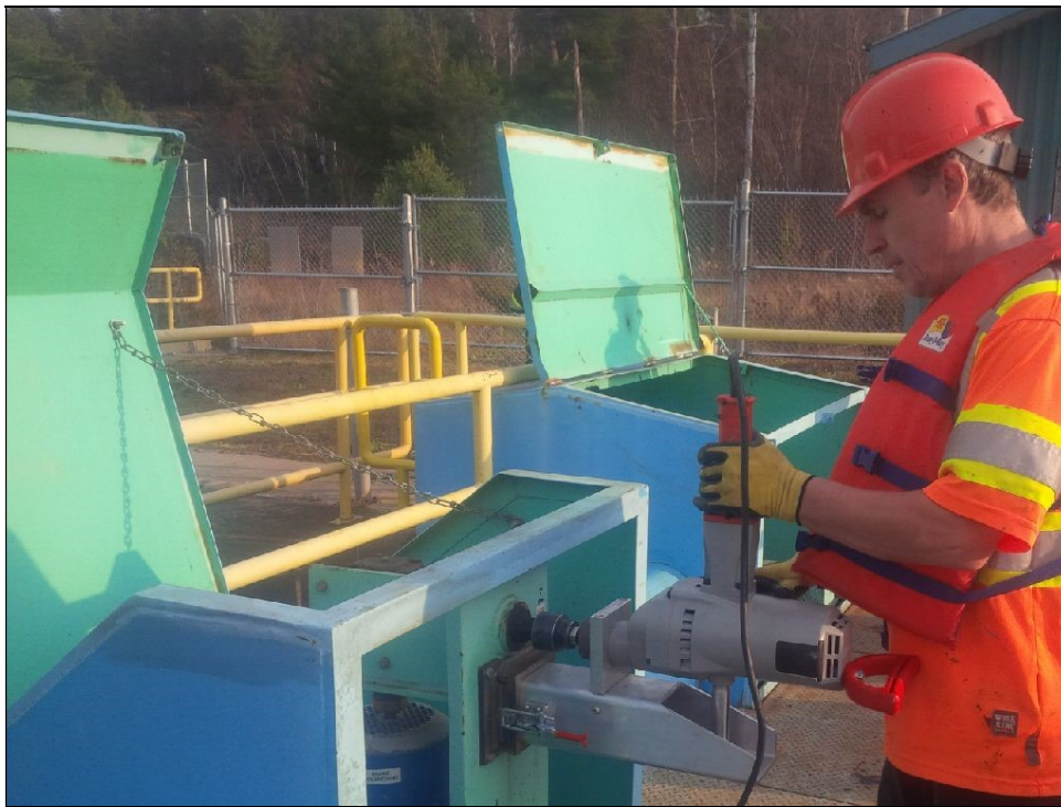
Figure 8: Portage Dam gates being operated through backup operating mechanism.
