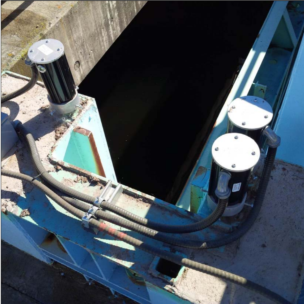
Figure 9: Portage Dam, gate gains with cover removed showing top of gain heaters.
