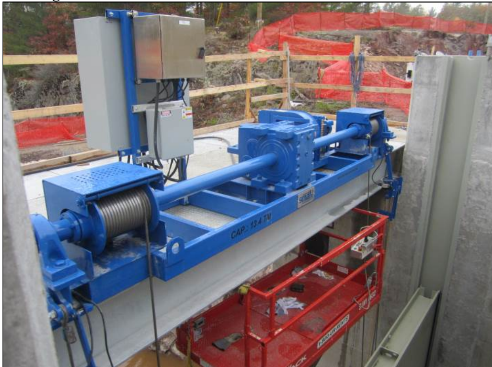
Figure 10: Big Chaudière South Dam gate hoist being installed.
