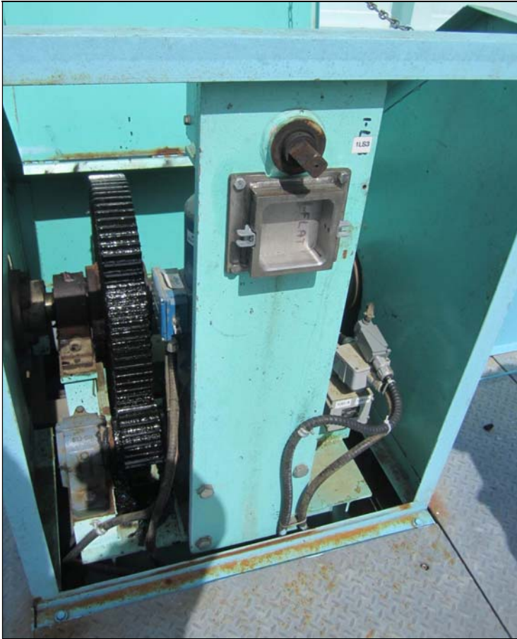
Figure 18: Little Chaudière Dam, hoist machinery with front of enclosure removed and lid lifted.
