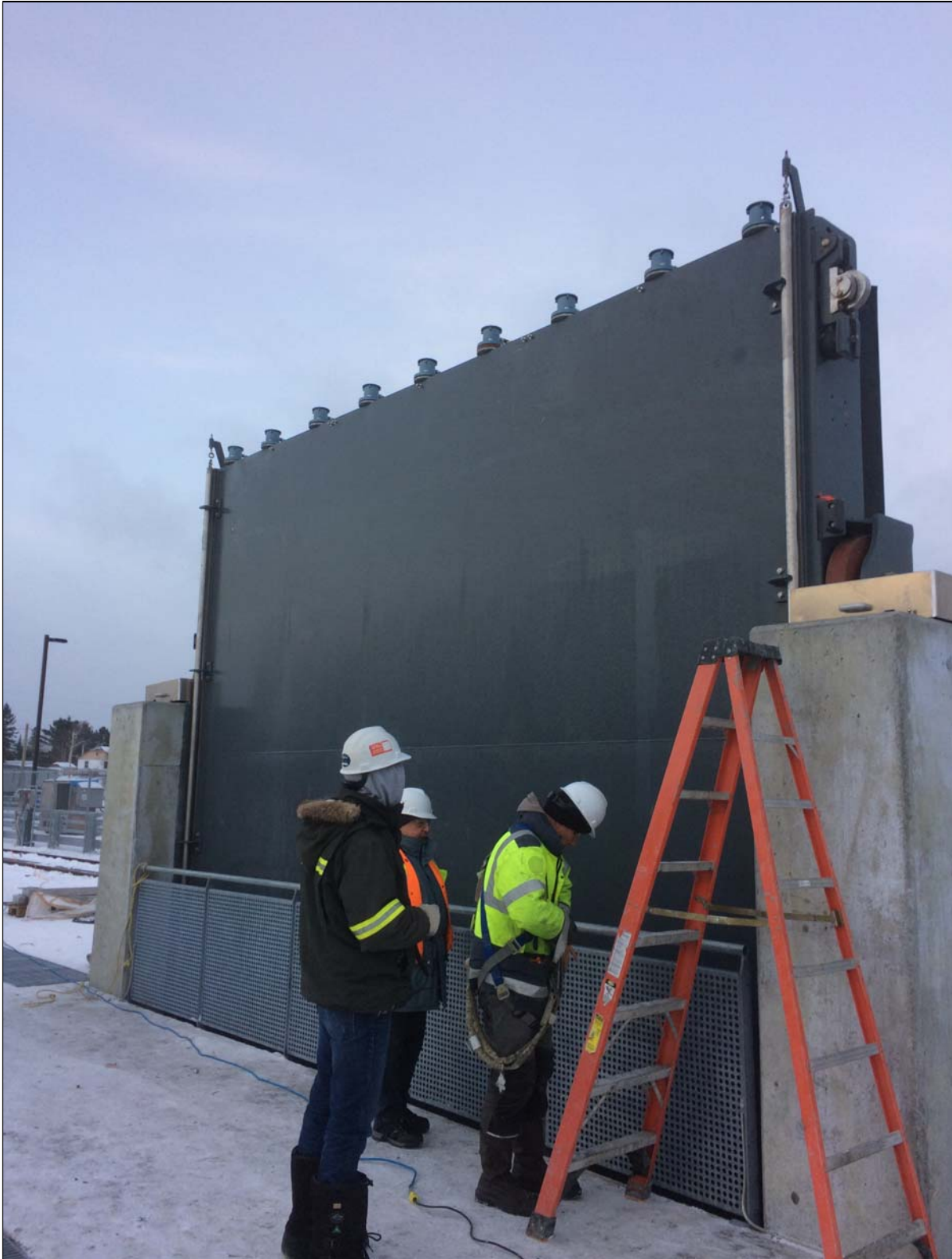
Figure 24: Latchford Dam gate being installed on site, early December 2016. Note heads of gate heaters on top.
