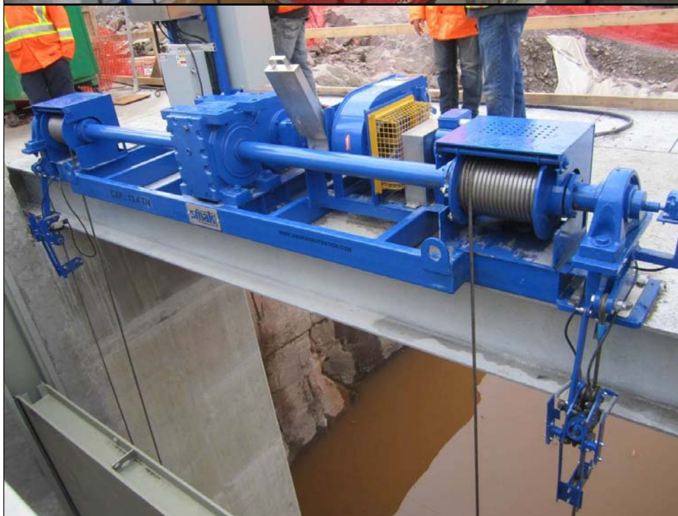
Figure 11: Big Chaudière South Dam gate hoist being installed.
