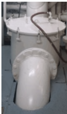
Starboard Side Strainer
