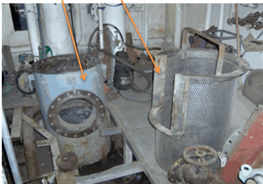
Figure 1.1 Strainer Body and inner strainer basket
