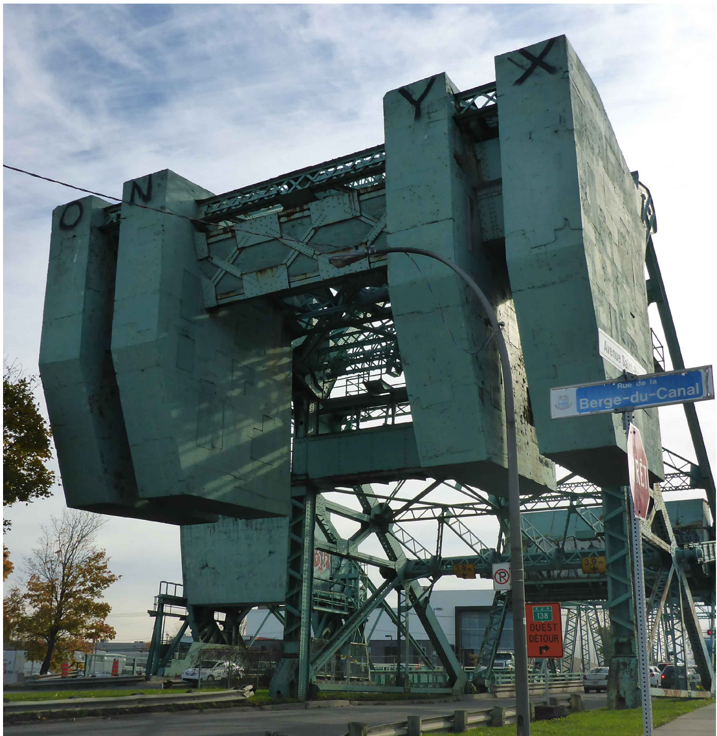
ÉLÉVATION NORD DU CONTREPOIDS / NORTH ELEVATION OF COUNTERWEIGHT
