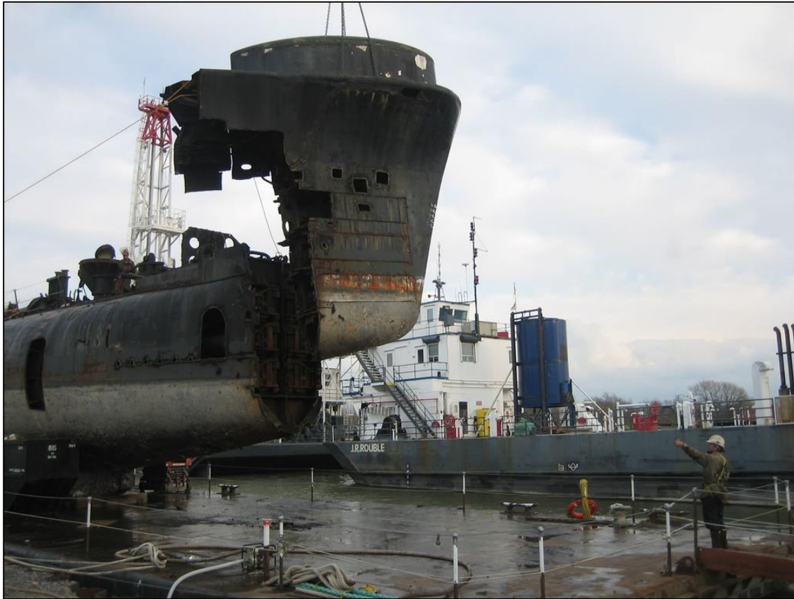
Figure 1: An Oberon Class submarine being scrapped at the MRC facility
