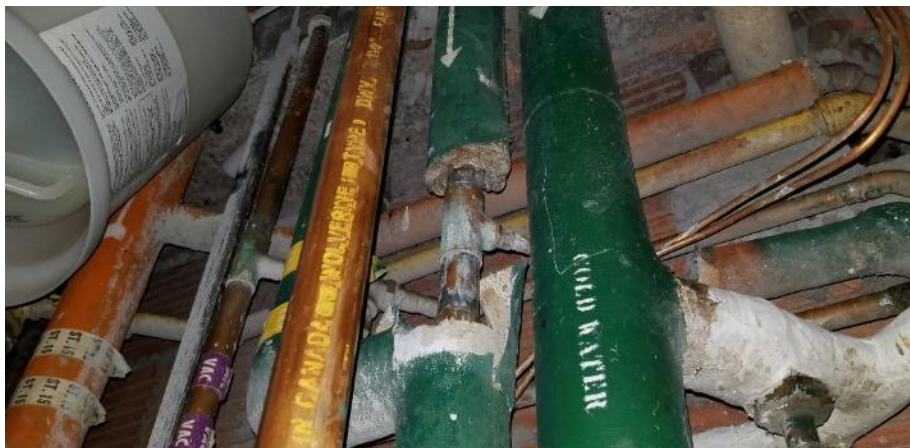
Photo 73: Pipe chase 4037-4039, Poor Condition Aircell Pipe Insulation and Pipe Fitting
