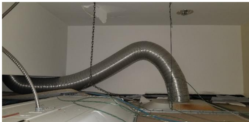
Photo 81: Room 4107, Poor Condition Ceiling Plaster and Plaster Debris located on and above ceiling tiles
