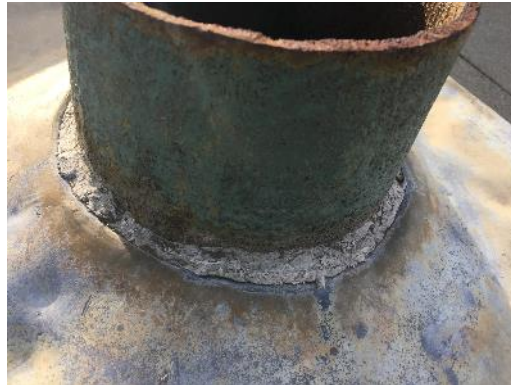
Non-asbestos brown oakum on a rooftop pipe
