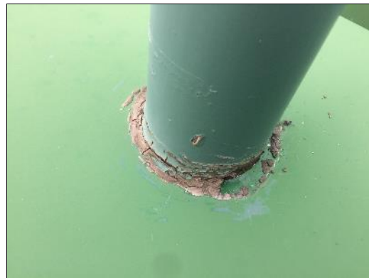
Non-asbestos brown caulking (sample S0005).
