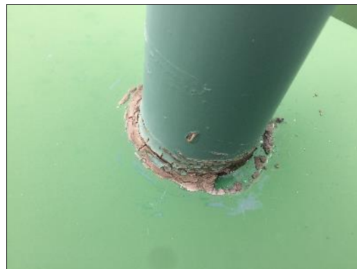
Non-PCB brown caulking.
