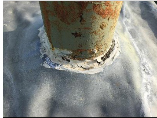
View of non-asbestos white caulking (sample S0003) surrounding a pipe.
