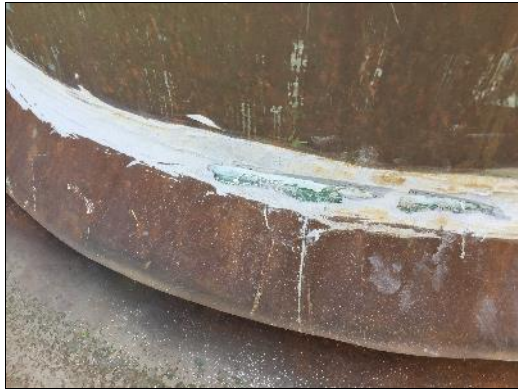
Non-asbestos light grey (sample S0002) caulking found on the roof.
