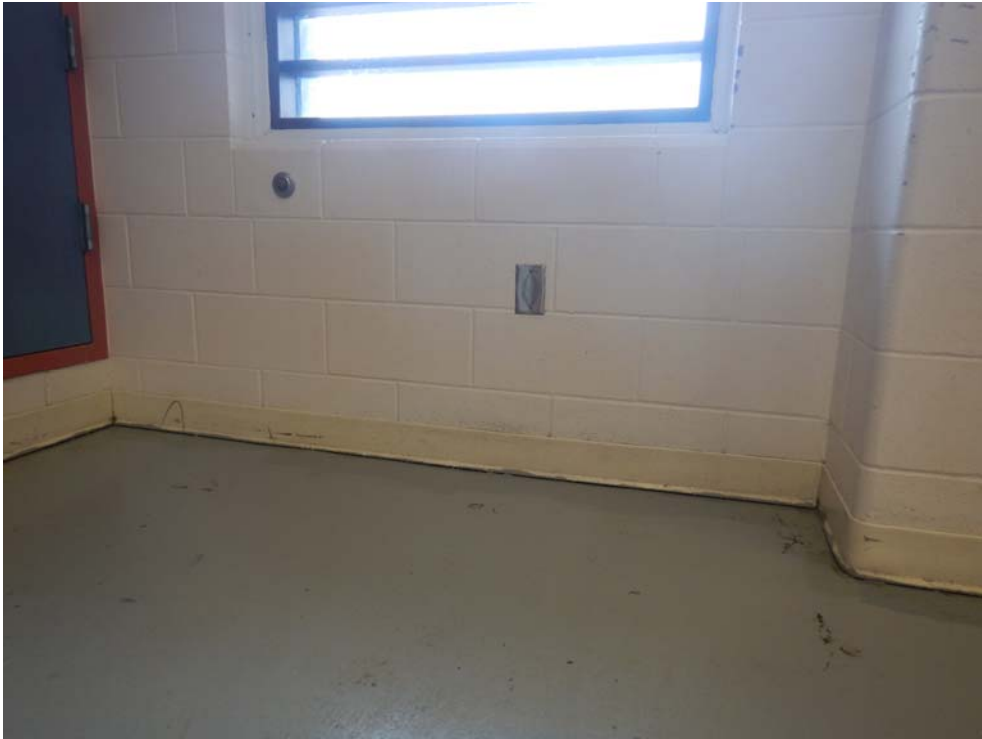
Photo # 5 Electrical box under existing window to be removed for new exit door. Range BD
