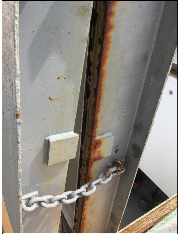
Figure 16: Condition of Side plates bottom edge
