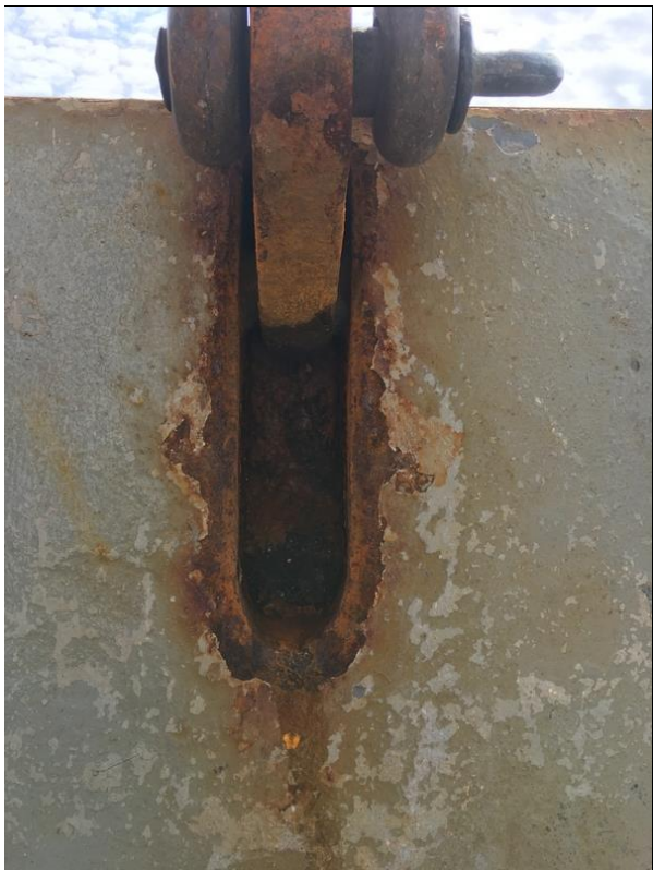
Figure 14: Condition of lifting lug, typ.
