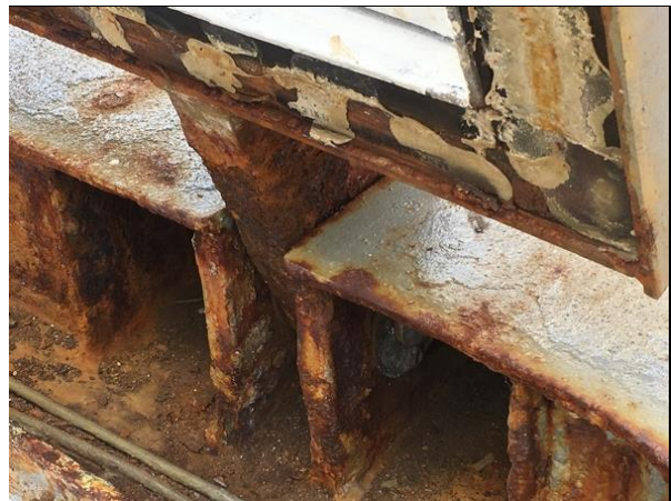
Figure 18: Condition of main hinges, typ.
