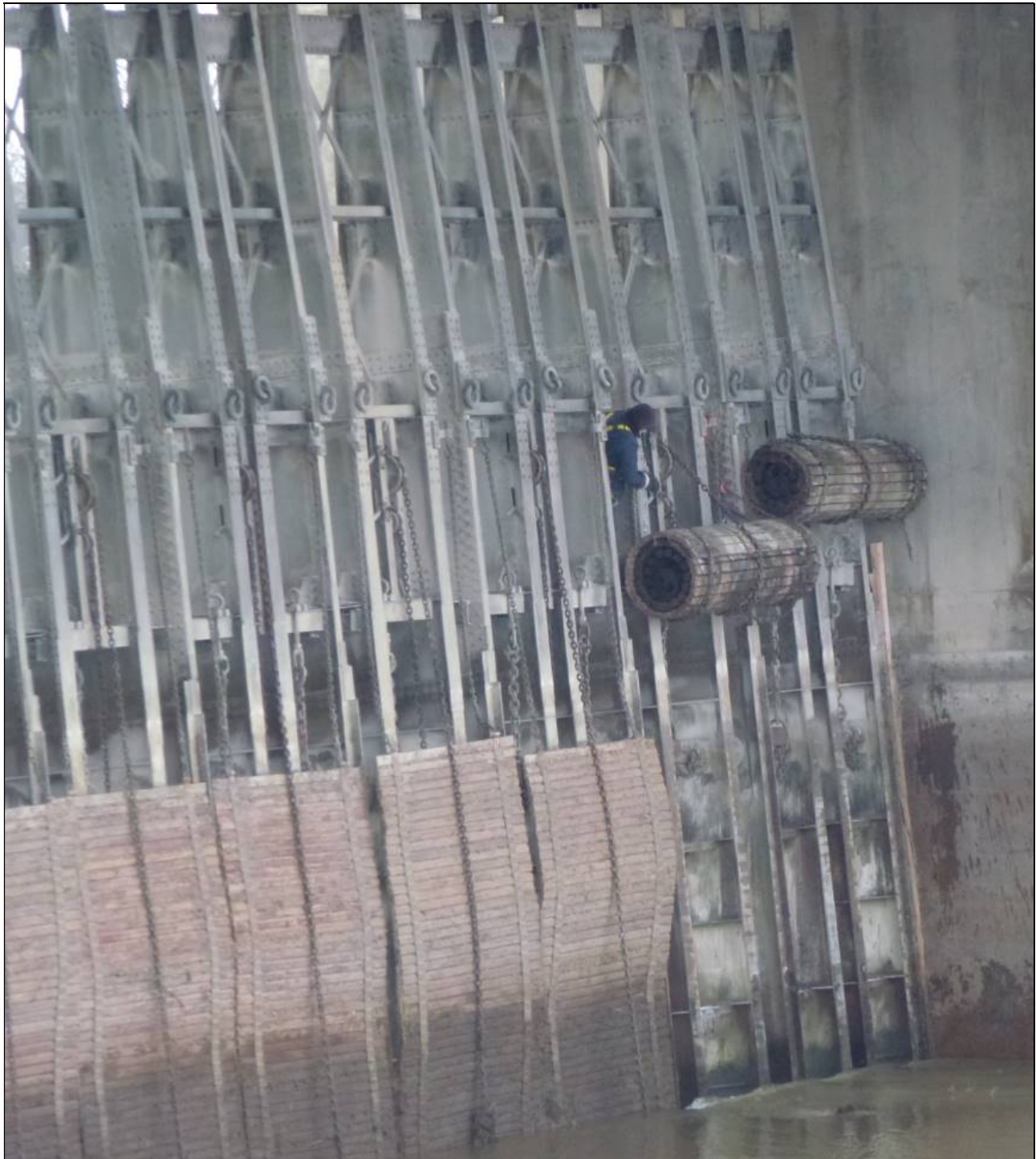
Figure 4: Upstream (south) side of frames. Curtains deployed at left, and being rolled-up at right The end of the curtain shoe is visible at the centre of each of the two rolled-up curtains
