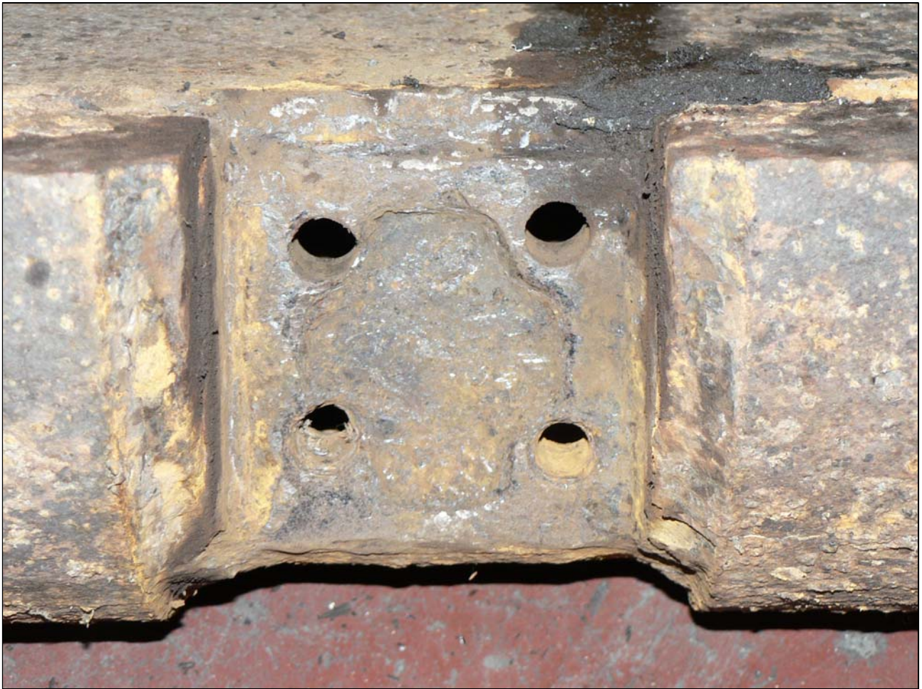
Figure 9: Existing curtain shoe, detail at centre showing holes for hinge connection
