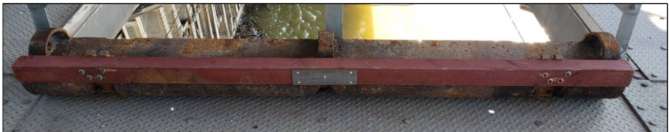
Figure 6: Existing curtain shoe connected to one wooden curtain slat
