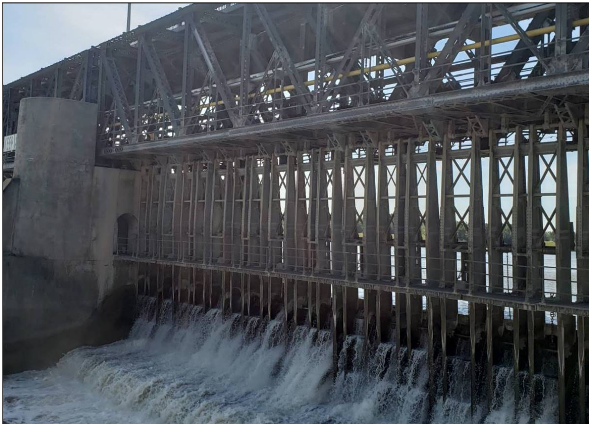
Figure 3: Downstream (north) side of dam with frames and curtains deployed
