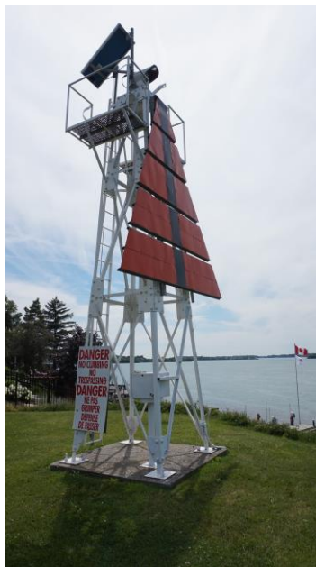
Figure 4: LL667 (front tower) Coordinates: 42° 6'51.00"N, 83° 6'42.90"W
