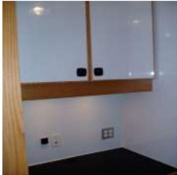
65. All exposed edges must have a 3mm, hardened PVC edge band applied to ensure durability and superior aesthetical qualities. Banding must be applied using AD-20, EVA Ethylene – Vinyl acetate based adhesive and using only machinery edge banding, may be color coordinated to match customer's countertop selection.
