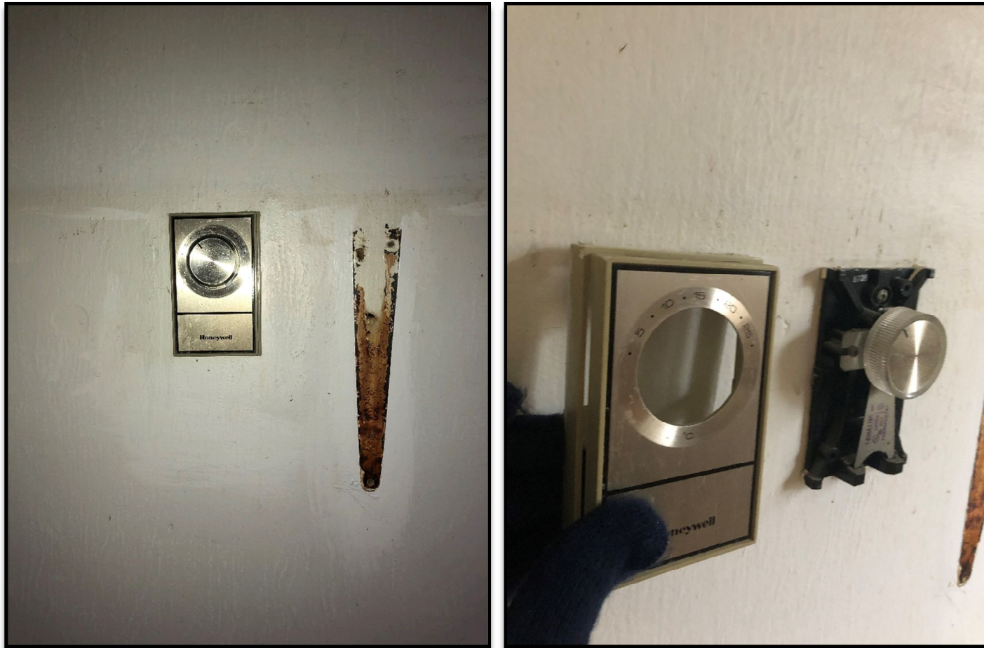
Thermostats within the Subject Site were inspected and did not contain mercury filled glass activator switch bulbs.
