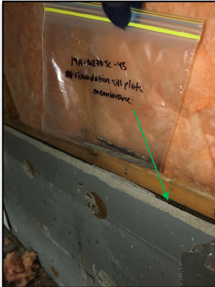
Sample 19A-6270-JC-43 membrane between sill plate and perimeter foundation in the warehouse was 'None Detected' for asbestos (left). Sample 19A-6270-JC-44 building paper between outer layer of OSB and exterior wood siding (coring) was 'None Detected' for asbestos (right).
