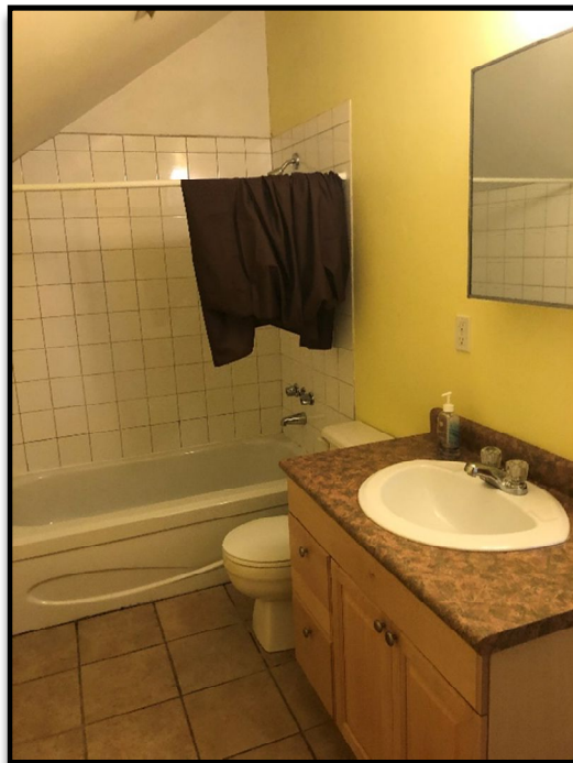
Upper residence bathroom showing 12" tan ceramic floor tile and 6" white ceramic wall tile (left). Sample 19A-6270-JC-41 of 12" tan ceramic floor tile with grout and mortar was 'None Detected' for asbestos (centre). Sample 19A-6270-JC-42 of 6" white ceramic wall tile with grout and mortar was 'None Detected' for asbestos (right).
