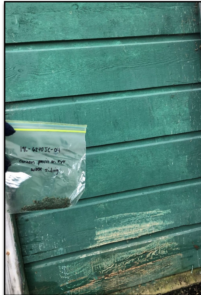
Green paint sample 19L-6270JC-04 applied to the exterior wood siding with lead concentration: 0.022\text{ wt\%} (220 ppm).
