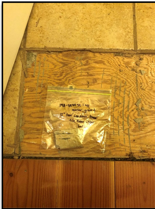
Upper residence bathroom showing 12" tan ceramic floor tile and 6" white ceramic wall tile (left). Sample 19A-6270-JC-41 of 12" tan ceramic floor tile with grout and mortar was 'None Detected' for asbestos (centre). Sample 19A-6270-JC-42 of 6" white ceramic wall tile with grout and mortar was 'None Detected' for asbestos (right).
