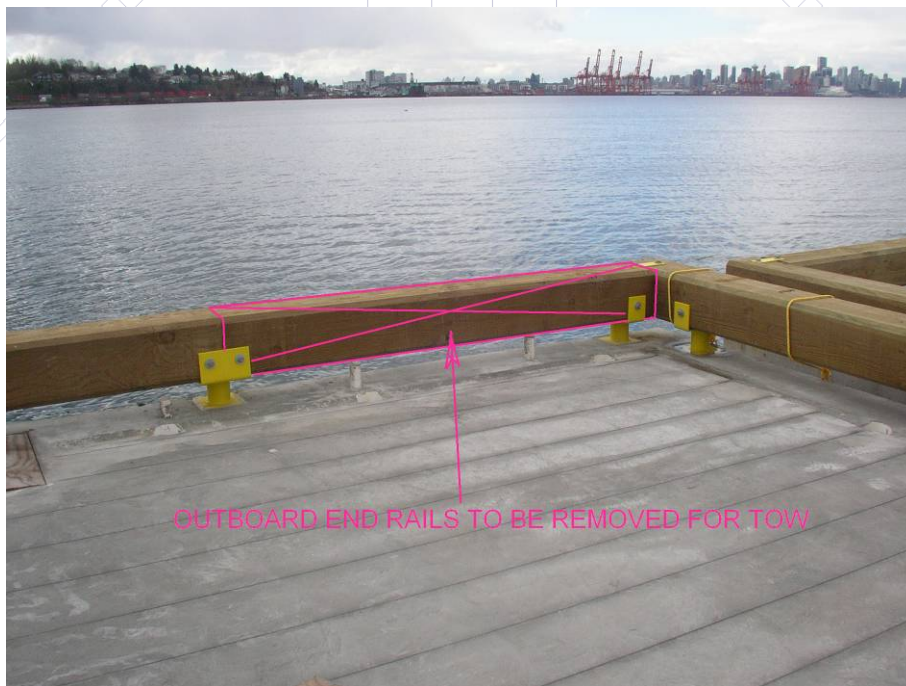
View showing 1 of 2 outboard bull rails to be removed for tow
