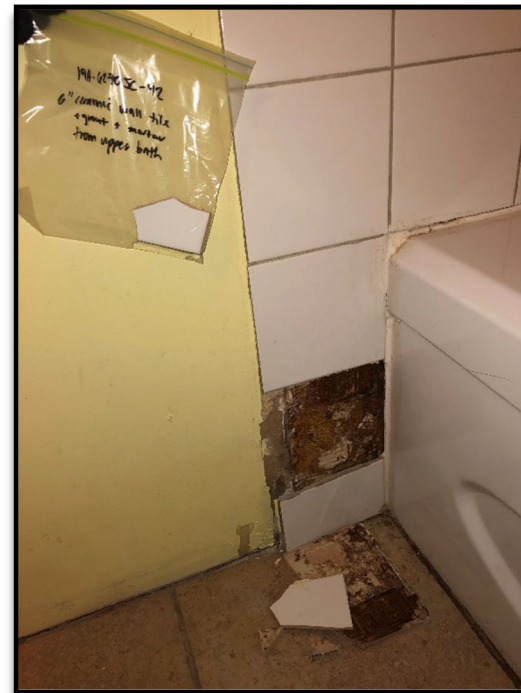
Upper residence bathroom showing 12" tan ceramic floor tile and 6" white ceramic wall tile (left). Sample 19A-6270-JC-41 of 12" tan ceramic floor tile with grout and mortar was 'None Detected' for asbestos (centre). Sample 19A-6270-JC-42 of 6" white ceramic wall tile with grout and mortar was 'None Detected' for asbestos (right).
