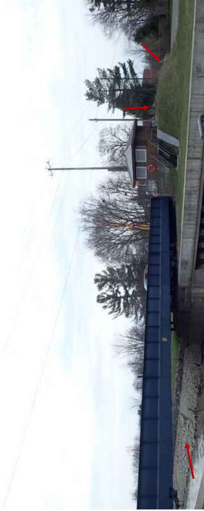
Figure 4. Warsaw Road Swing Bridge looking southeast (PCA 2019). Note that the area northwest of the swing bridge was built up while constructing the gatehouse. Also note the riprap treatment that covers the west bank south of the swing bridge to the bottom left of the picture.
