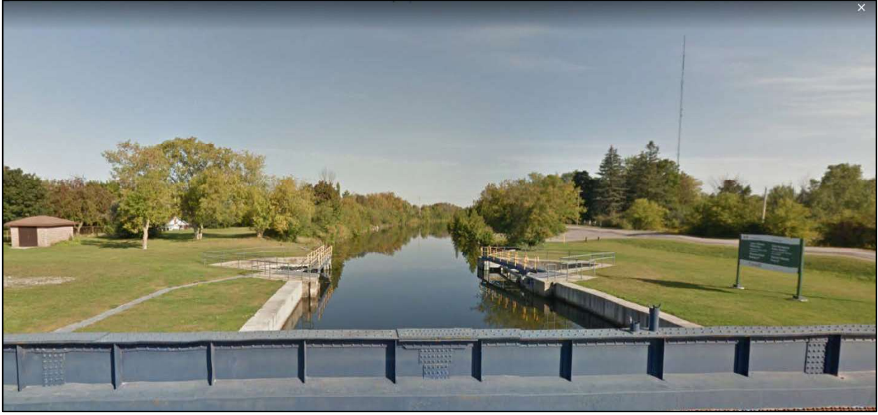
Figure 2: Google Street View of typical view upstream (north) of Warsaw Swing Bridge
