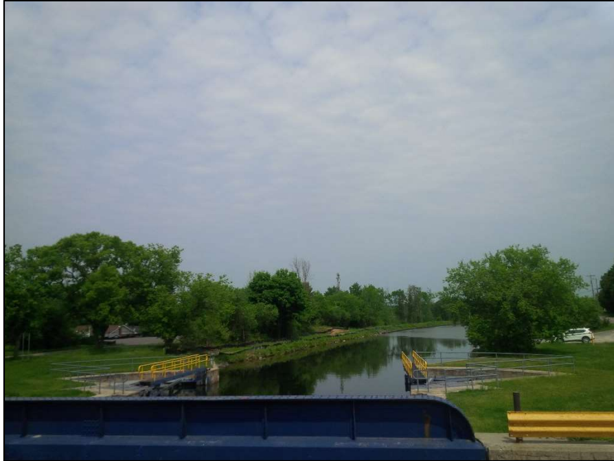
Photo 7: Typical landscape and vegetation of Warsaw Bridge area. Photo taken on the Warsaw Bridge, facing north (upstream). Photo taken by Environmental Officer, Sarah Bunting May 30th, 2018.
