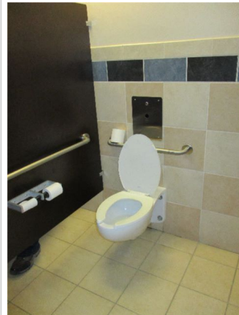
Plumbing Fixtures and Accessories - Washrooms - Typical fixture in office areas.
