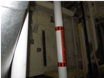
Humidifiers - Humidifier piping labelled
