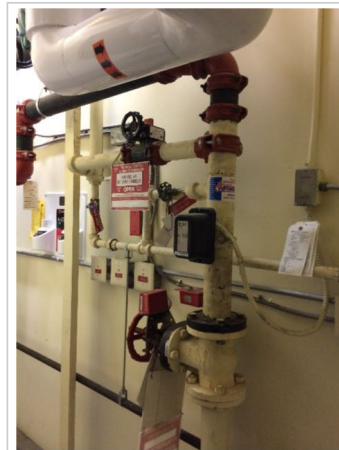
Wet Sprinkler System - Light Hazard w/Pump - Sprinkler with local zone valve
