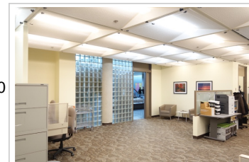
Glazed Block Partition - Typical interior glazed block wall
