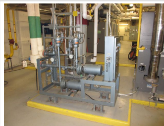
Plumbing Pumps - Domestic Water Booster System
