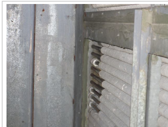
Test integrity and replace hydronic heating coils in air handling units - Fins removed from coil tube failure
