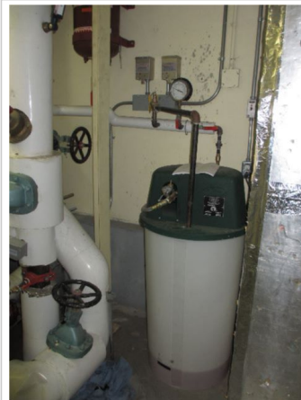
Penthouse Hydronics - Glycol feed system - typical
