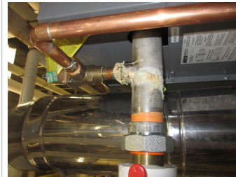
03.1A-050 Boilers - Corrosion on piping at DHW boiler
