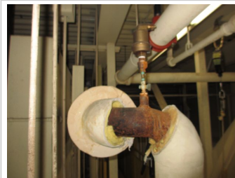
Heating & Cooling Piping Systems - Insulation removed for maintenance, not replaced
