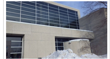
Curtain Wall System - Curtain wall above the main entrance on the south elevation.
