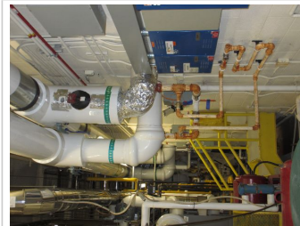
Repair piping insulation - chilled water piping. - Poorly insulated chilled water piping in boiler room at exterior wall
