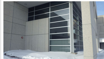
Curtain Wall System - Curtain wall on the east elevation.
