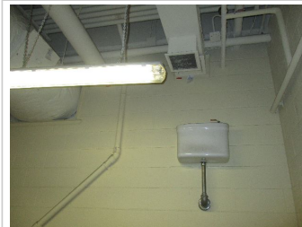
Plumbing Fixtures and Accessories - Washrooms - Abandoned flush tanks in janitor rooms
