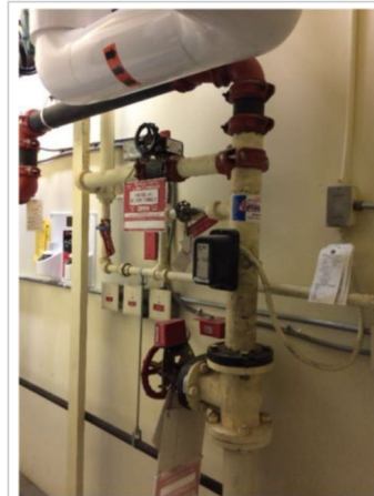
Revision to existing glycol sprinkler system per NFPA 25 - Glycol filled automatic sprinkler
