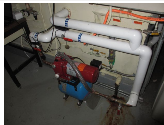
Plumbing Pumps - Penthouse DCW booster pump
