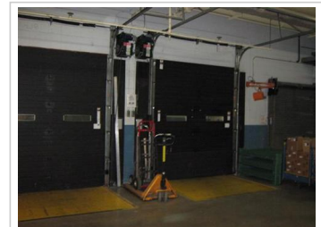
Oct.26-28 080 (Small).jpg - Two dock levelers in the shipping/receiving area.
