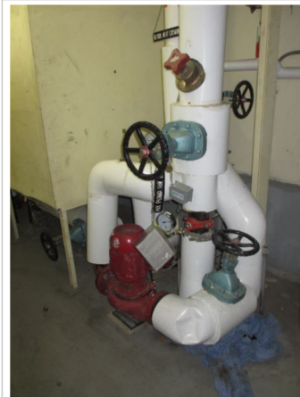
Penthouse Hydronics - Hydronic system arrangement in penthouse
