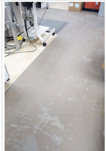
Sealed-Epoxy Concrete Floor - Mail Processing - Worn out sealed concrete flooring in mail processing area
