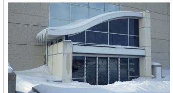
Ext.W-Synthetic plaster on rigid insulation - Synthetic plaster exterior finish
