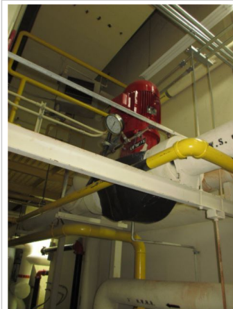
Penthouse Hydronics - Typical circulator pump.
