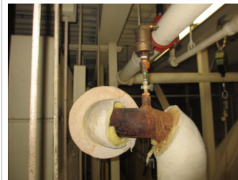
Repair piping insulation - chilled water piping. - Uninsulated chilled water piping
