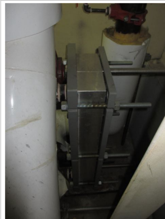
Penthouse Hydronics - Glycol heat exchanger
