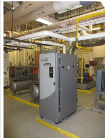
03.1A-050 Boilers - Heating system condensing boiler
