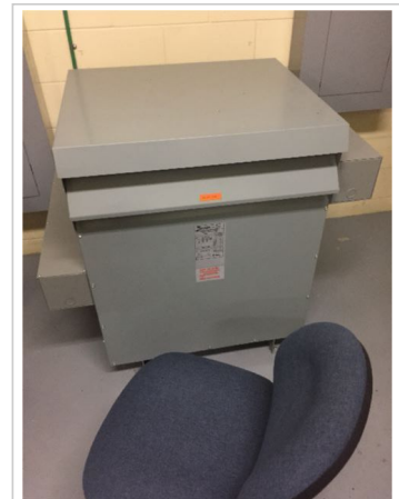
Secondary Transformer - 600V-120/208V Transformer
