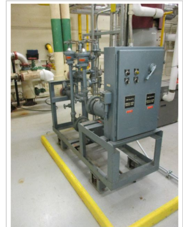
Plumbing Pumps - Domestic Water Booster Pumps
