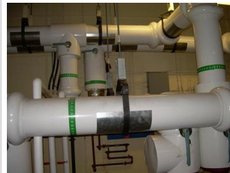
mech 025 (Small).jpg - Chilled water piping located in boiler room.
