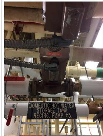
Replace 4 hot water circulator pumps - DHW pump 3
