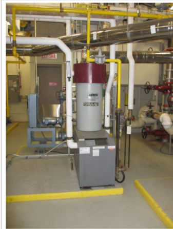
03.1A-050 Boilers - DHW boiler
