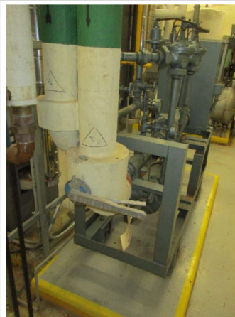
Plumbing Pumps - Domestic DCW Booster Pumps- Basement mech rm
