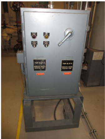
Plumbing Pumps - DCW booster control system
