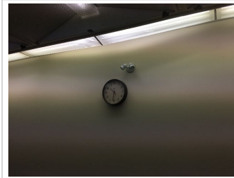
Emergency Lighting - Emergency Light Remote Head
