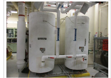
Water Storage Tanks - DHW - Domestic water storage tanks
