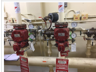
Fire Alarm System - Tamper and Flow Valves
