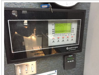
Fire Alarm System - Remote Annunciator Panel
