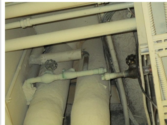
Water Dist Complete - Average - exposed piping, disconnected branch
