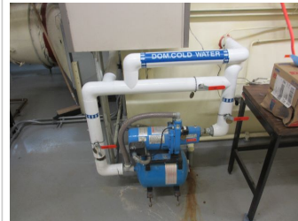
Water Dist Complete - Average - domestic water in penthouse is boosted
