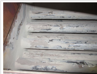
Humidifiers - HU-2 Steam tube calcification - open for maintenance
