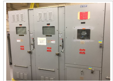
Primary Switch Gear - Primary Switchgear
