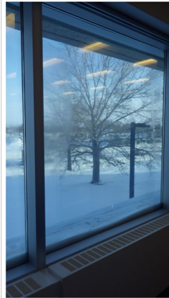
Aluminum Windows - Condensation build-up with-in the sealed glazing unit.
