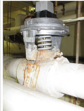
Renew pneumatic control valves - long term renewal - Leaking control valves.
