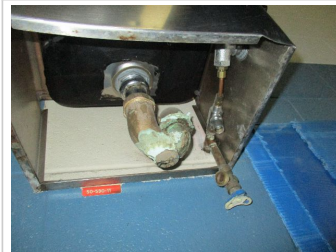
Water Coolers - Wall-Mounted - Disconnected - loading dock
