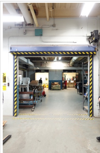
Painted Concrete Floor - Worn painted concrete floors in heavy traffic corridors.
