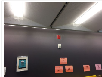
Fire Alarm System - Horn and Strobe Signalling Devices
