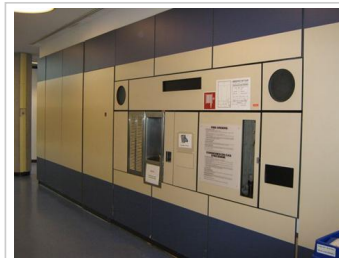
Oct.26-28 063 (Small).jpg - Plastic laminated wall panels enclose the washroom and service areas.
