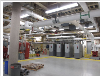
03.1A-050 Boilers - Heating system condensing boilers
