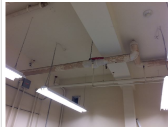
Water Dist Complete - Average - piping with discoloured insulation
