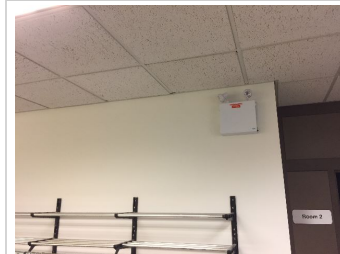
Emergency Lighting - Emergency Battery Unit
