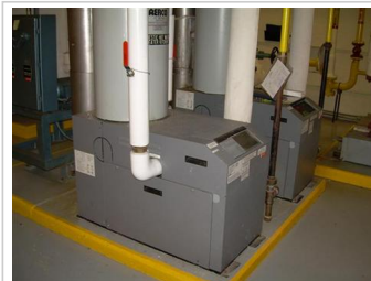
mech 004 (Small).jpg - Two Aerco domestic hot water boilers, located in the boiler room.
