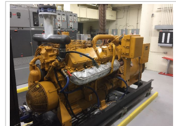
Emergency Power System - Diesel Generator
