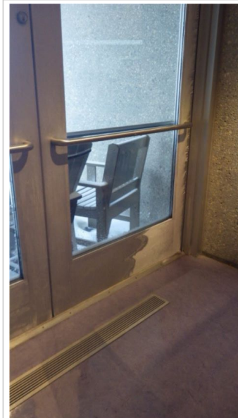
Glazed Doors - Frost build-up on one of the glazed aluminum doors in the lunchroom.
