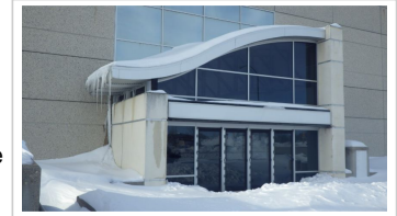
Metal Roofing - High End - New - Standing seam metal roof on the east facing exit/entrance vestibule.
