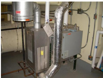
mech 055 (Small).jpg - A Dri-Steem humidifier, which services an AHU, and is located in one of the penthouses.
