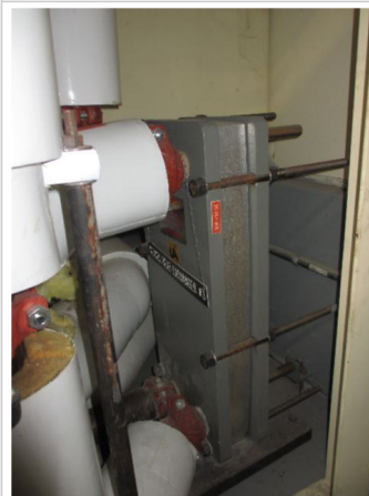
Penthouse Hydronics - Glycol heat exchanger
