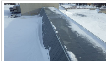
Modified Bitumen - Modified bitumen roofing membrane at the clearstory.
