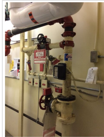
Testing of automatic sprinkler systems with glycol - Typical glycol filled automatic sprinkler
