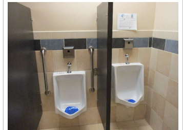
Plumbing Fixtures and Accessories - Washrooms - Urinal with auto-flush - representative of average unit
