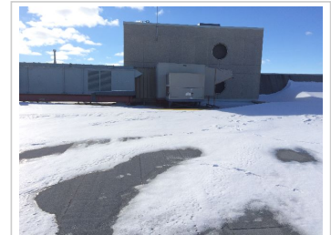
Roof Top Units - RTU - heating and cooling - RTUs shown together (Eng Air and Racan w/McQuay chiller)
