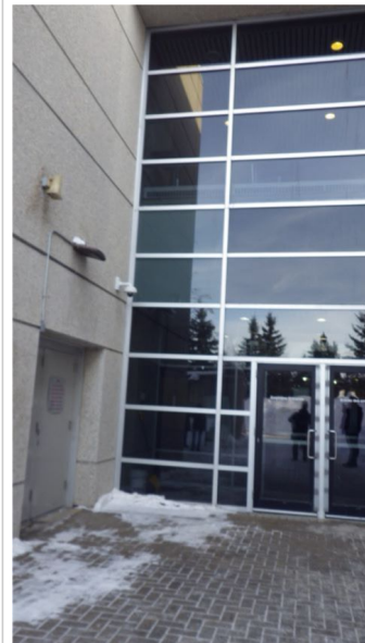
Curtain Wall System - Curtain wall on the west elevation.
