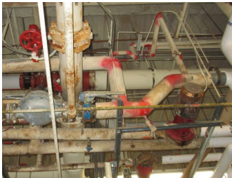
Replace 2 DHW pumps - Domestic water pump (RHS)
