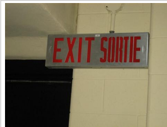
IMG_0051 (Small).JPG - Typical bilingual exit light fixture.
