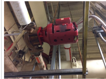
Replace 4 hot water circulator pumps - DHW pump
