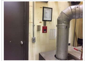
Fire Alarm System - Manual Pull Station
