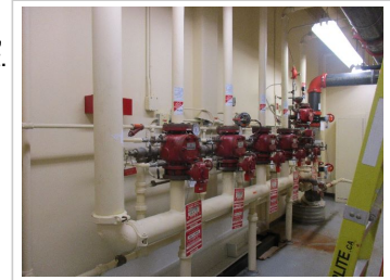
Wet Sprinkler System - Light Hazard w/Pump - Sprinkler tree
