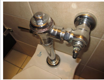
Plumbing Fixtures and Accessories - Washrooms - Manual flush valve, corroded
