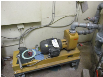
Plumbing Pumps - Pond Aerator Pump
