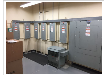
Distribution System - Heavy Capacity - Distribution Panels
