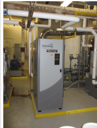
03.1A-050 Boilers - Heating system condensing boiler
