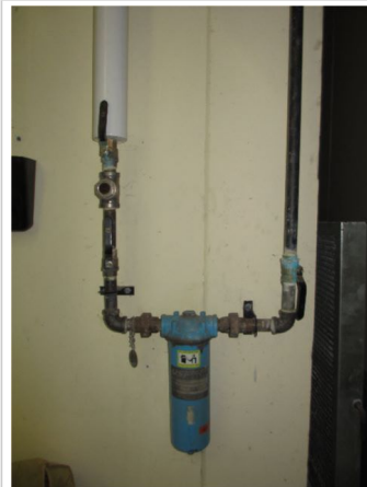
Penthouse Hydronics - Hydronic system treatment
