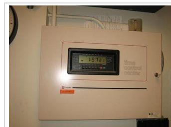
IMG_0066 (Small).JPG - Main control panel for clock system.
