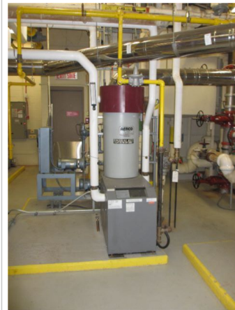
Replace 1 domestic hot water boilers - Existing domestic hot water boiler
