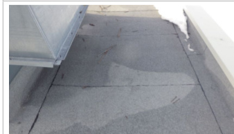
Modified Bitumen - Modified bitumen roofing membrane on one of the mechanical penthouses.
