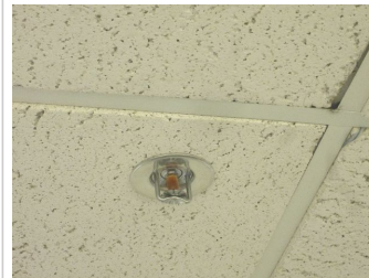
Wet Sprinkler System - Light Hazard w/Pump - Typical sprinkler head in office area
