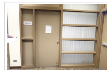
Steel Windows - Typical Interior sidelite glazing
