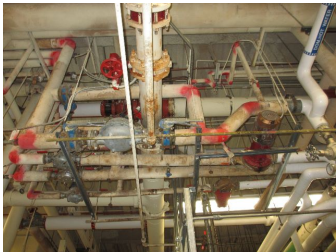
Plumbing Pumps - DHW Recirculator pumps
