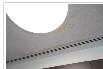
Gypsum Board Ceiling - Water staining around light and ceiling grille
