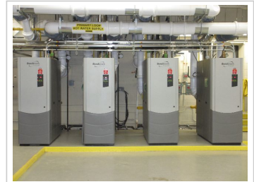
03.1A-050 Boilers - Heating system condensing boilers
