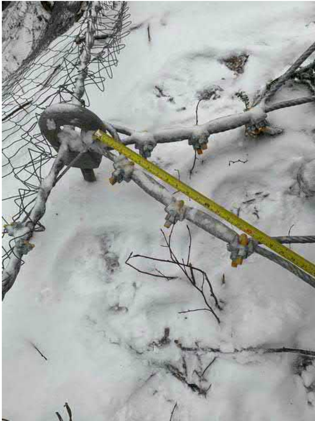
Photograph 1: View of Intermediate Main Anchor and supporting Auxiliary Cables.
