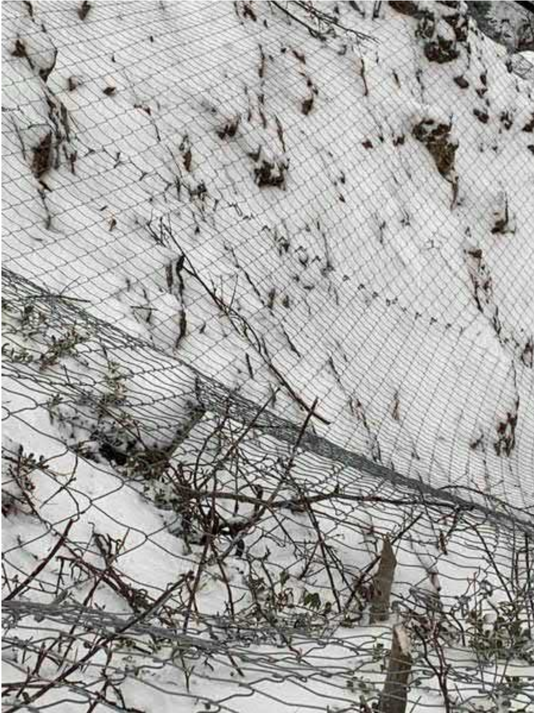
Photograph 4: View looking down mesh showing mesh connection clip arrangement.
