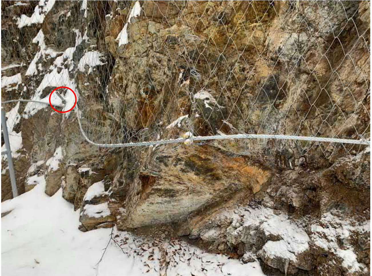
Photograph 7: View looking along base of mesh where it is above the top of the valve house. Red circle indicates a rock anchor used to pin the mesh to the slope.
