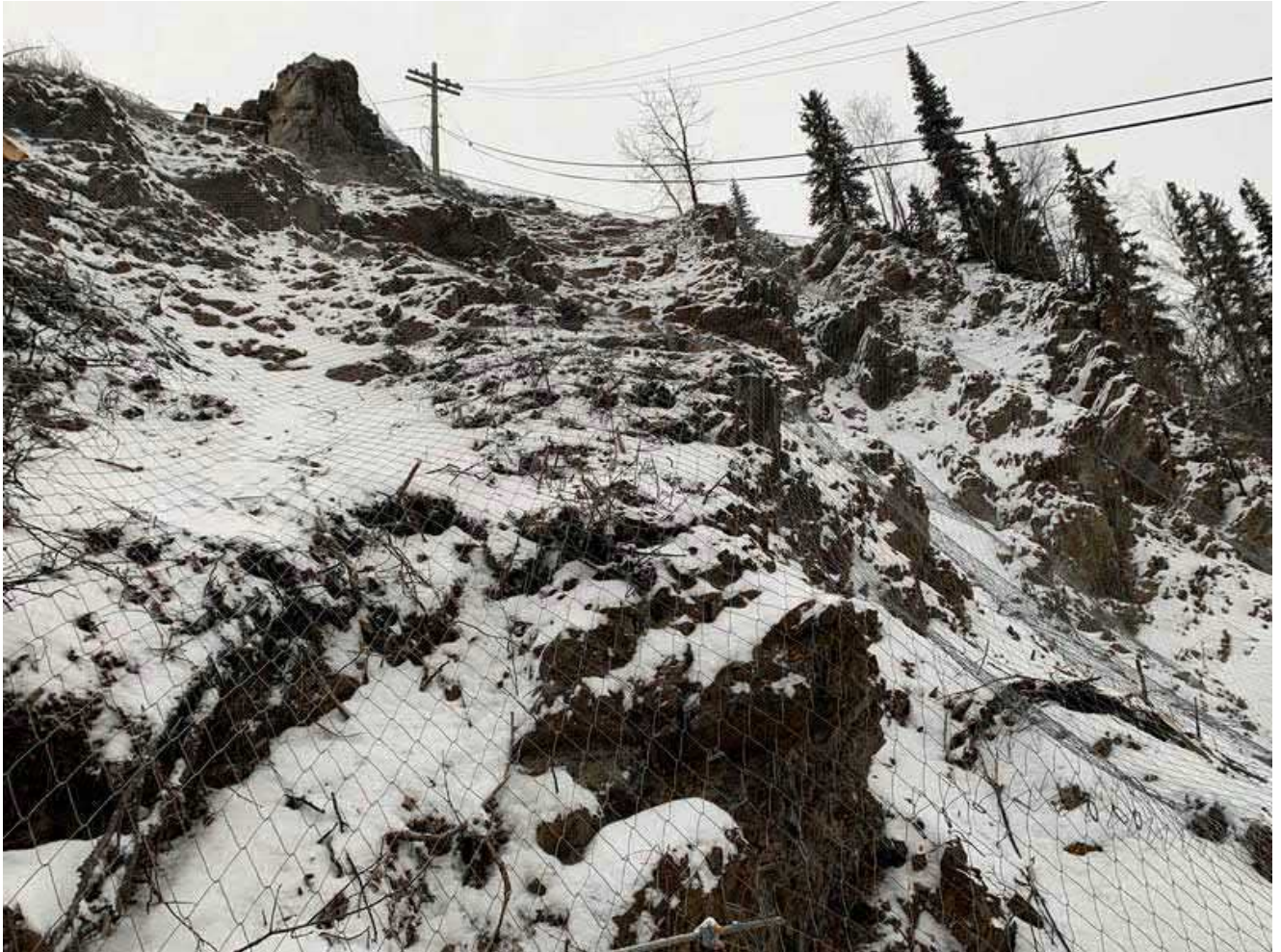
Photograph 6: View looking up slope showing mesh area.
