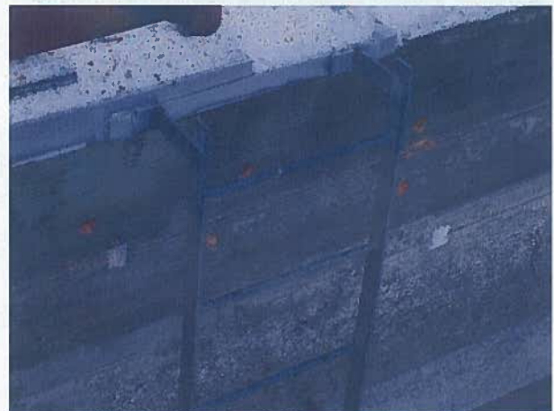
Photo 6: View of upper timber sampling locations on the downstream gate.
