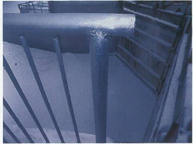
Photo 8: View of railing located on concrete structure past the downstream gate. Gate appeared to be finished with a galvanized or very thin powder coat finish. No sample collected.
