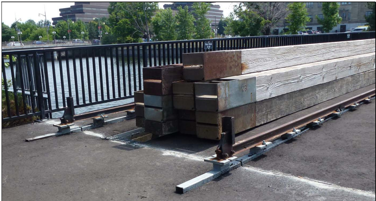
Figure 7: Stoplog storage on the operational deck is immediately downstream of the sluice.
