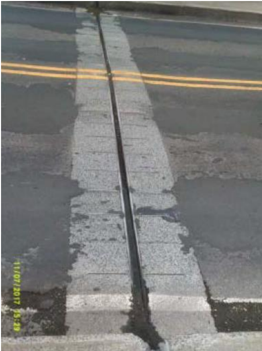
Photography 13: Concrete expansion joint.
