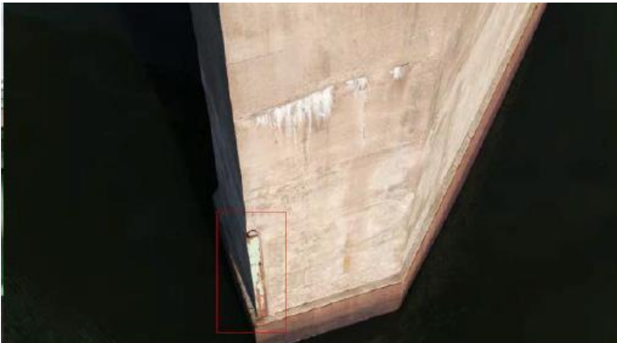
Photograph 4: Ice shield on pier 7.
