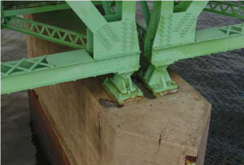
Photograph 1: Pier – bearing grout.
