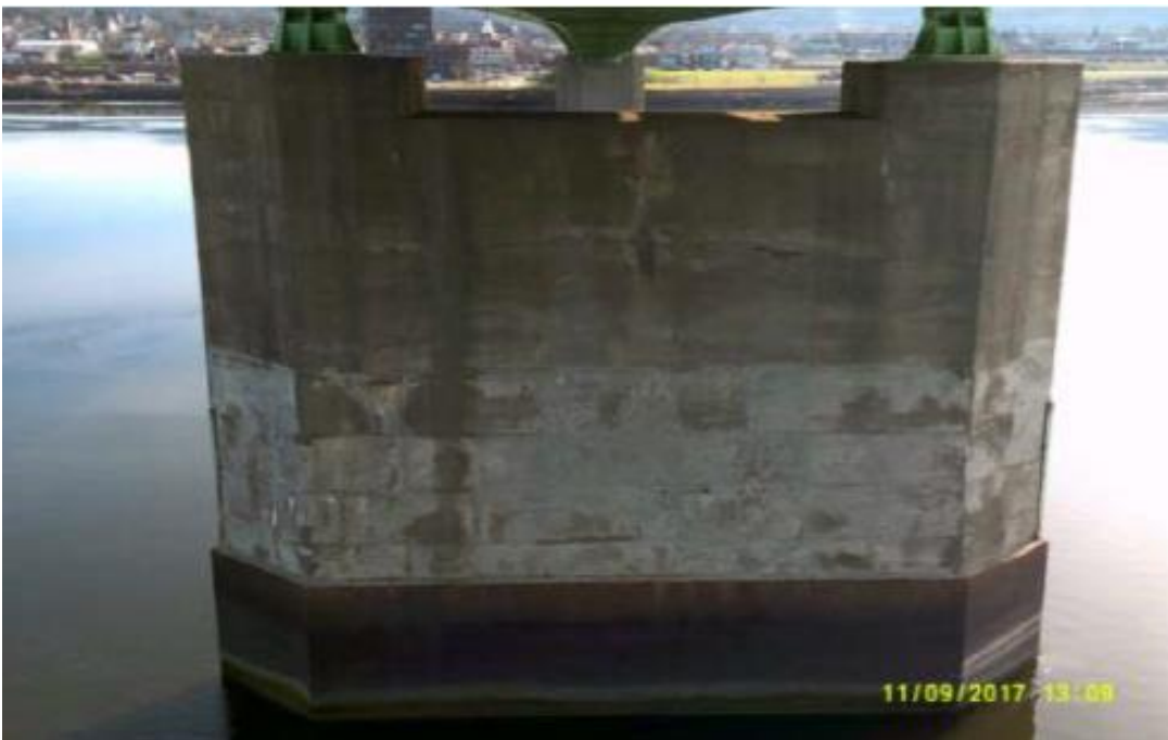
Photograph 2: Pier – example of concrete surface repairs.
