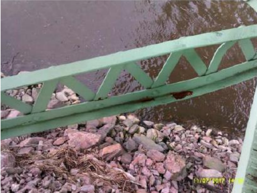
Photography 12: Lateral brace rail to be replaced.
