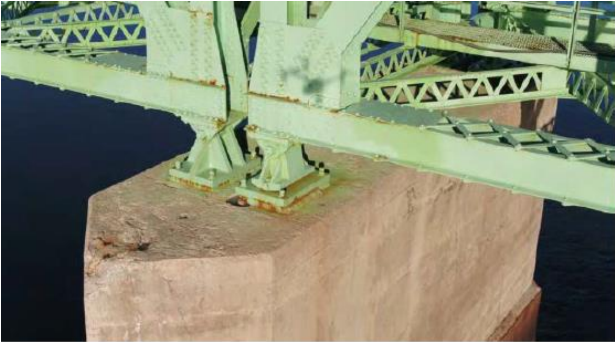
Photograph 3: Pier – example of concrete surface repairs.
