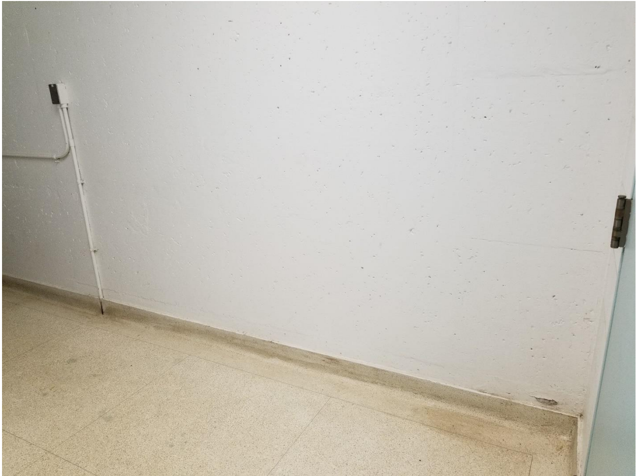
Photo 3: White paint applied to walls in the south-east stairwell, contains 557 ppm lead (DST Sample LP-03).
