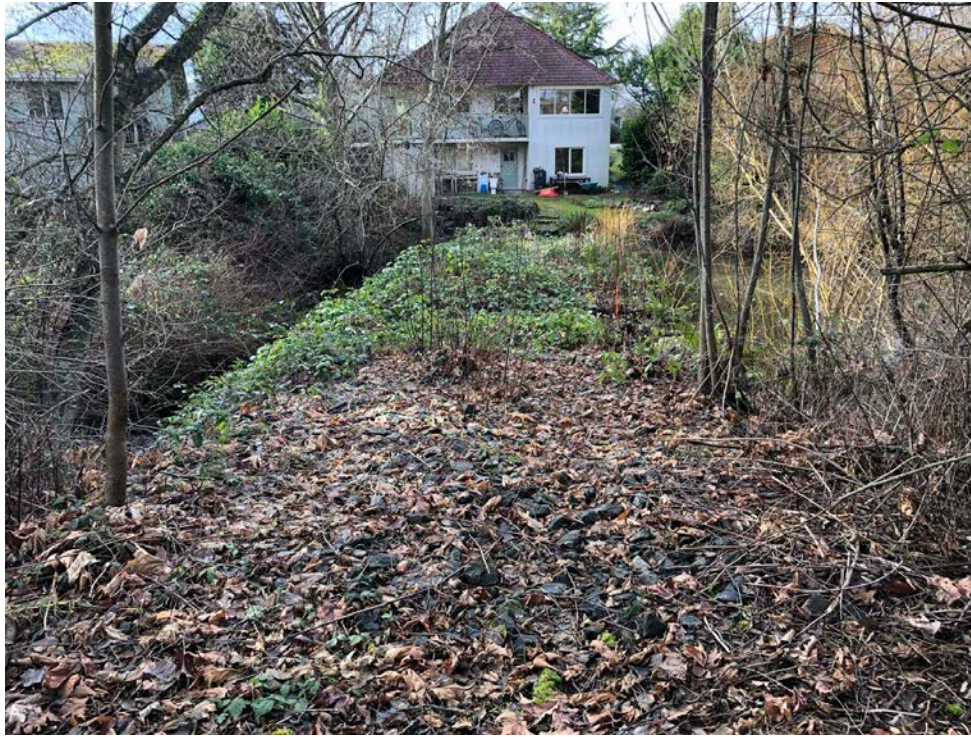
Photo 1: KÉL,SET (Reay) Creek Pond Dam, looking southwest.
