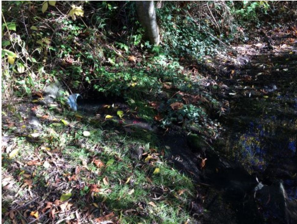
Photo 33: One of several storm outlets along north side of KÉL,SET (Reay) Creek Pond on Town of Sidney property, looking east.
