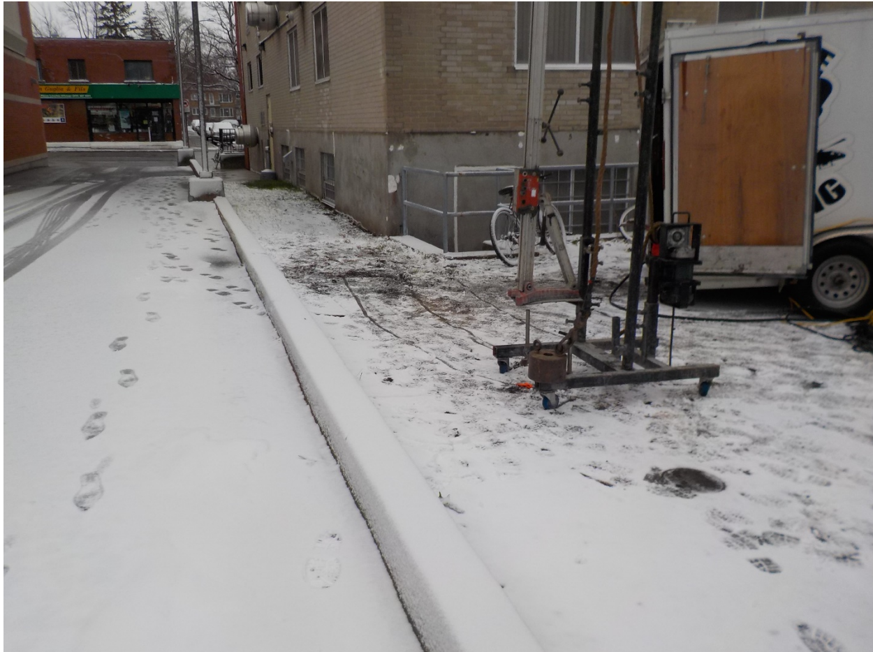
Photograph 1: View of the site at borehole 19F01 location – November 28 th , 2019
