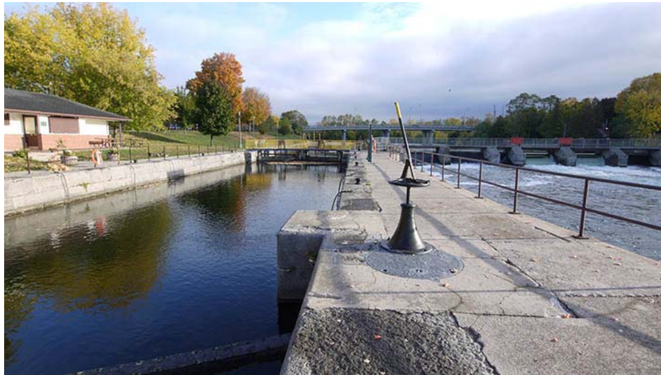
Figure 12: The mass, scale of the lock and the colour and the finish of the concrete are valued characteristics. [HCS, 2016]
