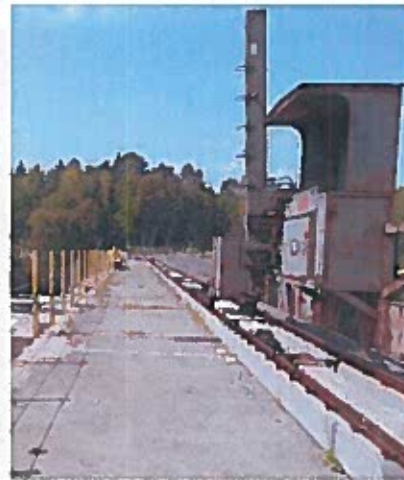
Figure 14. Otonabee Dam with a hydraulic log lifter mounted on rails to right (PCA 2015d).
