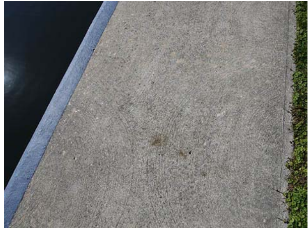
Figure 54: The broom finish of the concrete work at Talbot is a valued characteristic. [HCS 2016]
