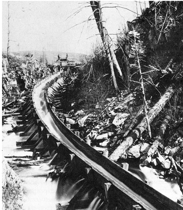
Figure 71: Example of one of the means of moving lumber within the waterway – a single timber slide. [Angus, 1998]
