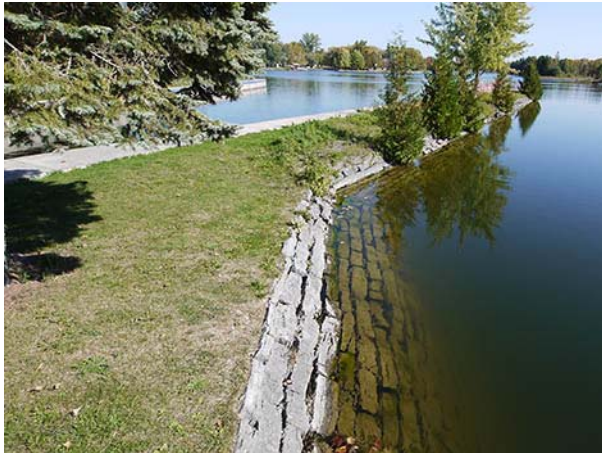
Figure 53: The neat rows of stone along the water's edge are a valued built element in addition to the concrete canal and dam and shared with other sites such as at Otonabee. [HCS 2016]
