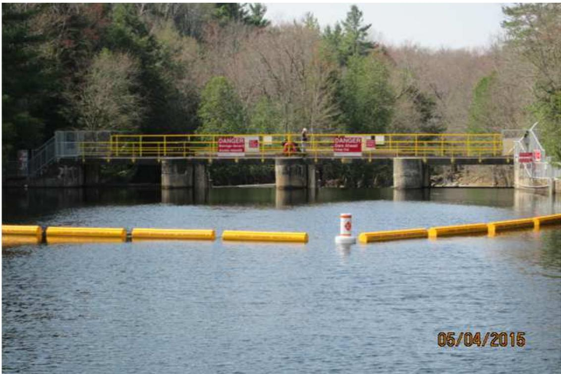
FLOAT COLLAR CAN BUOY C/W INTERNAL CONCRETE BALLAST. SEE SPECS
