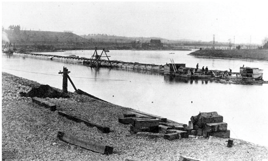
Figure 75: Myers Island protection wall under construction 1913. [Angus, 2000]
