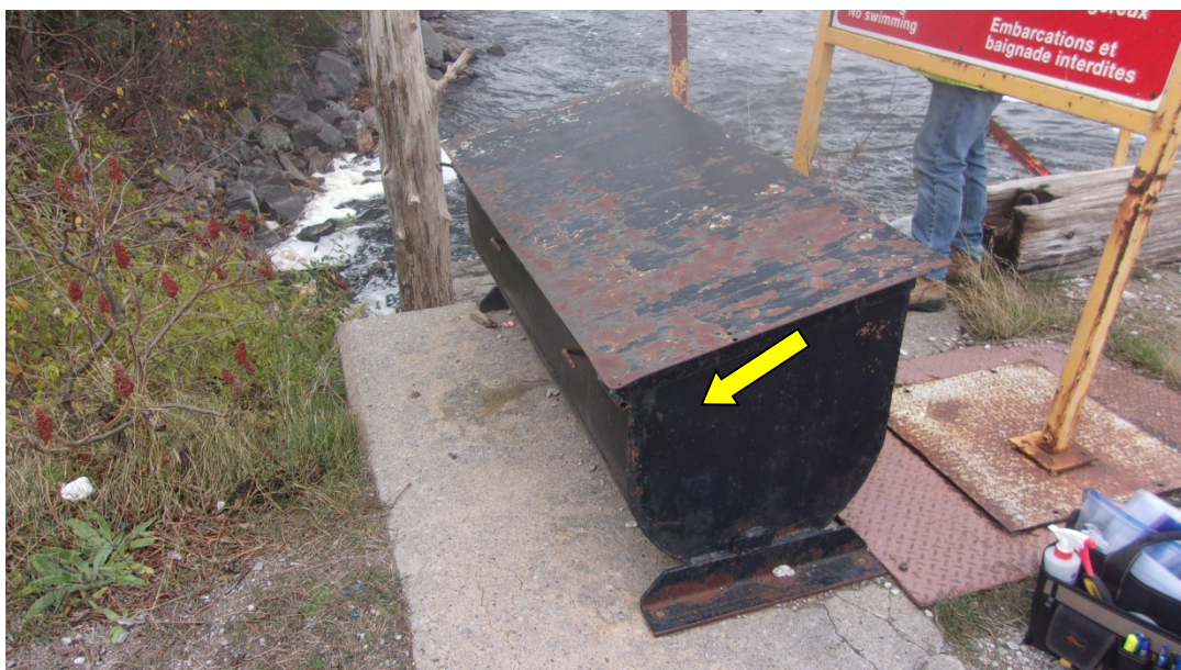
Photograph 4: Lead containing black paint on storage box
