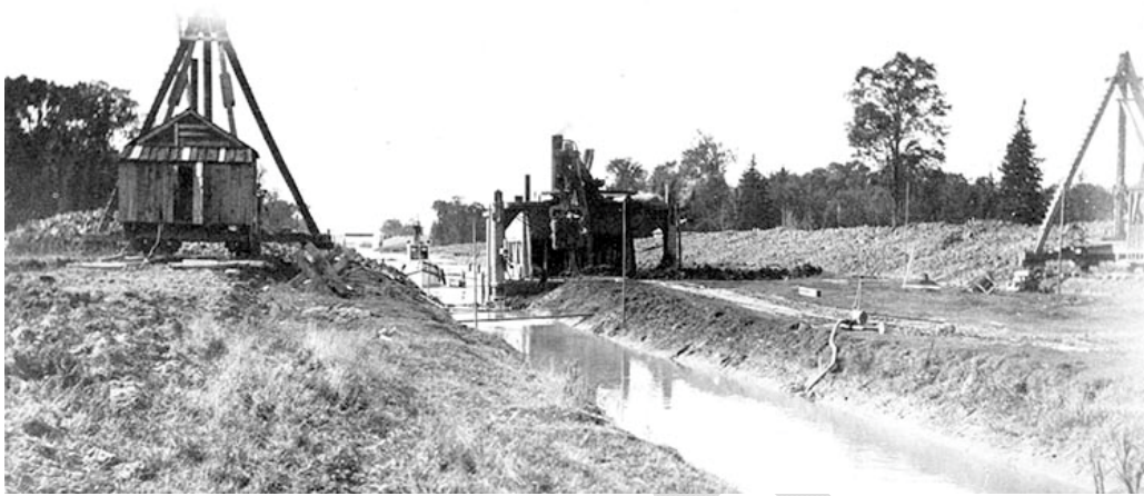
Figure 48: Dredge excavating the canal prism between Gamebridge and Lake Simcoe. Date Unknown [Angus, 2000]
