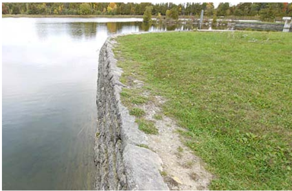
Figure 40: The stone retaining wall detail at Otonabee lock no. 23 is also present at other sites, including Talbot lock no. 38. [HCS 2016]
