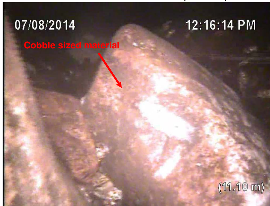
PHOTO 4.1-5 CONDITION OF VOID AT PIER #1 (CH14-103)
