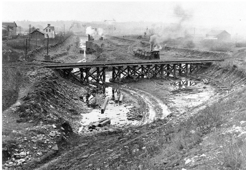
Figure 72: Temporary Rail bridge constructed at Trenton 1908. [Angus, 2000]
