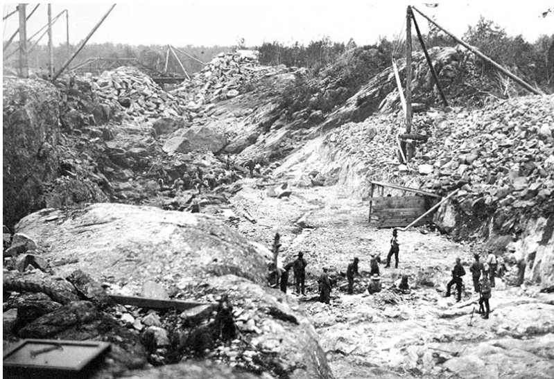
Figure 16: Excavating canal prism at Burleigh Falls through hard granite 1885. Note the bridge crossing in top left hand corner. [Angus, 2000]
