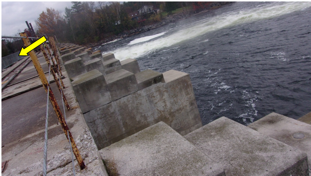
Photograph 3: Lead containing yellow paint on guardrails
