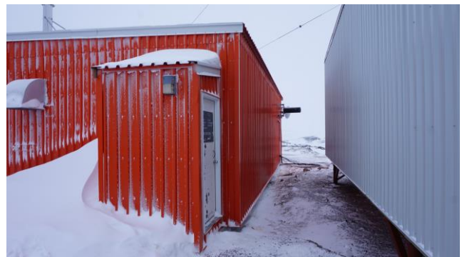
Figure 7: Building viewed from South
