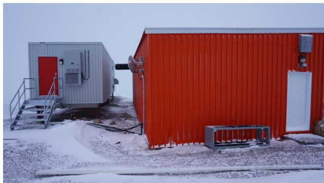
Figure 6: Building viewed from East
