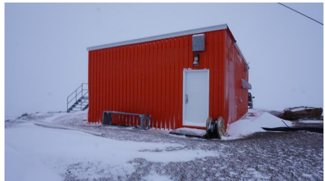
Figure 5: Building viewed from North
